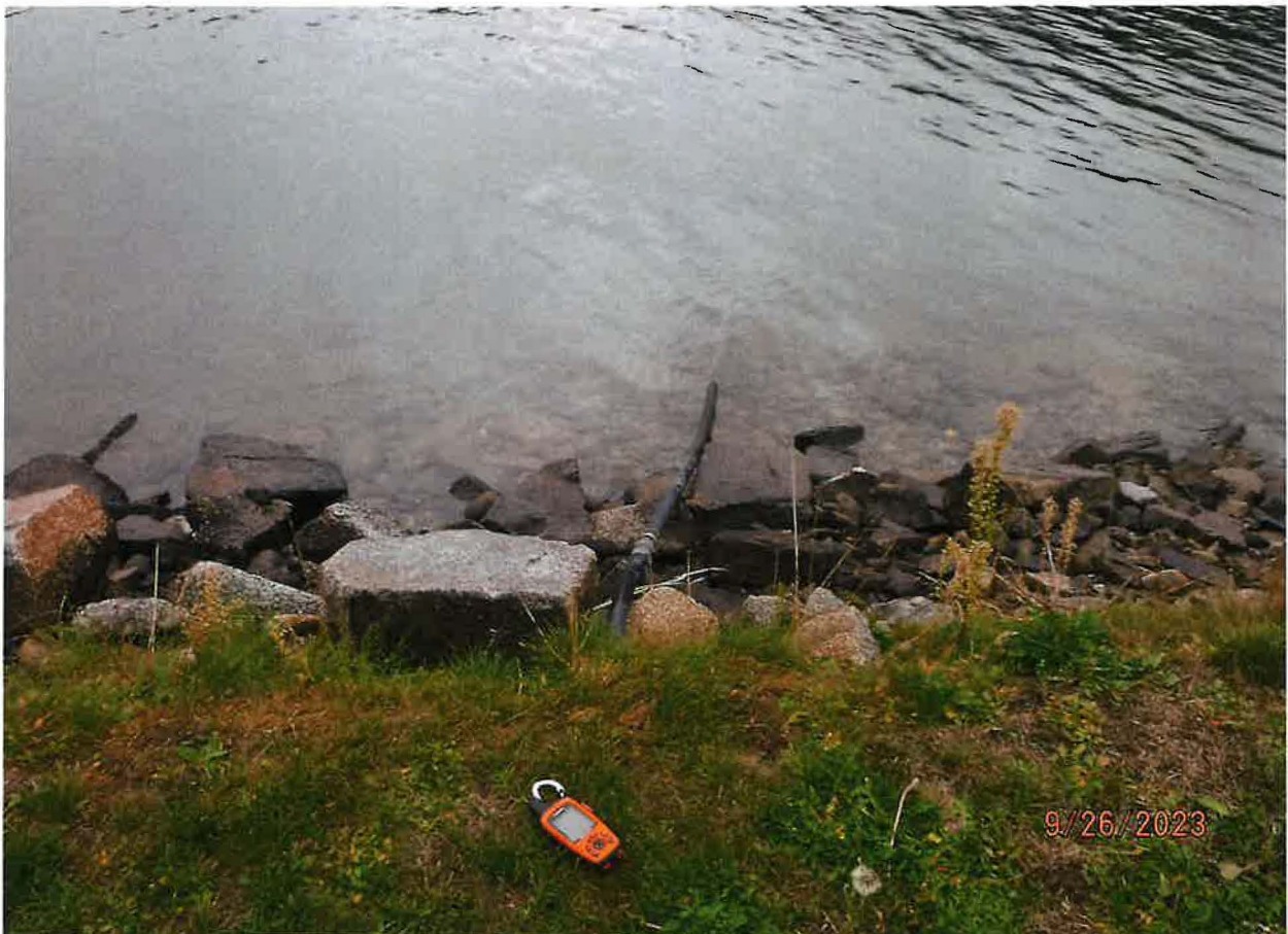
POD – INTAKE PIPE WITH SCREENED FOOT VALVE IN RIVER
