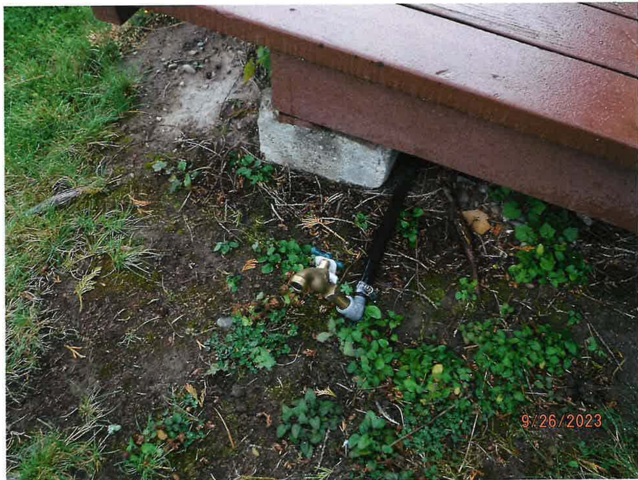
FROM PUMP BURIED POLY LINE ROUTES TO 2EA IRRIGATION HOSE BIB RISERS
