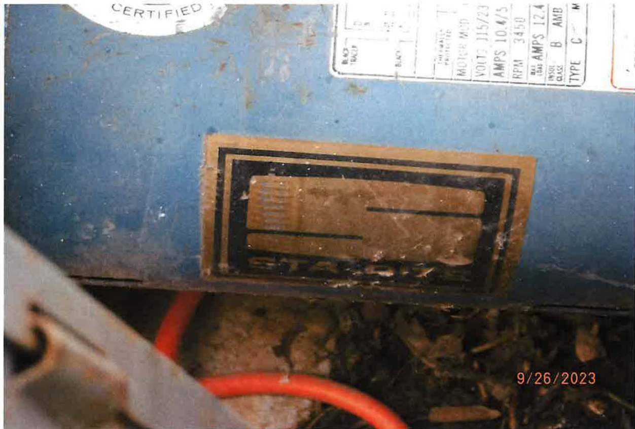
STA-RITE 3/4 HP PUMP MOTOR P/N C48J2EC11
