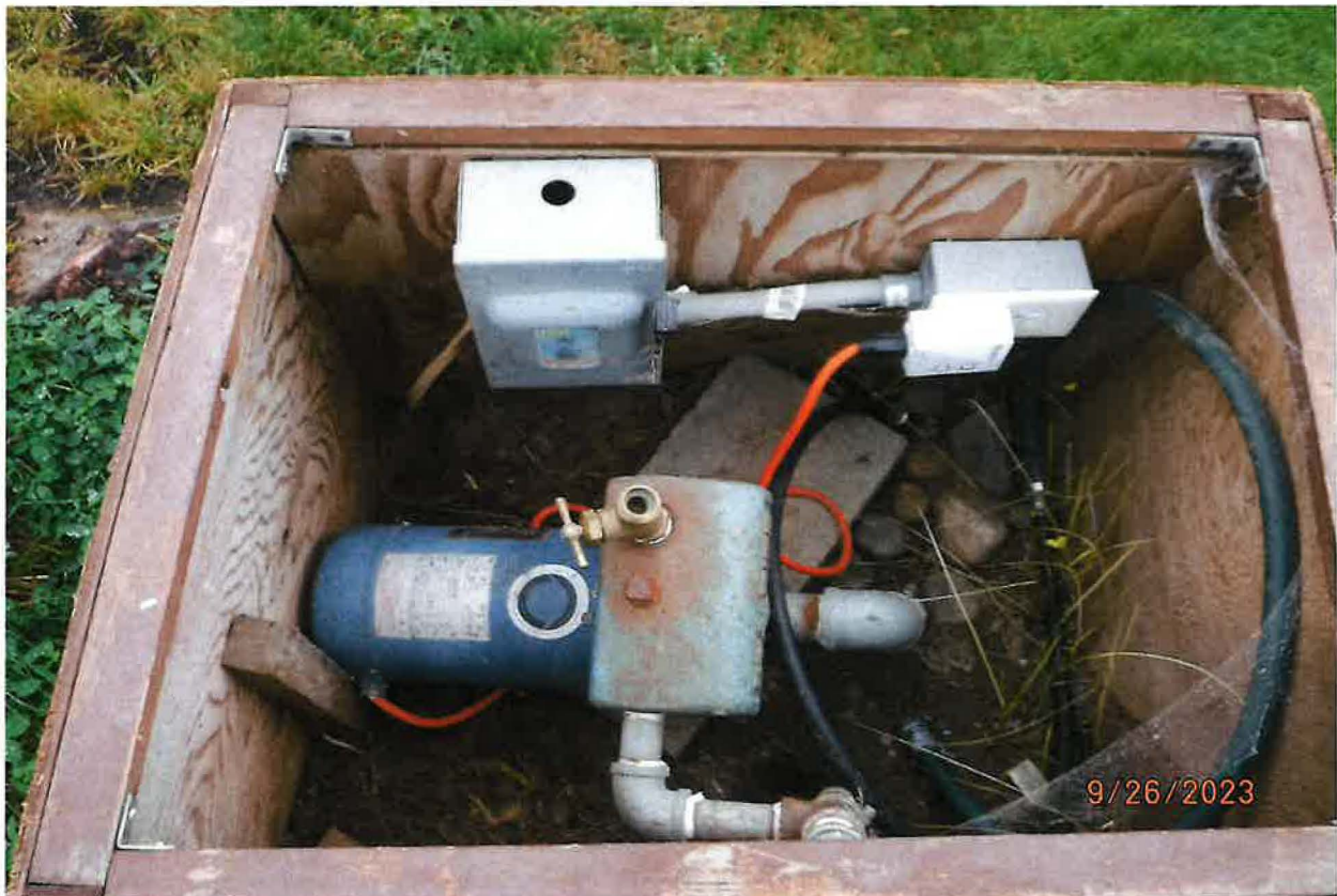
DIVERTING WORKS INCLUDE \frac{3}{4} HP WATER TRANSFER PUMP TO TWO SEPARATE HOSE BIBS
