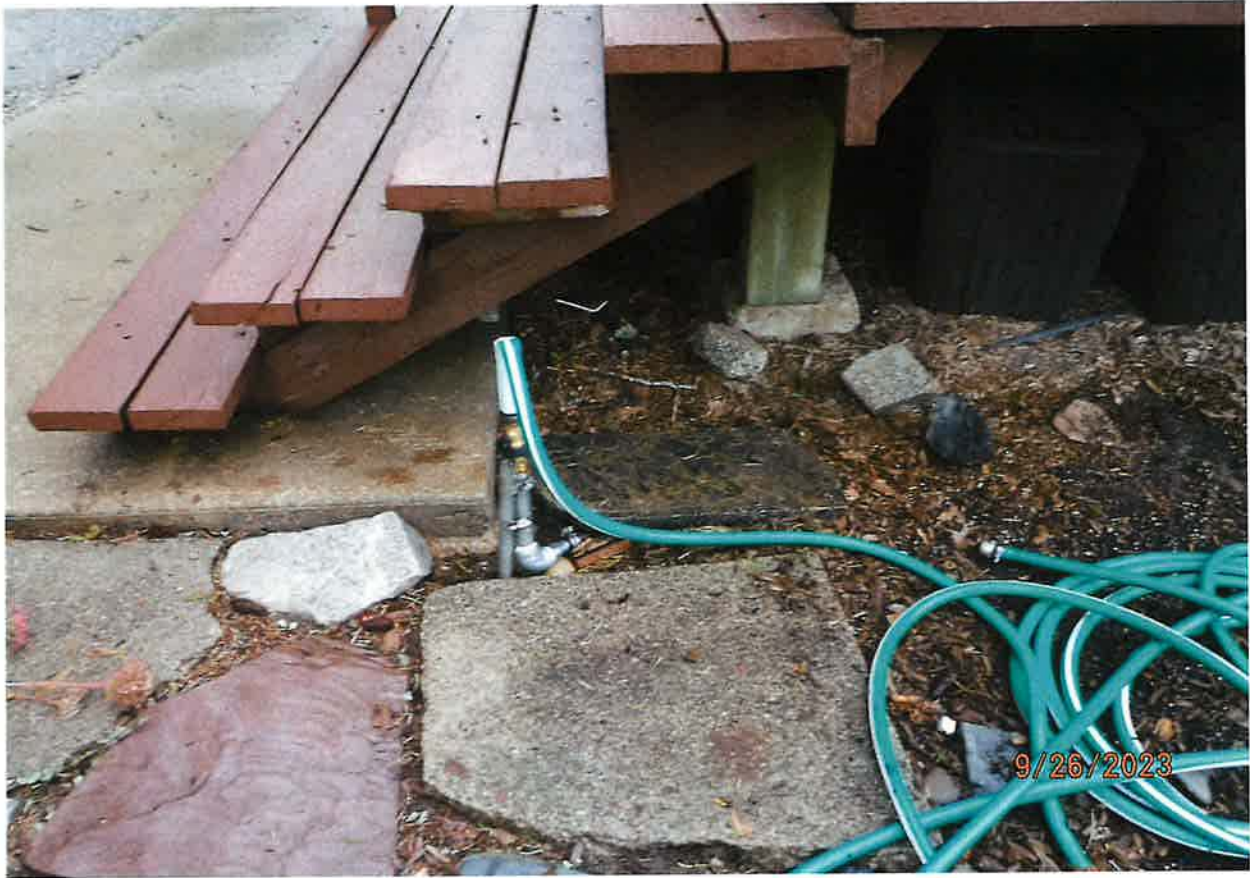
FROM PUMP BURIED POLY LINE ROUTES TO 2EA IRRIGATION HOSE BIB RISERS
