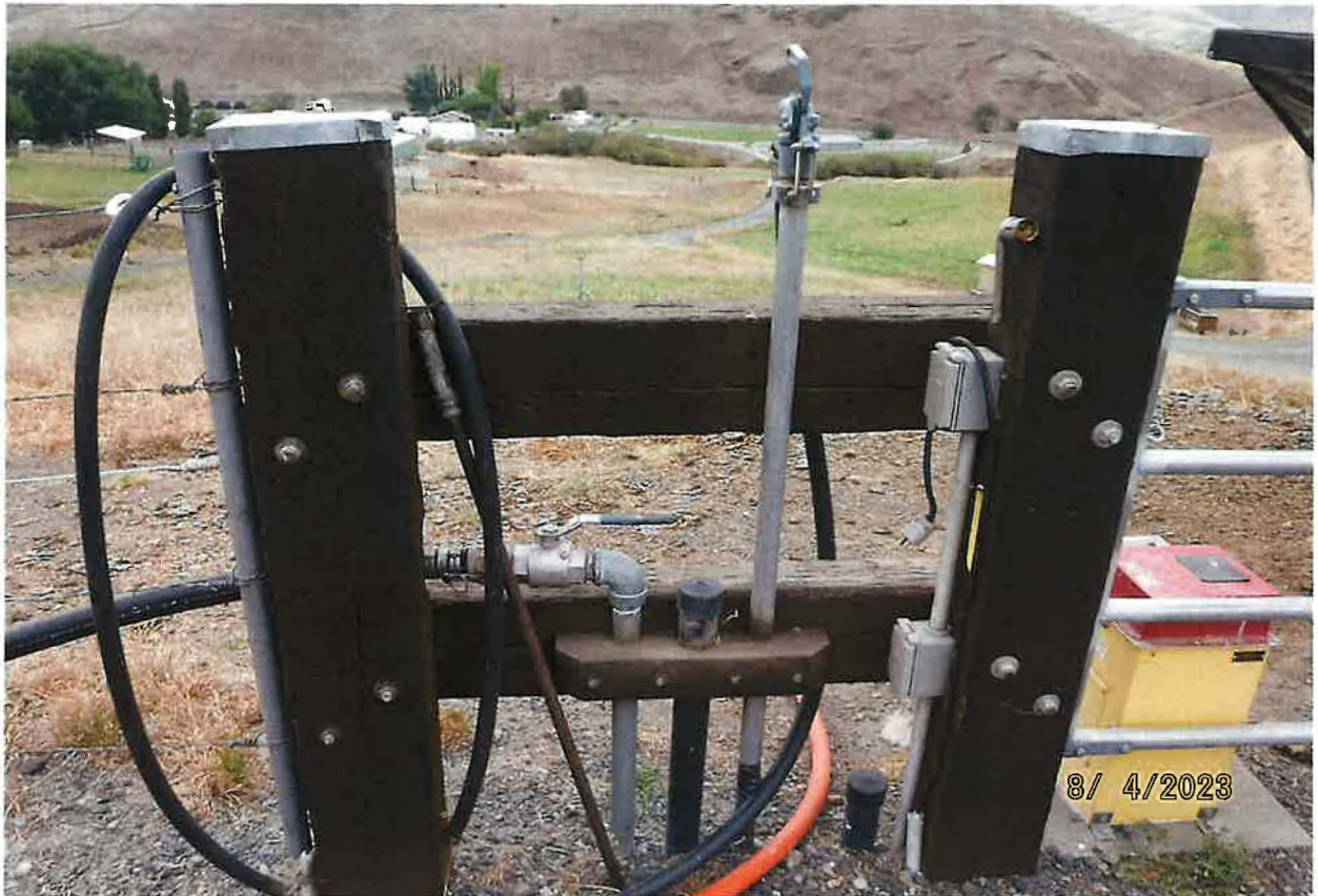
IRRIGATION POU – FROST FREE HYDRANT AND 1 INCH POLY PIPE RUNS TO PRESSURIZED SPRINKLERS & IMPACT SPRINKLERS.
