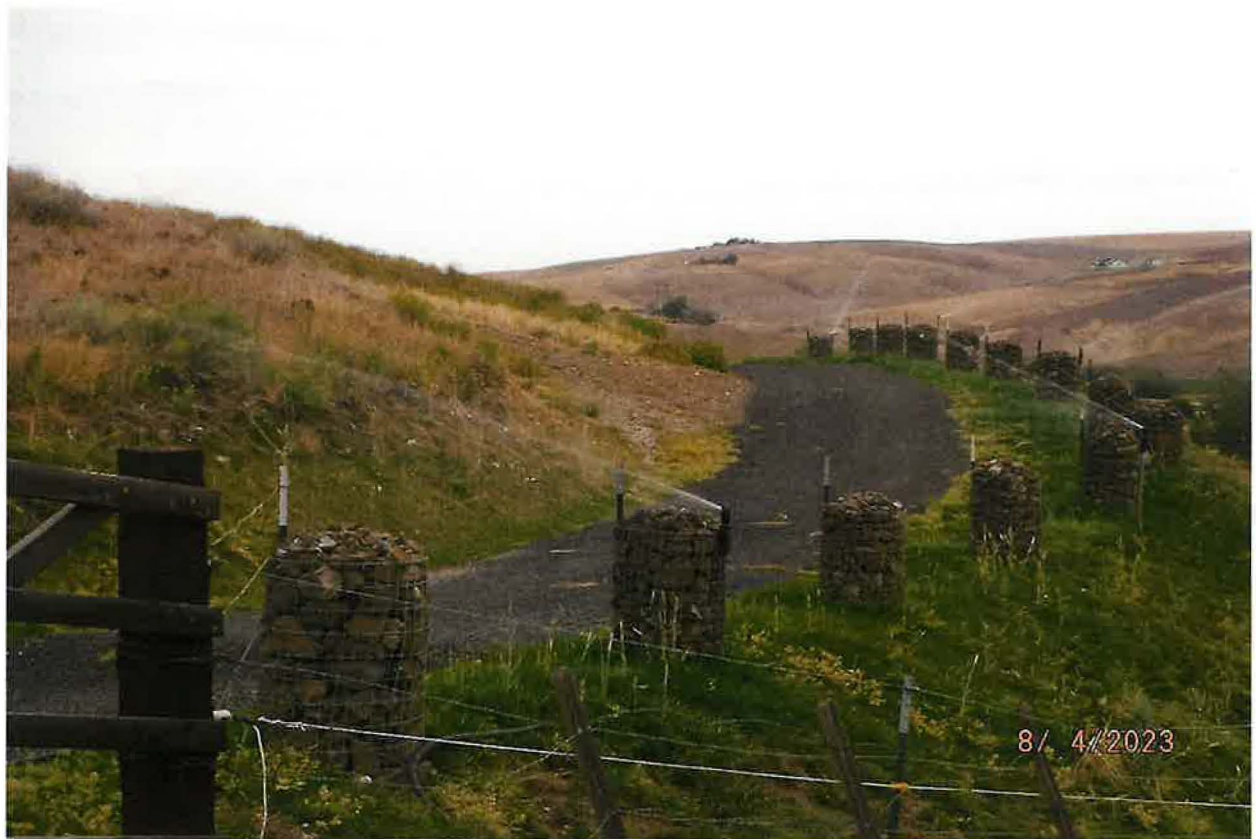
IRRIGATION POU – LOWER FIELDS IN POU
