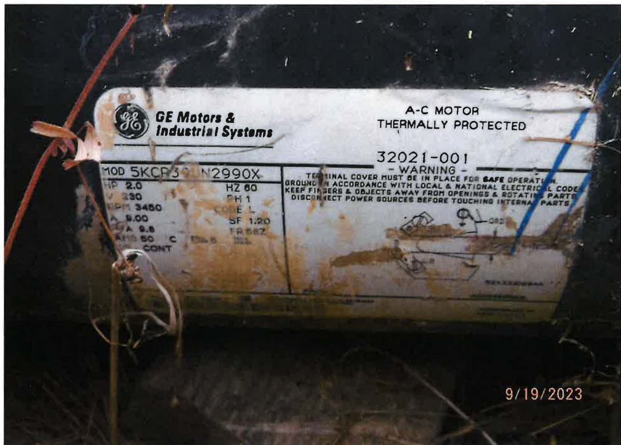
IRRIGATION FROM STORAGE DIVERTING WORKS – 2 HP WATER TRANSFER PUMP TO PRESSURIZED SPRINKLERS
