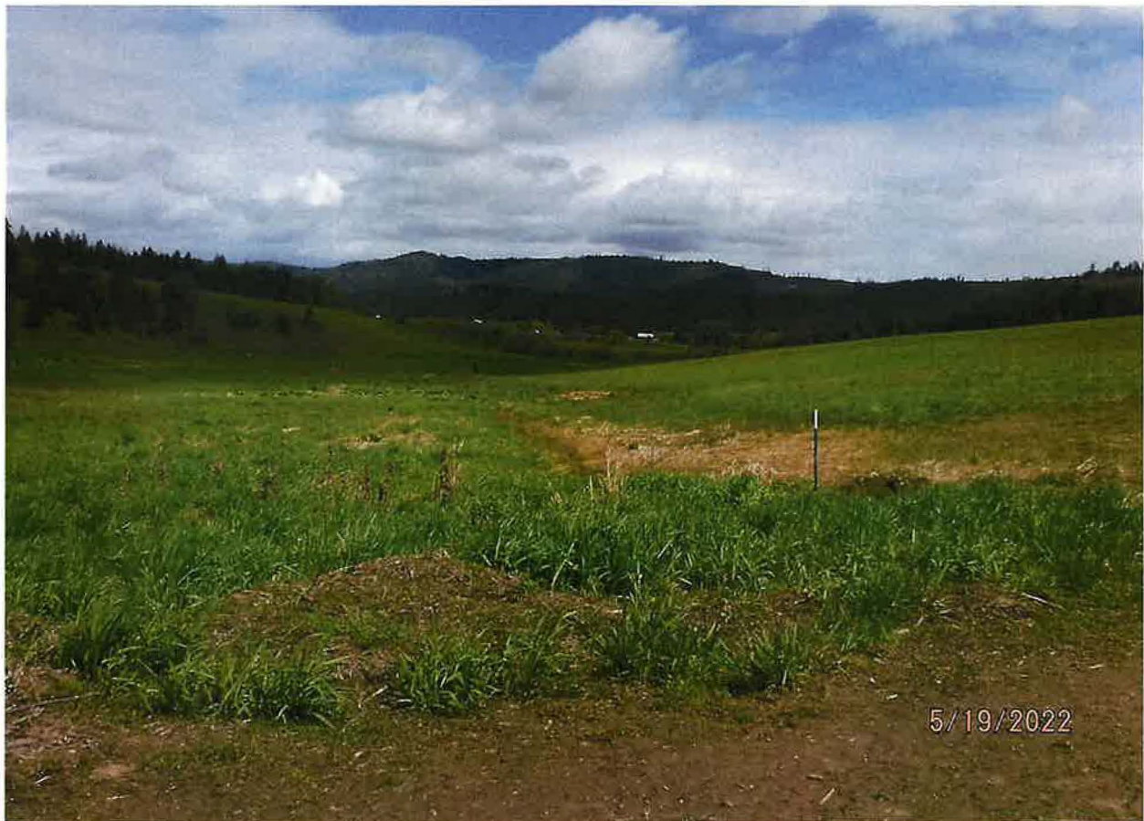
STANDING ON POND DAM WITH VIEW DOWNSTREAM TO THE EAST OF THE STORAGE POND
