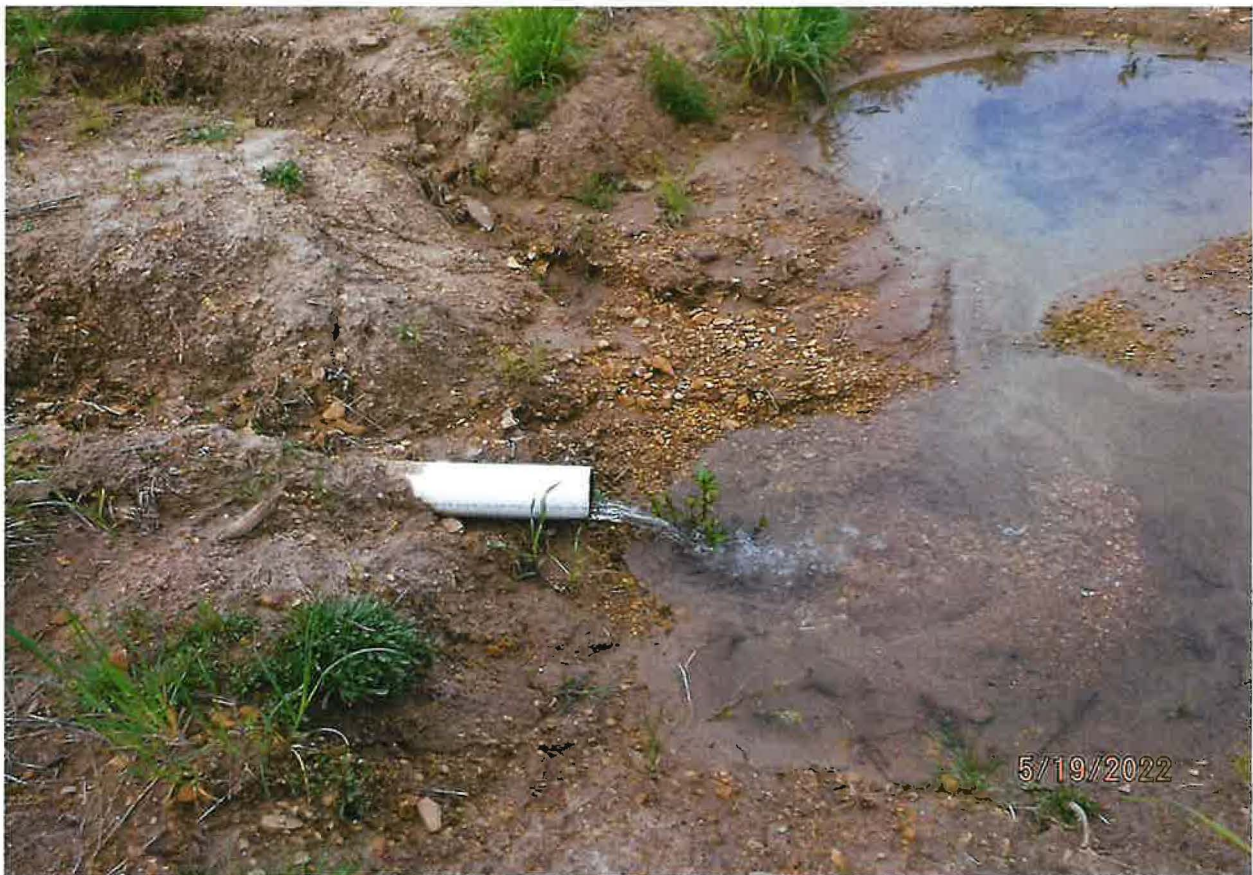
POD – GROUNDWATER FROM FRENCH DRAIN NEAR SHOP & DIVERSION TO STORAGE FOR GROUNDWATER SOURCE
