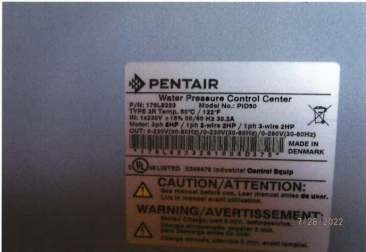
5 HP PENTAIR VARIABLE FREQUENCY DRIVE PUMP MOTOR INSTALLED; 62 PSI OPERATING PRESSURE FROM 2 PRESSURE TANKS
