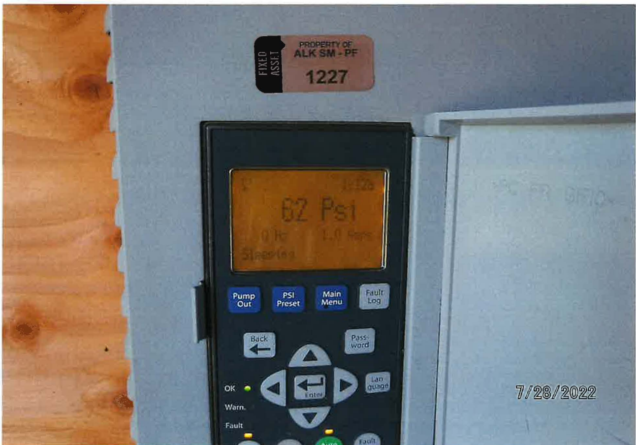
5 HP PENTAIR VARIABLE FREQUENCY DRIVE PUMP MOTOR INSTALLED; 62 PSI OPERATING PRESSURE FROM 2 PRESSURE TANKS
