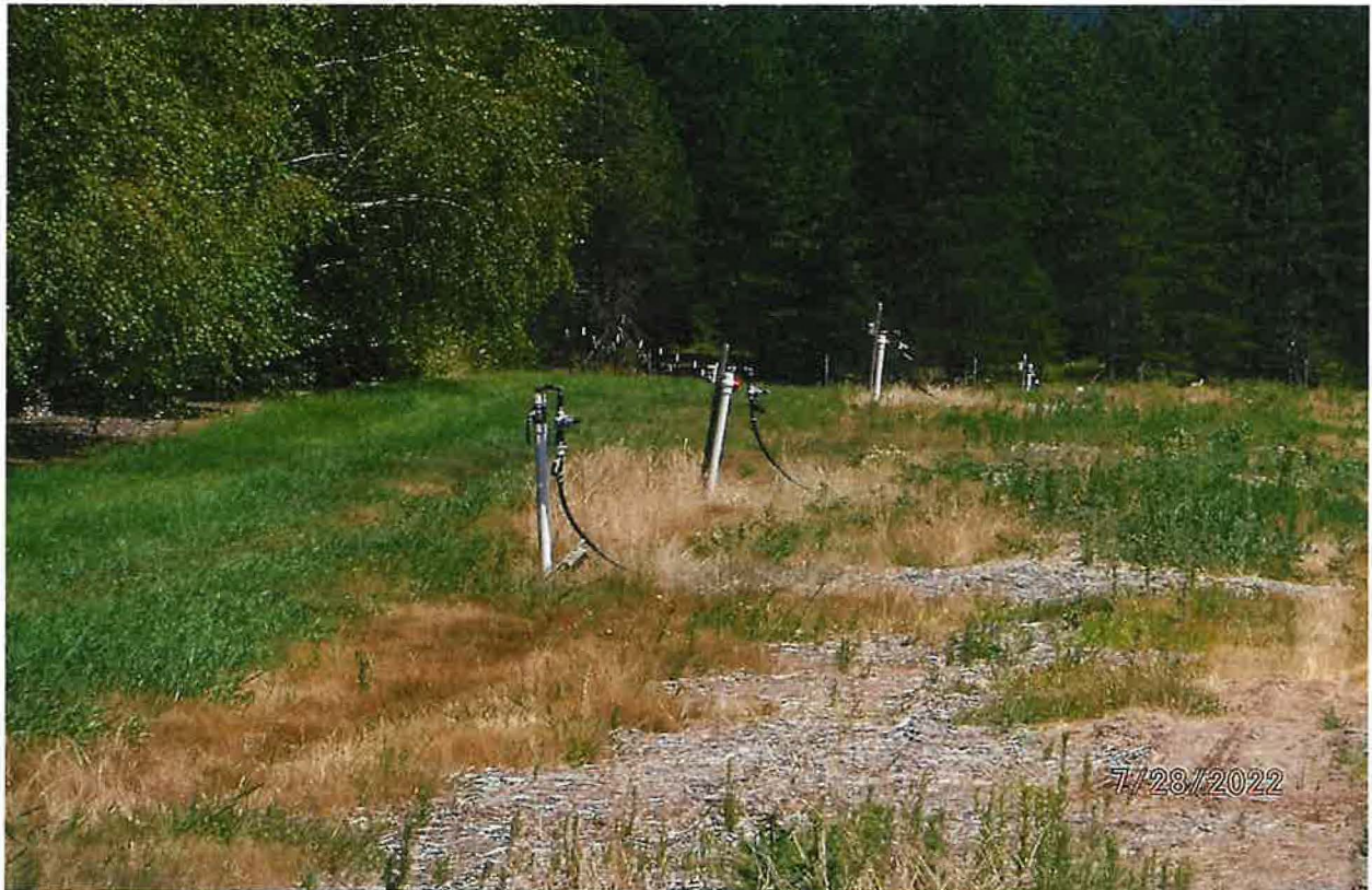
IRRIGATION POU – 1 ½ INCH RISER PIPES TO DRIP LINES, MICRO EMITTERS, & ¾ NOZZLE BRASS IMPACT SPRINKLERS
