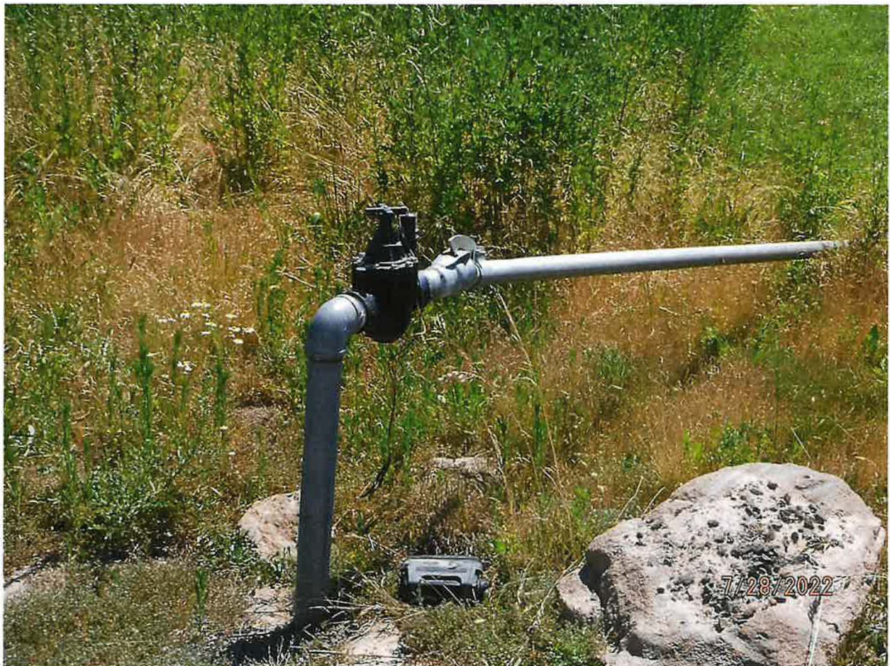
IRRIGATION POU – 1 ½ INCH RISER PIPES TO DRIP LINES, MICRO EMITTERS, & ¾ NOZZLE BRASS IMPACT SPRINKLERS
