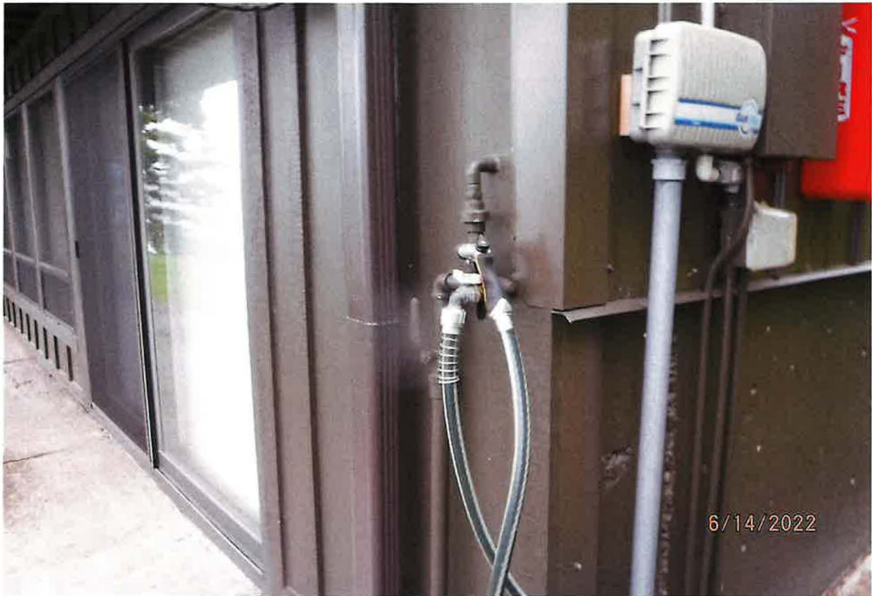
IRRIGATION SYSTEM CONTROL PANEL – RAIN DIAL SYSTEM
