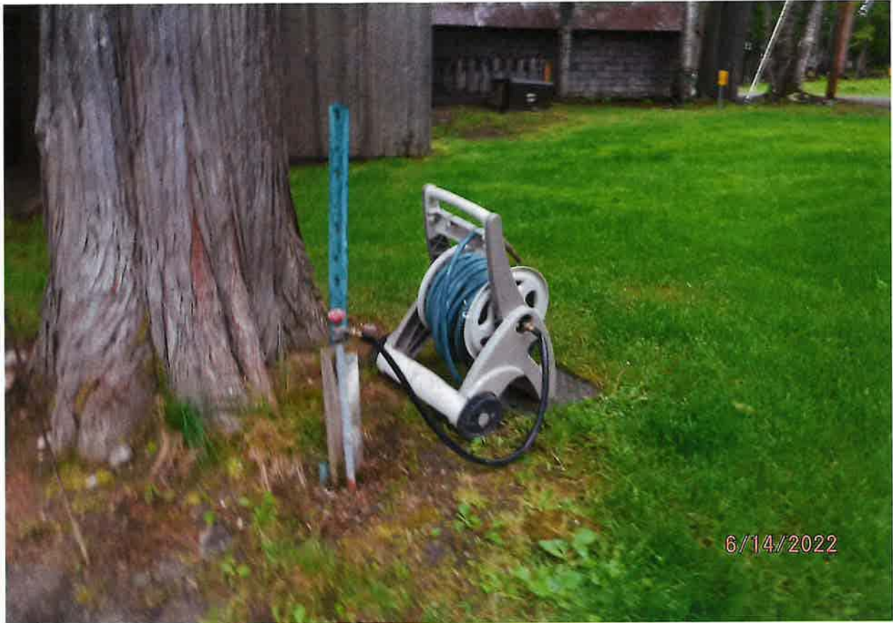
IRRIGATION POU – RISER PIPE TO HOSE & SPRINKLER
