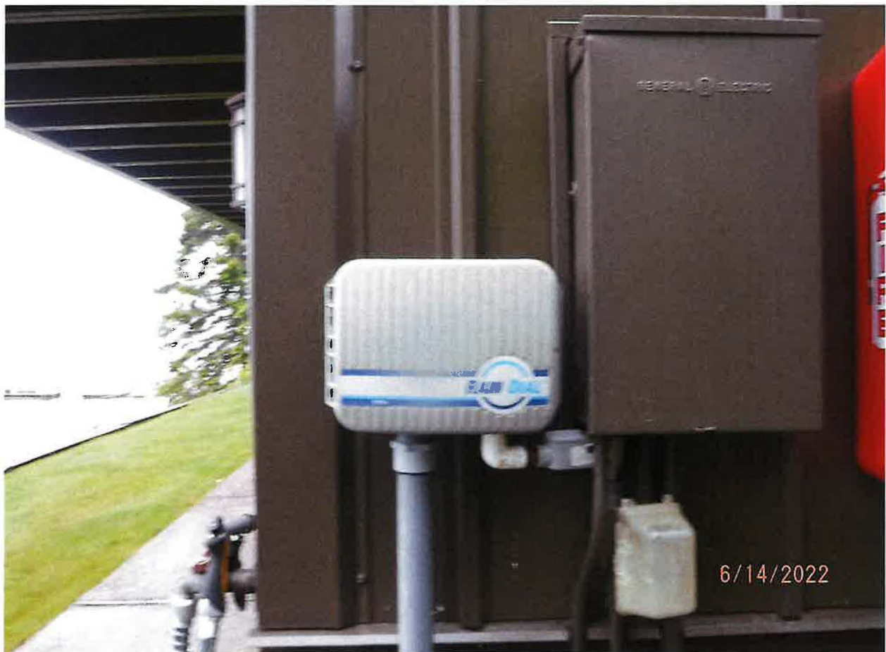
IRRIGATION SYSTEM CONTROL PANEL – RAIN DIAL SYSTEM
