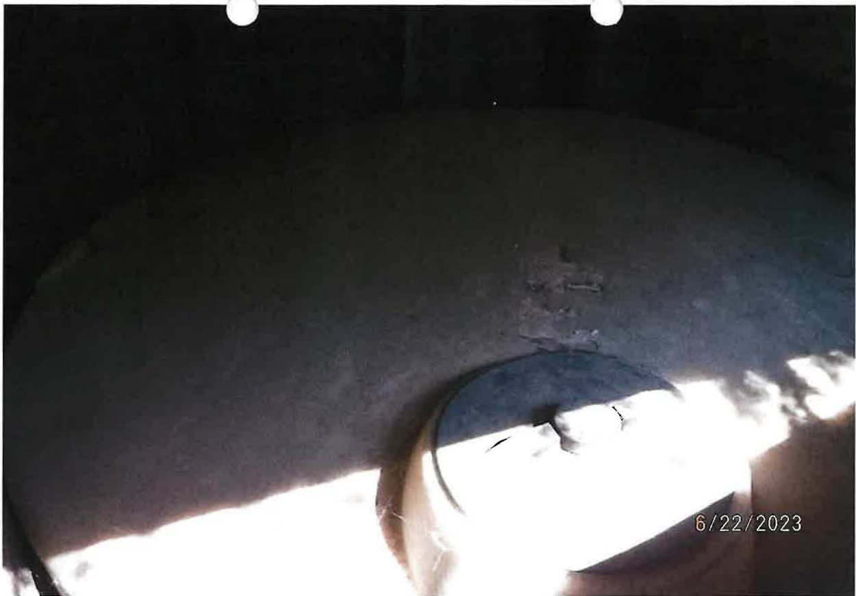
LARGE STORAGE TANK USED AT LAKEFRONT HOME – FILLED USING PORTABLE TANK FROM POD ON HILL AND TRANSPORTED BY VEHICLE W/TRAILER DOWN TO HOME.
