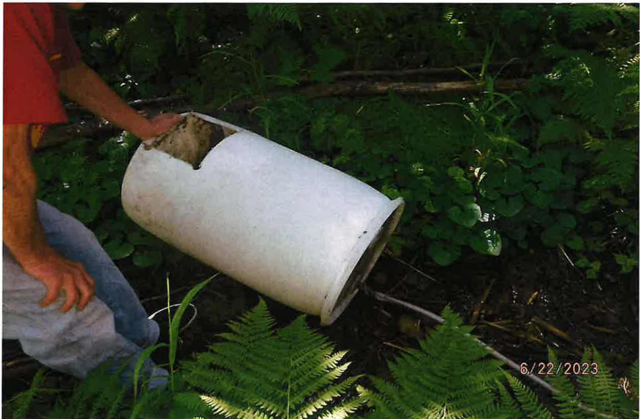
POD – REPURPOSED PLASTIC DRUM USED TO CAPTURE STREAM WATER AND GRAVITY PIPE BY HOSE TO WATER USES
