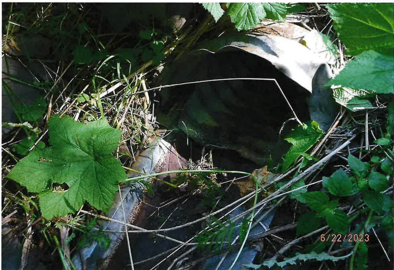
POD – SEASONAL CREEK (DRY AT TIME OF EXAM) WATER COLLECTED BELOW CULVERT
