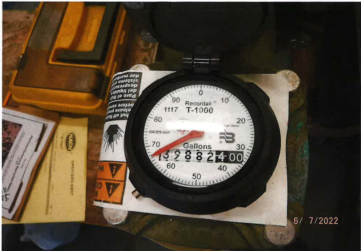
BADGER METER – FLOWMETER INSTALLED IN DIVERTING WORKS FOR WELL D0072339
