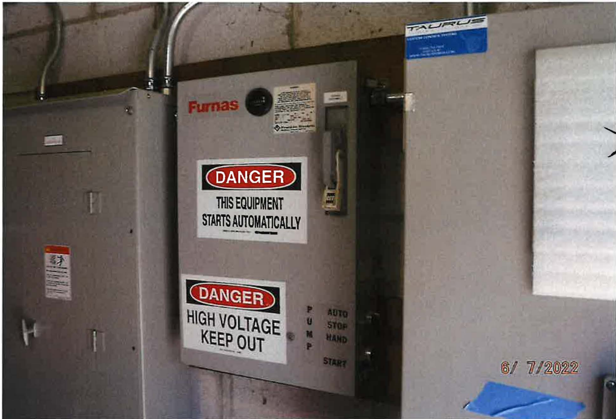
PUMP CONTROL PANEL, IN PROCESS INSTALLATION OF SCADA SYSTEM (R/H PANEL IN PHOTO)
