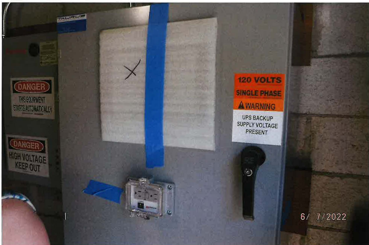
CITY OF STITES IN PROCESS INSTALLING SCADA SYSTEM FOR WATER SYSTEM MANAGEMENT
