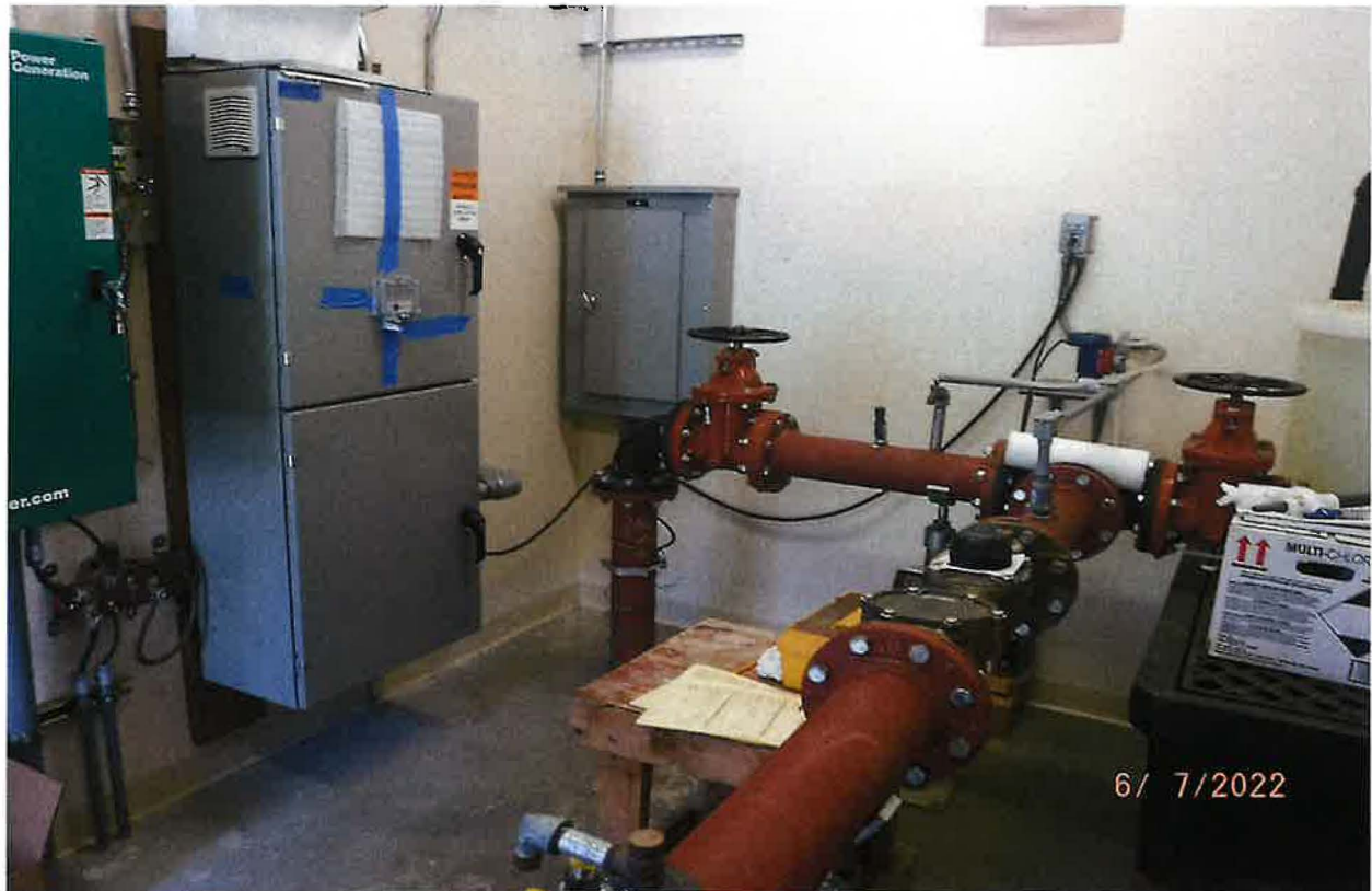
DIVERTING WORKS FOR WELL D0072339; SCADA SYSTEM INSTALL IN-PROCESS
