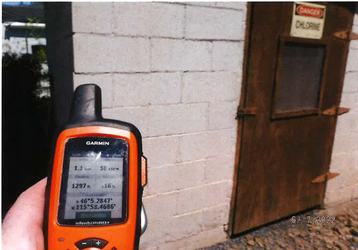
WELL HOUSE / PUMP HOUSE FOR GROUNDWATER WELL IN NE¼NE¼, SEC. 29, TWP 32N, RGE 04E
