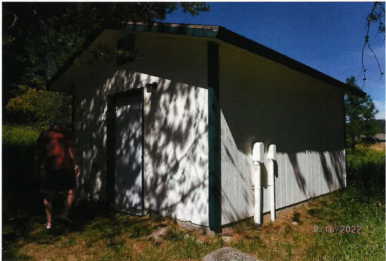
MAIN SERVICE LINE ROUTES DIRECT TO PUMP HOUSE AND PRESSURE TANKS PRIOR TO DISTRIBUTION TO POU
