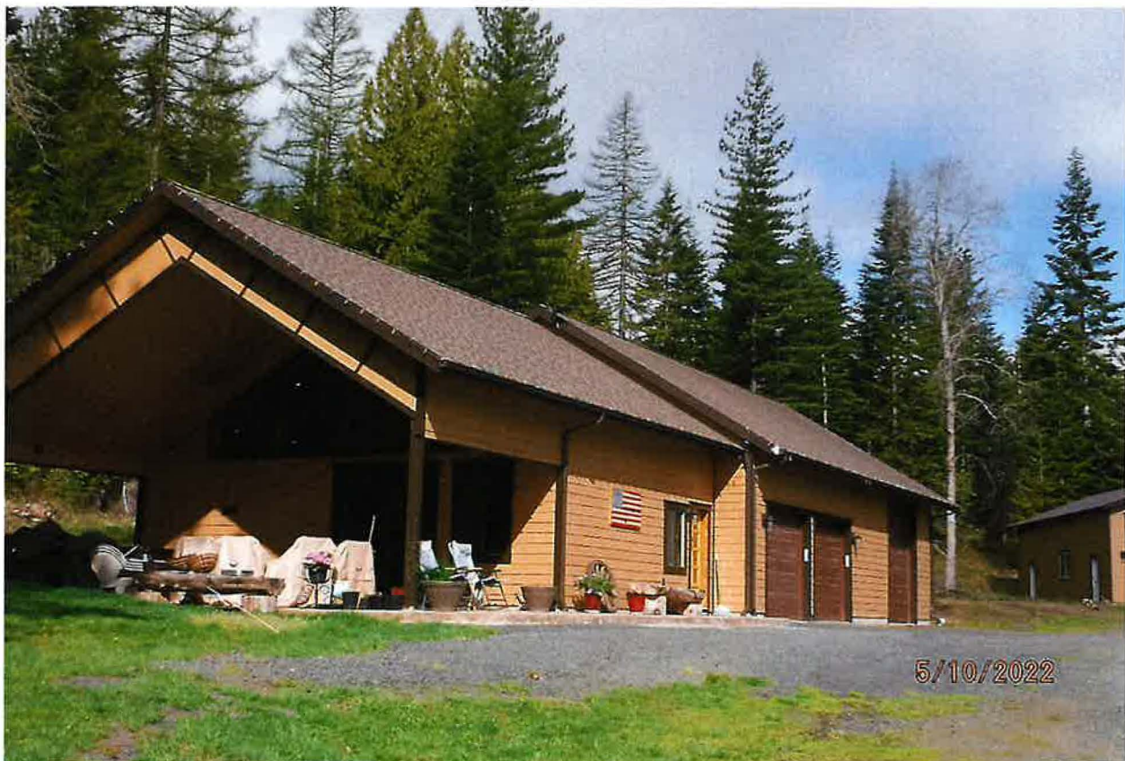
POU – DOMESTIC SHOP HOME
