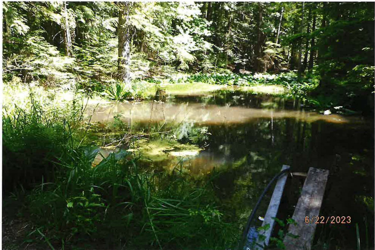
POD – POND WITH EARTHEN DAM AND CUVLVERT OVERFLOW DISCHARGE PIPE
