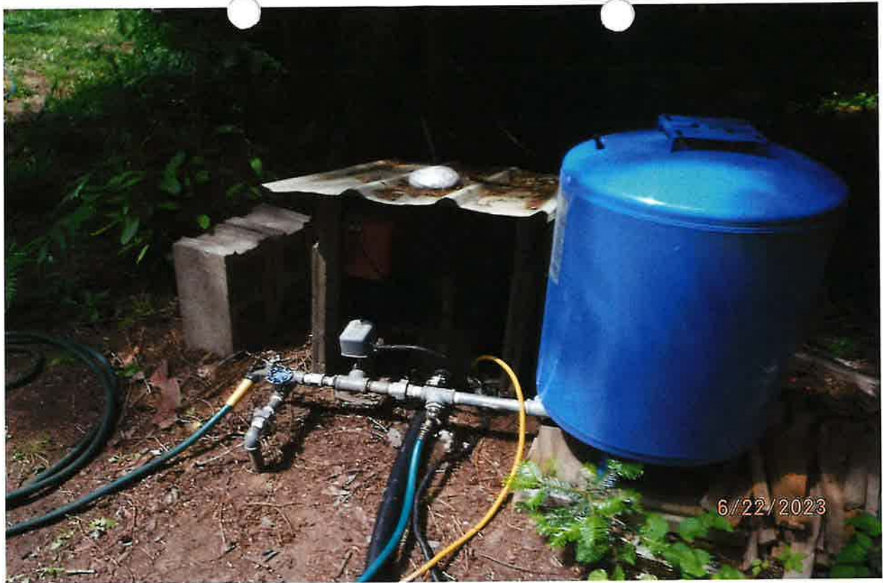
IRRIGATION FROM STORAGE DIVERTING WORKS \frac{1}{2} - \frac{3}{4} HP CENTURY PUMP TO HOSE AND SPRINKLERS
