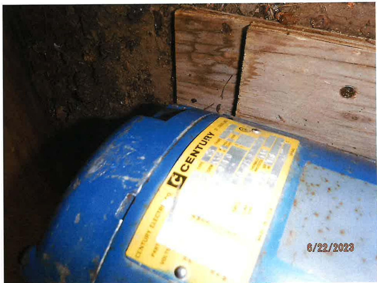
IRRIGATION FROM STORAGE DIVERTING WORKS \frac{1}{2} - \frac{3}{4} HP CENTURY PUMP TO HOSE AND SPRINKLERS
