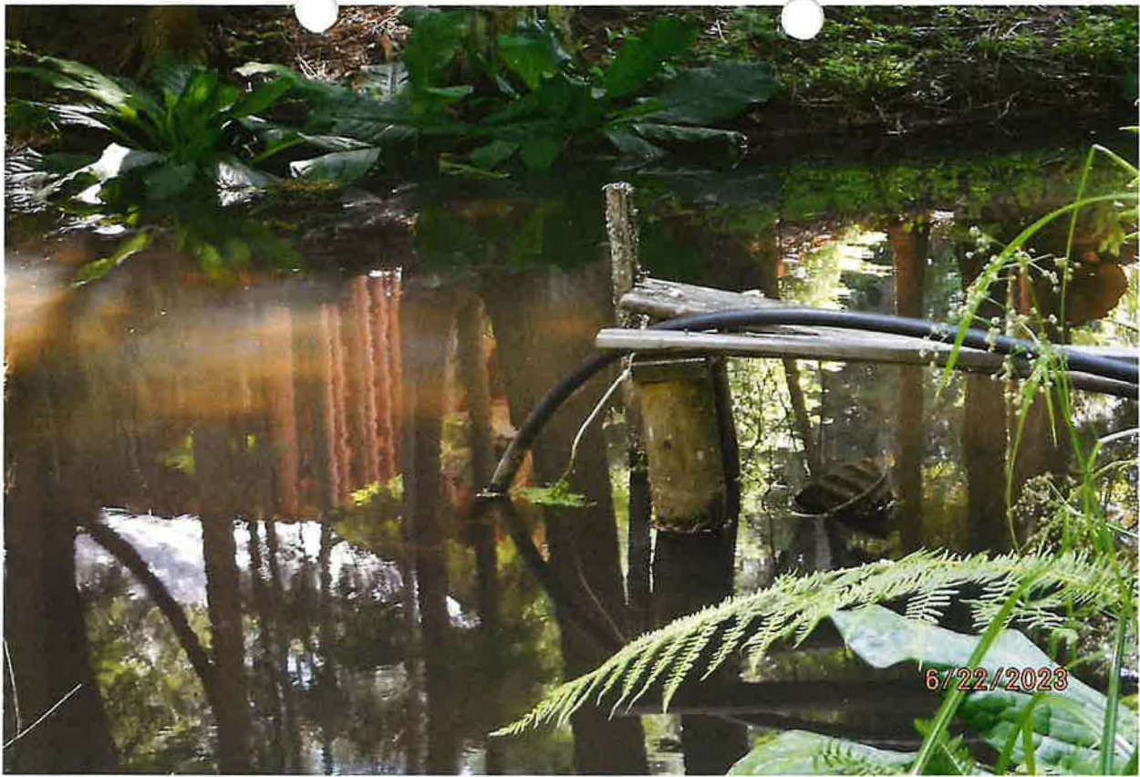
POU – IRRIGATION STORAGE & FIRE PROTECTION STORAGE POND WITH OVERFLOW DEVICE
