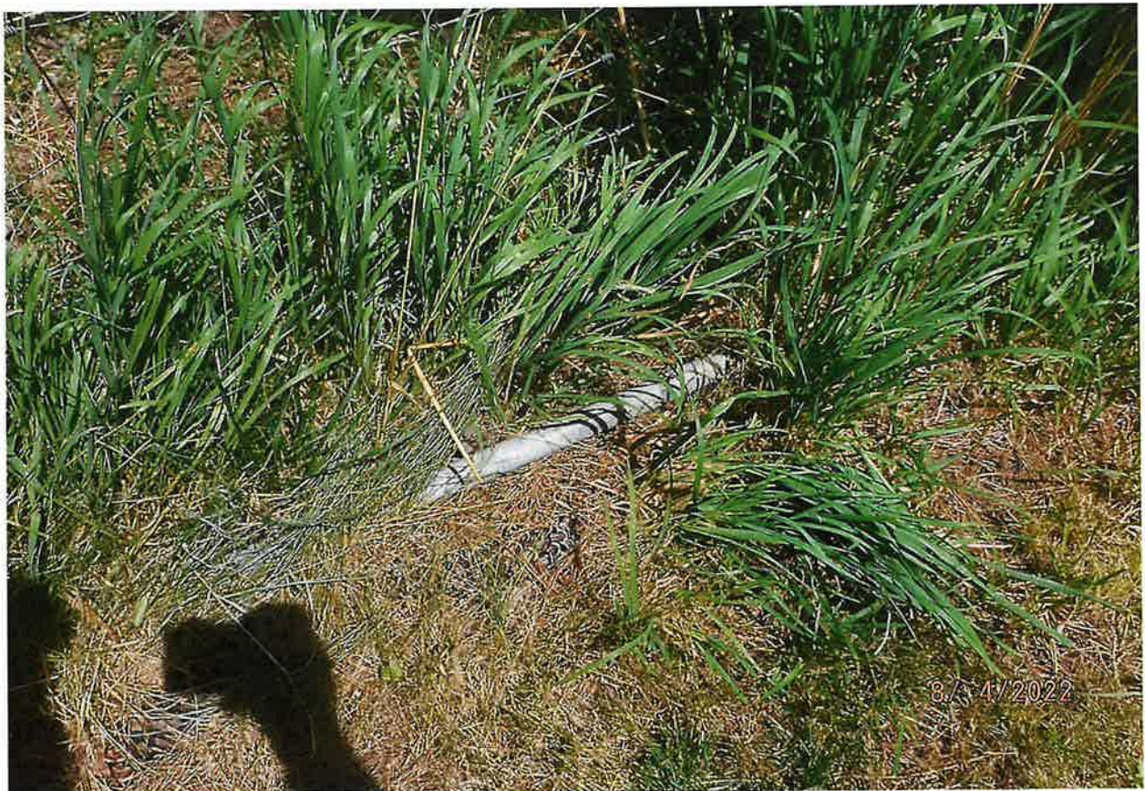
1 INCH IRRIGATION PIPE ROUTES ALONG FENCE WITH RISERS AT 50 YARD INTERVALS
