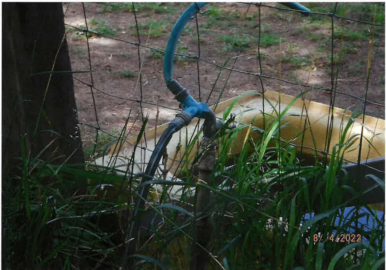
IRRIGATION RISER PIPE TO HOSE BIB ATTACHMENT
