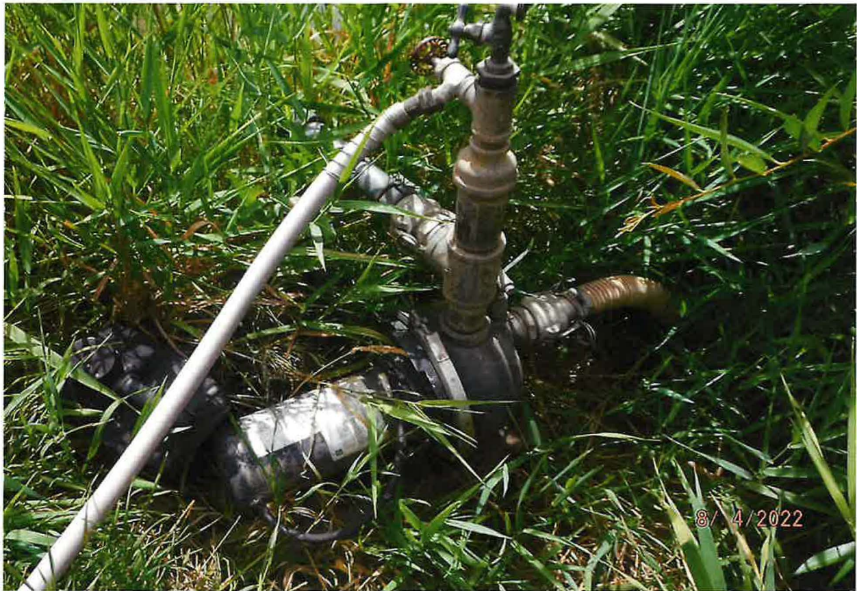
DIVERTING WORKS – 2 HP PUMP TO 1 ½ INCH MAIN LINE TO 1 INCH IRRIGATION RUNS AND HOSE/SPRINKLER ATTACHMENT POINTS AT INTERVAL
