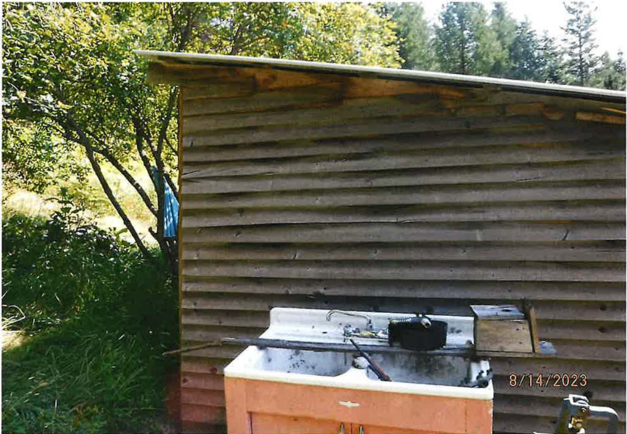
SMALL WOODEN ENCLOSURE HOUSES GW WELL
