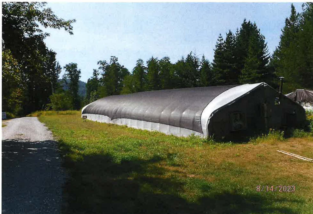
IRRIGATION POU – 2 OF 2 LARGE HOOP GROW STRUCTURES
