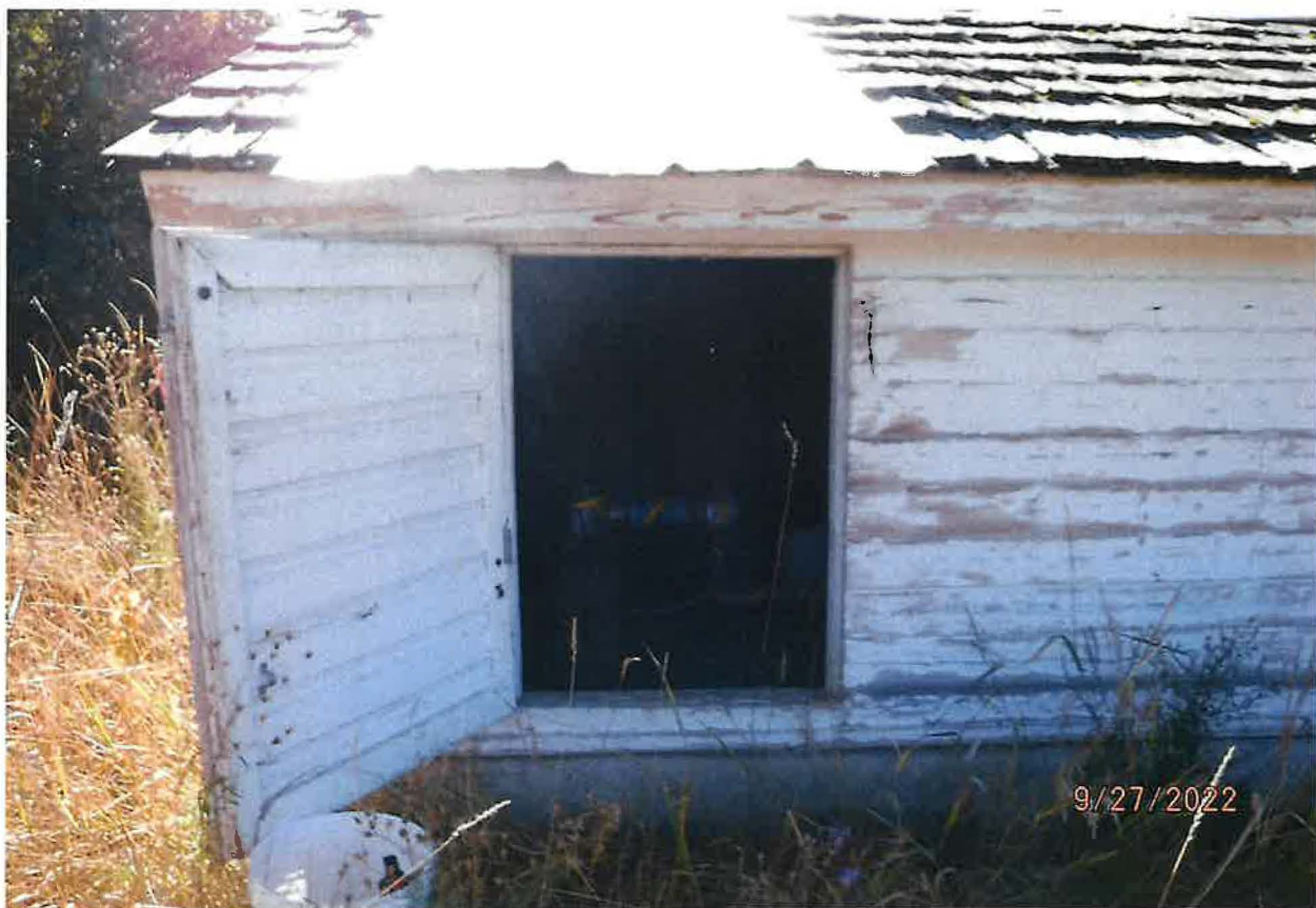
POD – GROUNDWATER WELL LOCATED WITHIN WELL HOUSE
