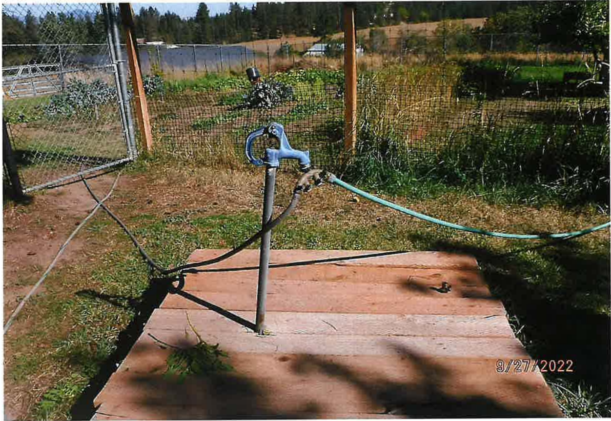
EXAMPLE – FROST FREE HYDRANT WITH HOSE SPLITTERS USED FOR IRRIGATION AT POU
