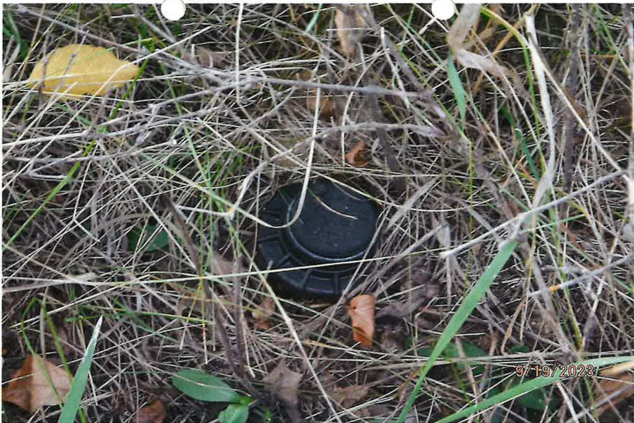
IRRIGATION POU – Lot 5, The Cove at Strong Creek Sub. RP02854000005A0A – FRUIT TREES WATERED ON ON PARCEL BY PRESSURIZED IRRIGATION SYSTEM FROM HYDRANT.
