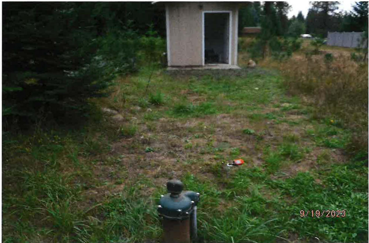
WELL HEAD CO-LOCATED WITH SMALL PUMP STATION
