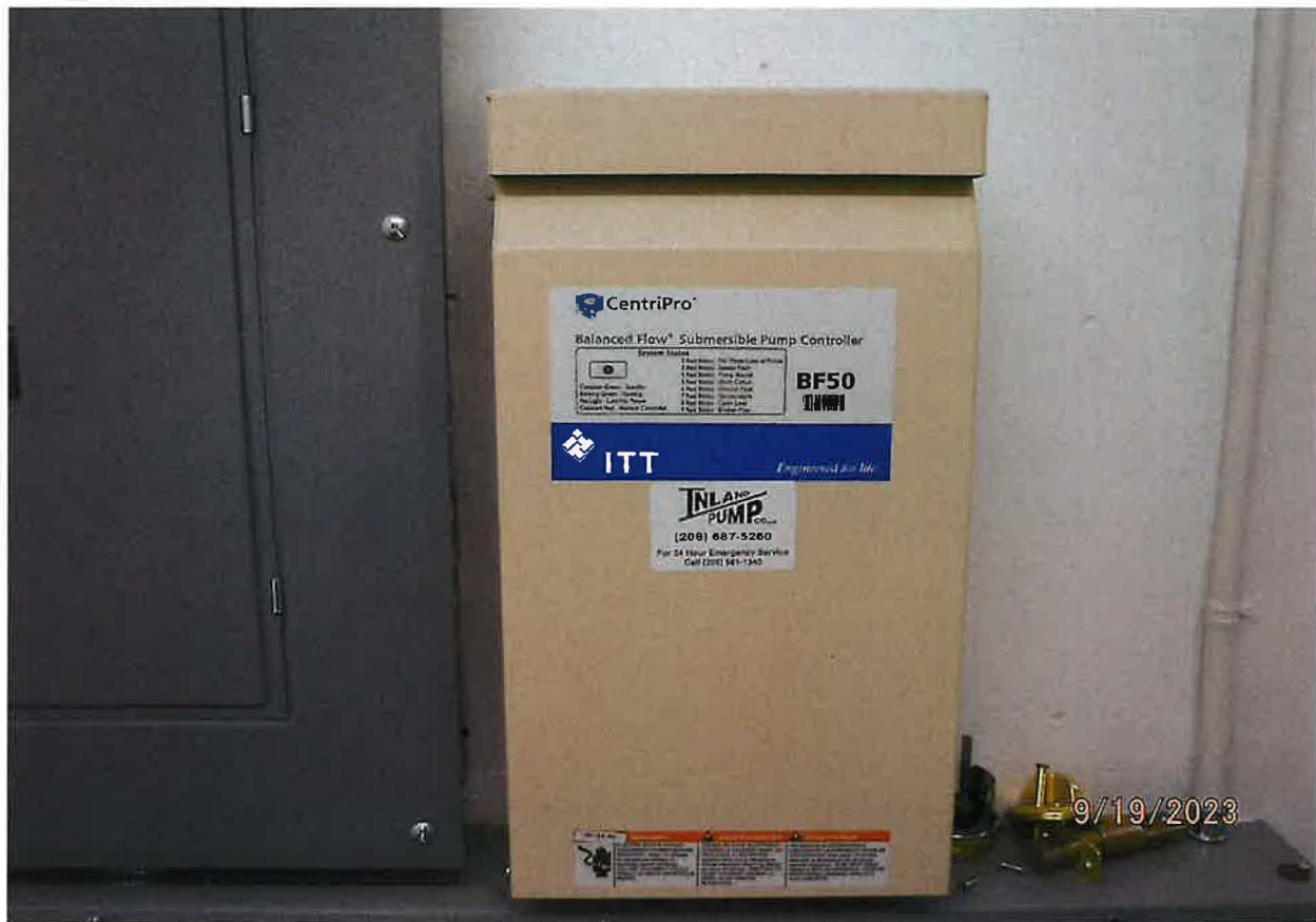
GOULDS PUMP WITH CENTRIPRO PUMP MOTOR INSTALLED IN WELL – BF50 5 HP MOTOR SET TO 80 Hz
