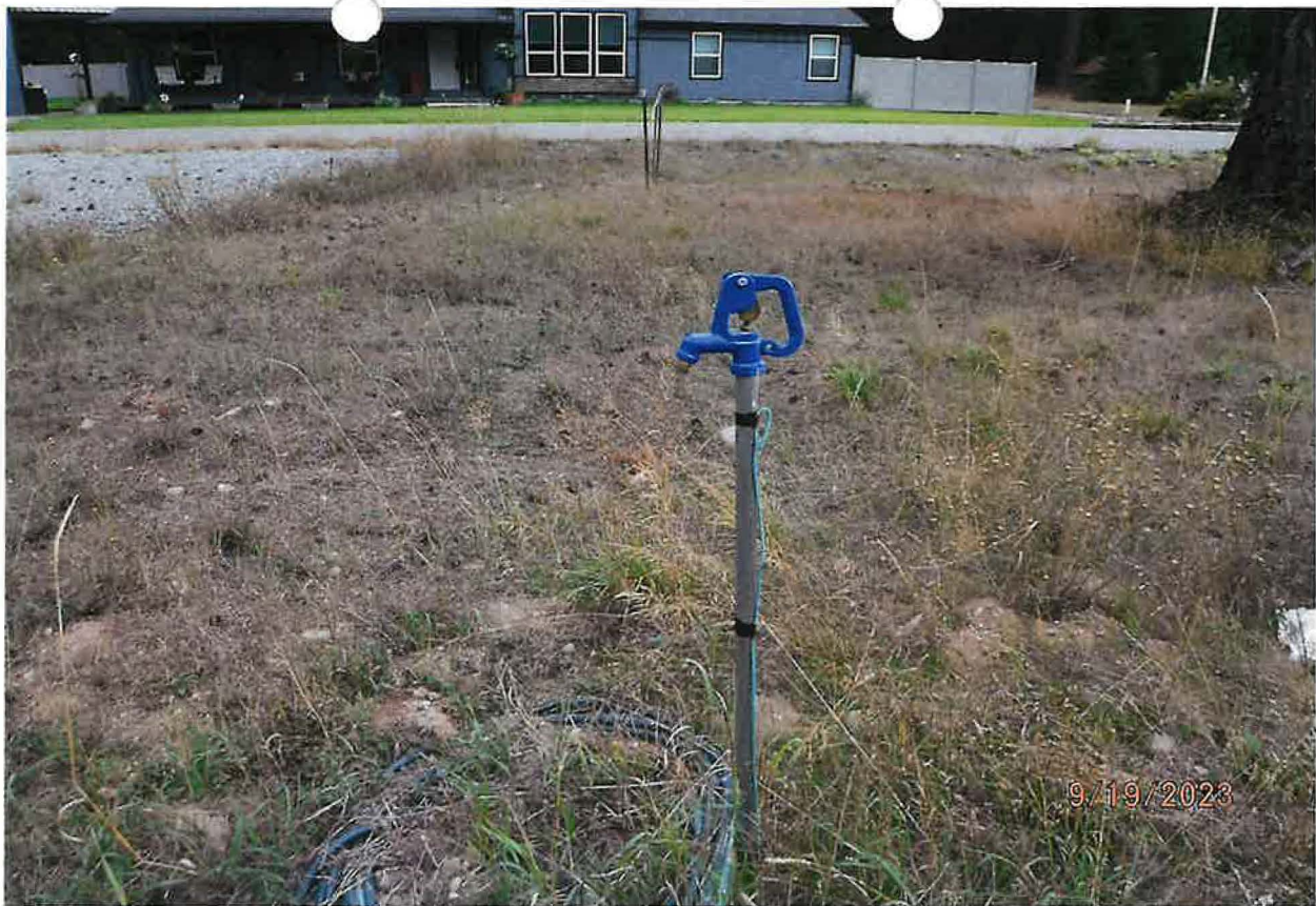
DOMESTIC POU – STUB-IN – Lot 5A Replat, The Cove at Strong Creek Sub. RP0285400005A0A
