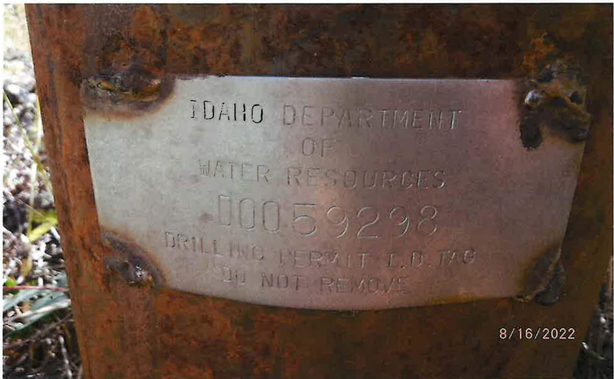
GROUNDWATER WELL D0059298 (NOT SERVICE CONNECTED TO WATER SYSTEM AT TIME OF EXAM)
