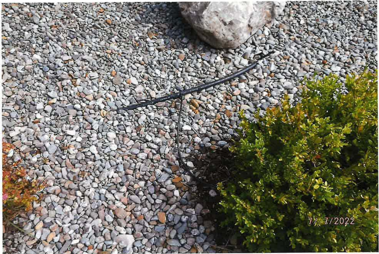
MICRO EMITTERS USED FOR LANSCAPING PLANTS
