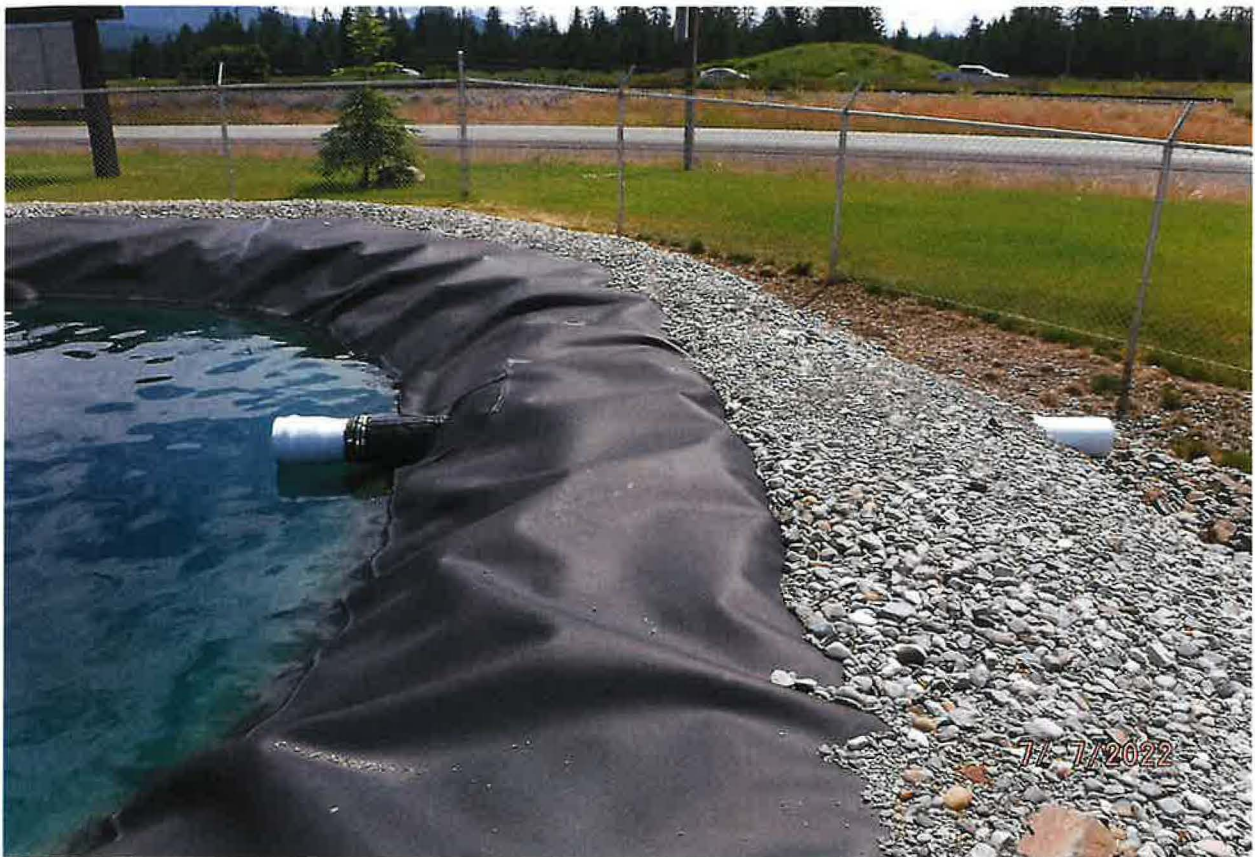
OVERFLOW DEVICE FOR STORAGE POND
