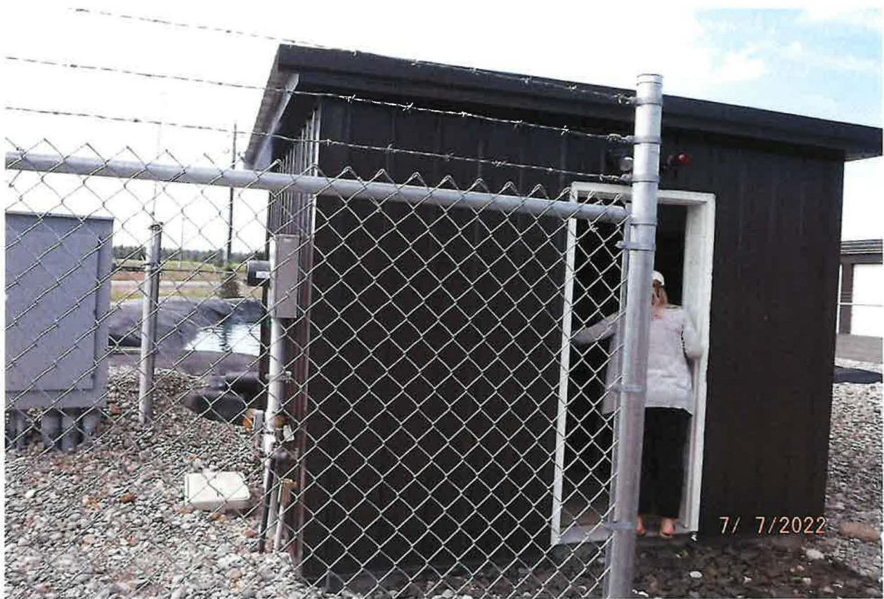
PUMP CONTROL STATION
