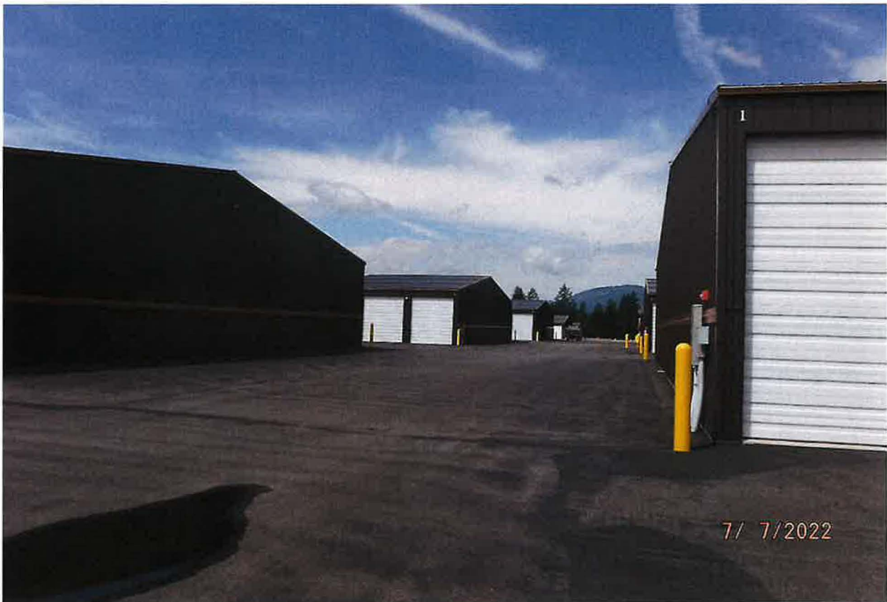
COMMERCIAL POU – STORAGE UNIT FACILITY; WATER USED FOR CLEANING OF UNITS & EQUIPMENT
