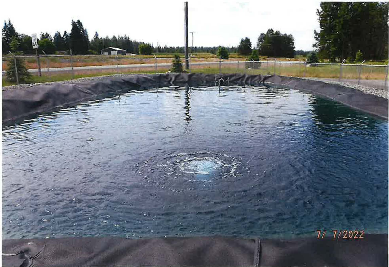
FIRE PROTECTION STORAGE POU – LINED POND
