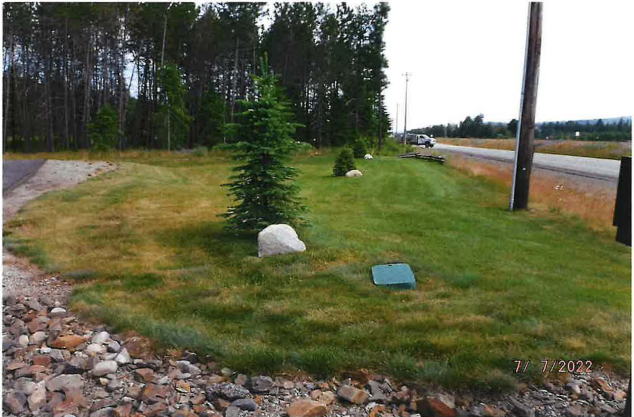
IRRIGATION POU – LAWN SPACE WITH ZONE CONTROL BOX
