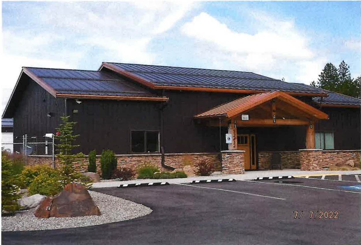
DOMESTIC POU – MAIN OFFICE/RESIDENCE LOCATED ON PROPERTY
