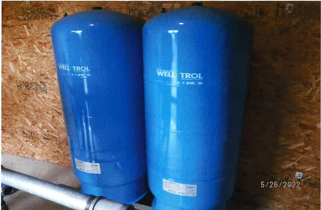
2EA PRESSURE TANKS INCLUDED IN DIVERTING WORKS
