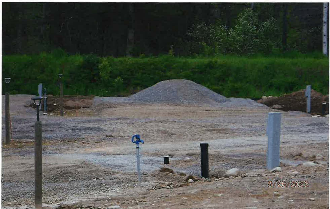
ADDING ADDITIONAL FINISH ROCK TO SITES – UPGRADED SOME SEPTIC SYSTEM COMPONENTS AT TIME OF EXAM
