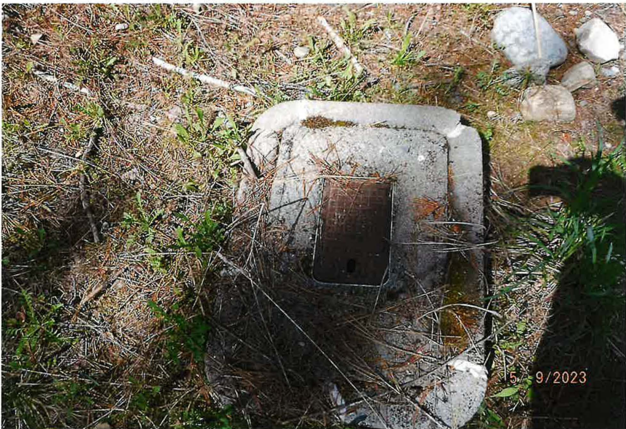
EXAMPLE – 1 OF 6 WATER LINE STUB OF MAIN SERVICE PIPELINE
