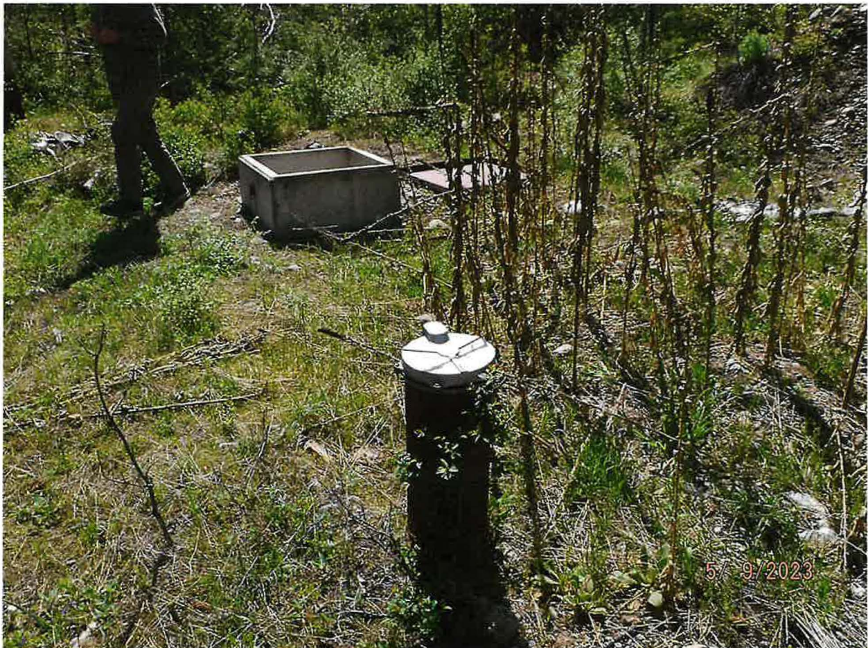
POD – GW WELL 96-N-105-000; VAULT IN BACKGROUND HOUSES DIVERTING WORKS COMPONENTS
