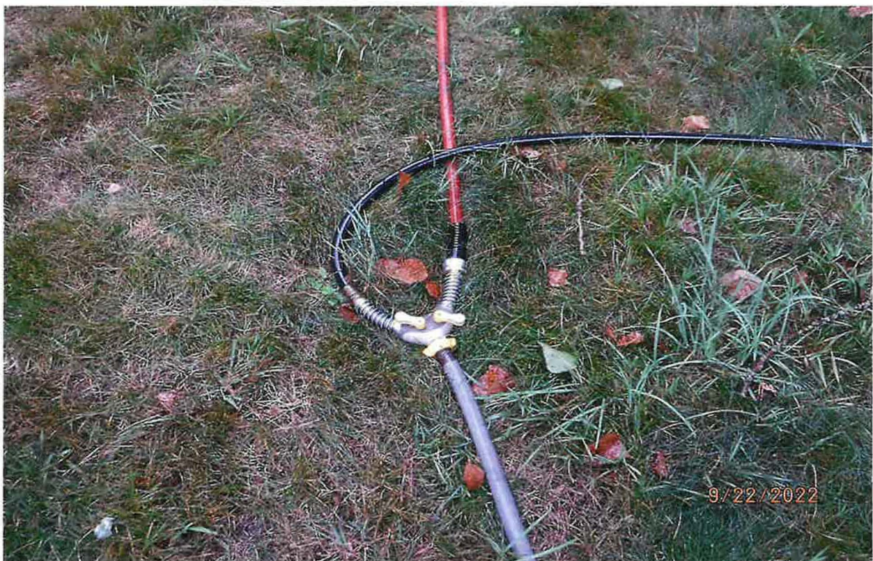
IRRIGATION SYSTEM INCORPORATES TWO LONG RUNS OF GARDEN HOSE WITH SPLITTERS AT 100 FT INTERVALS & HOSE TO TRIPOD SPRINKLERS FOR USE
