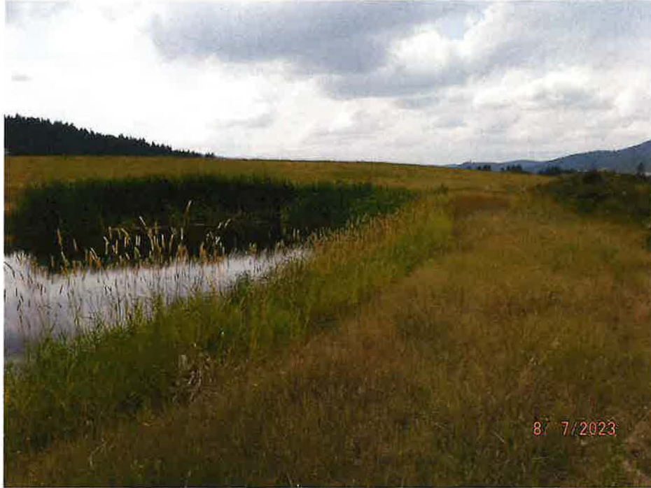
POD - EARTHEN DAM FOR POND
