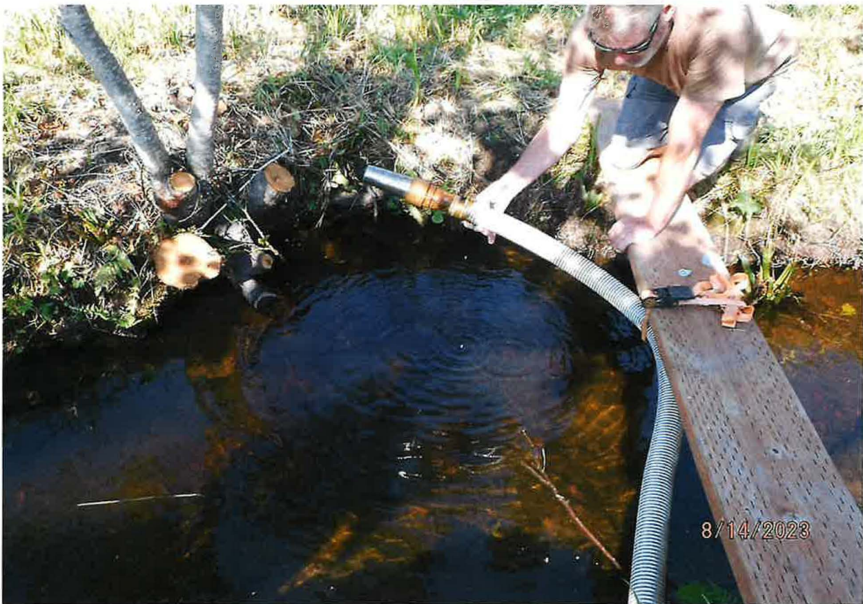
POD – SCREENED FLEXIBLE INTAKE HOSE LOCATED IN CREEK
