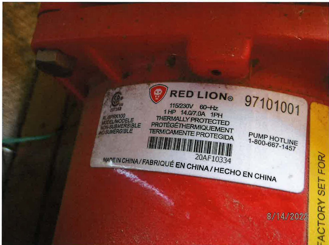
1 HP RED LINE TRANSFER PUMP WITH PRESSURE POT USED AS DISTRIBUTION PUMP FOR IRRIGATION SYSTEM
