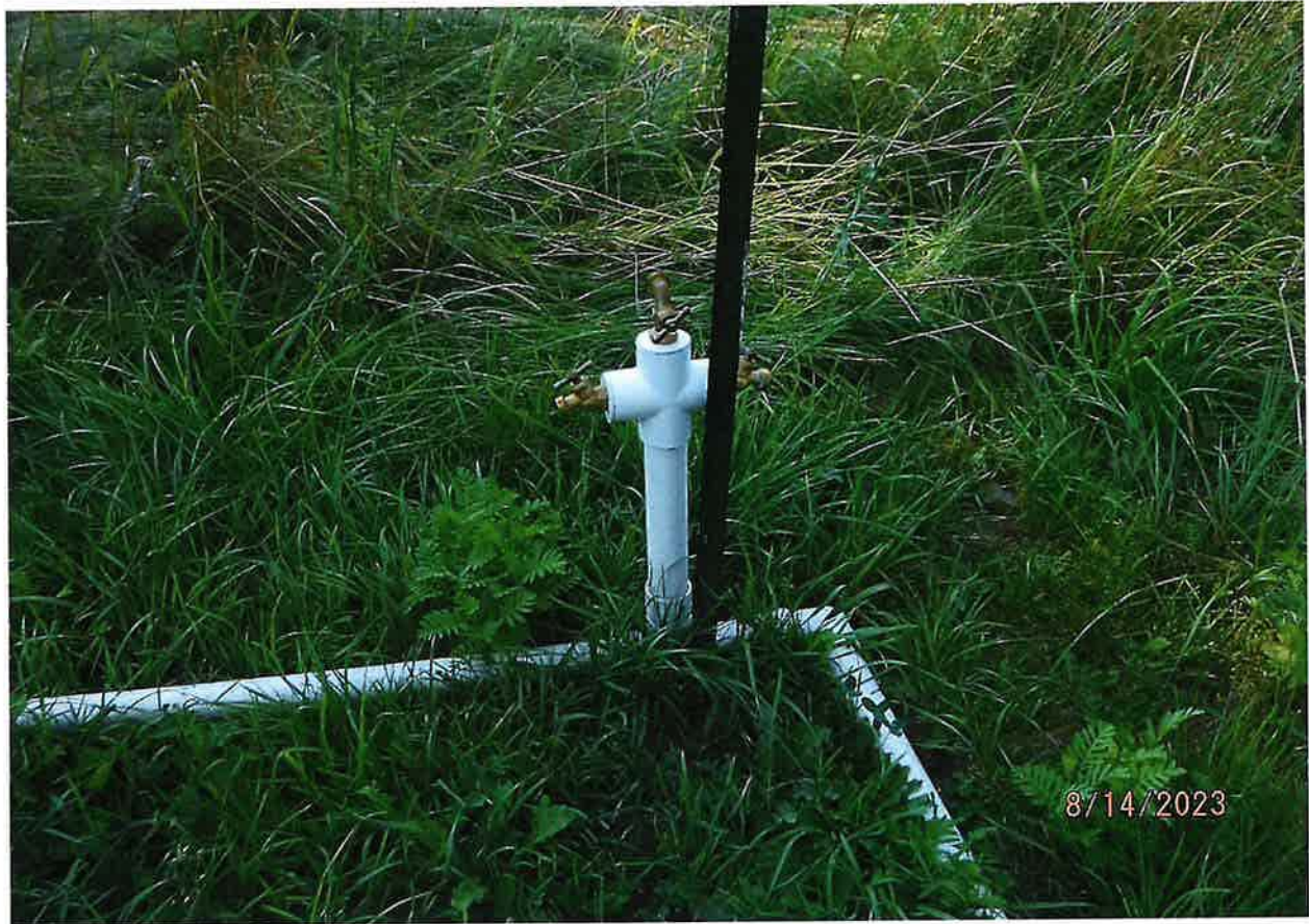
EXAMPLE – IRRIGATION POU WATER CONVEYANCE SYSTEM – RISER PIPES WITH THREE HOSE BIBS
