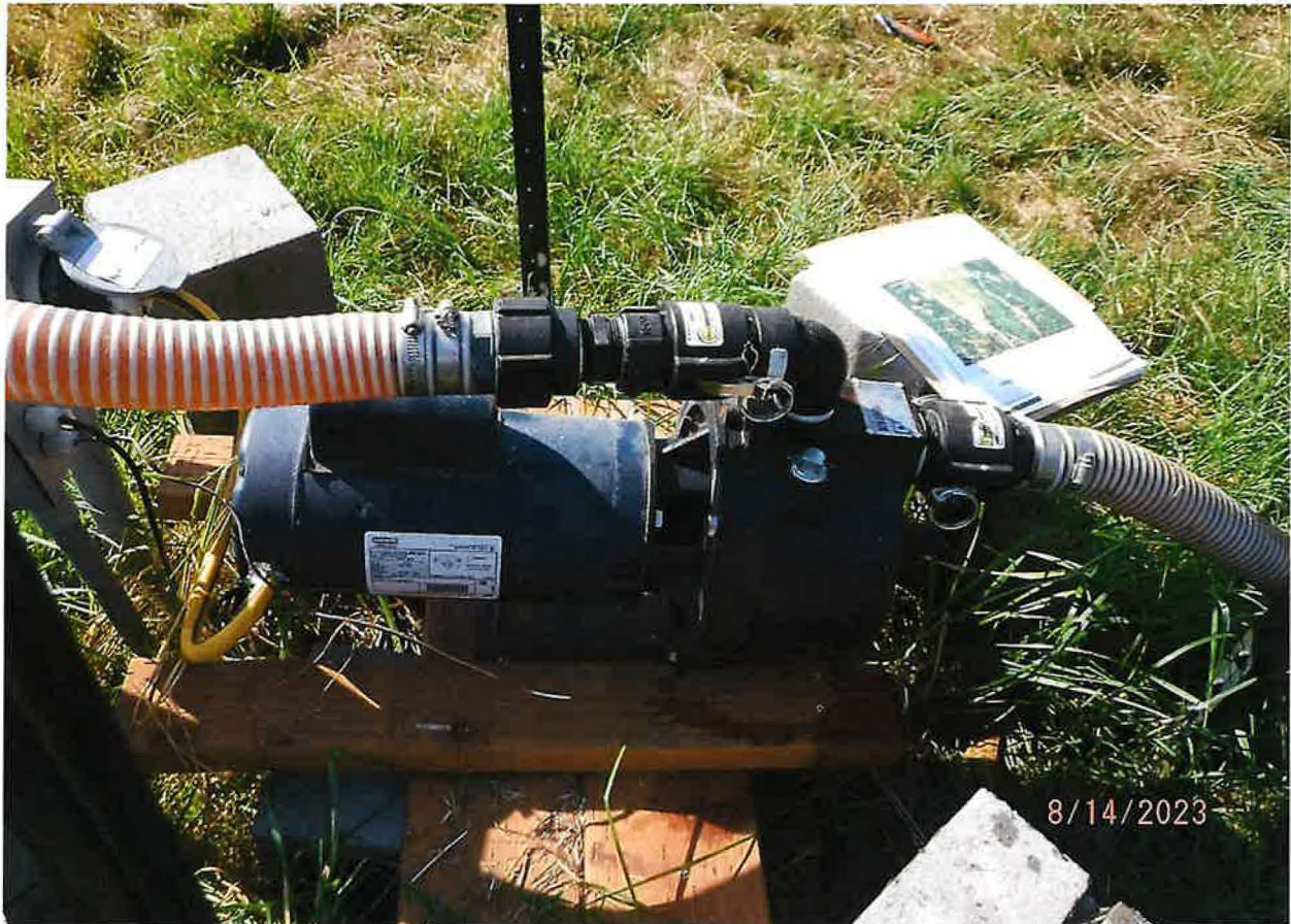
DIVERTING WORKS – 3 HP LEESON ELECTRIC TRANSFER PUMP
