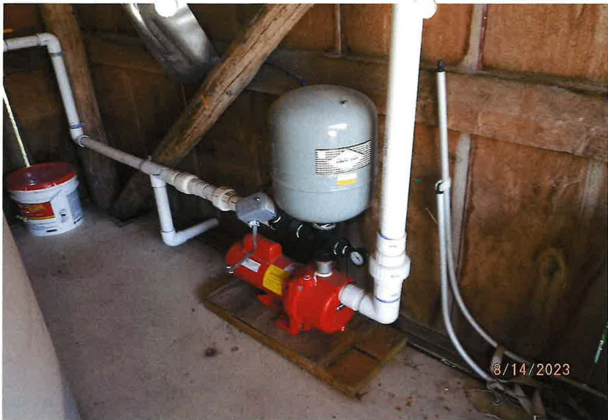
1 HP RED LINE TRANSFER PUMP WITH PRESSURE POT USED AS DISTRIBUTION PUMP FOR IRRIGATION SYSTEM
