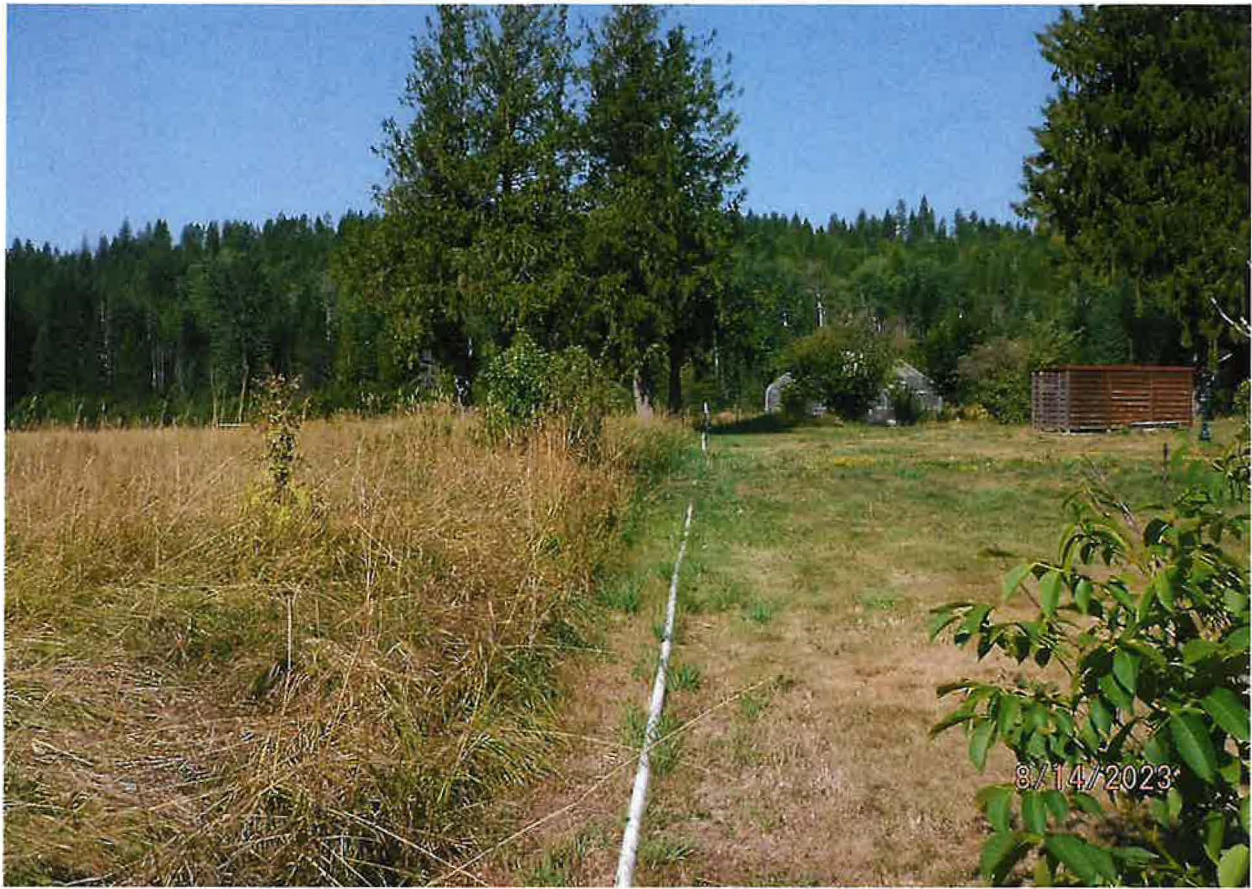
IRRIGATION POU – PIPELINE LOCATED IN FIELD SECTION SOUTHERN PORTION OF POU
