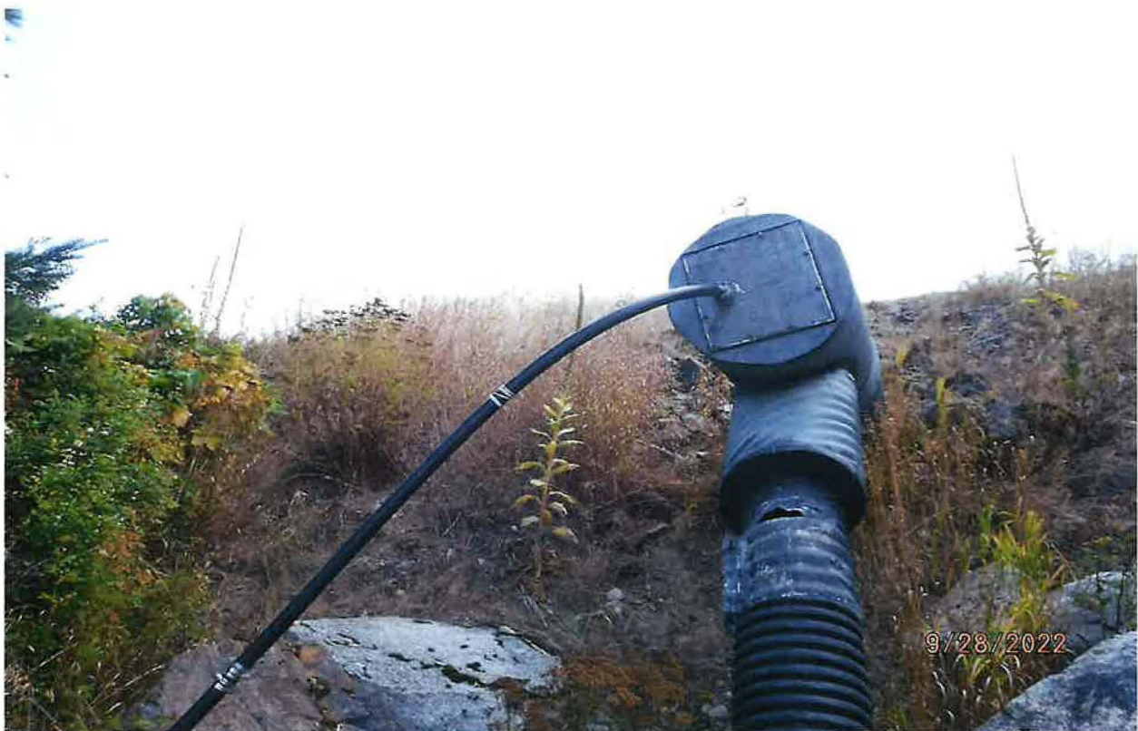
DIVERTING WORKS INCLUDES 1 ½ POLY LINE THAT ROUTES THROUGH CULVERT UNDER ROAD TO HOUSE SIDE IRRIGATION ACREAGE
