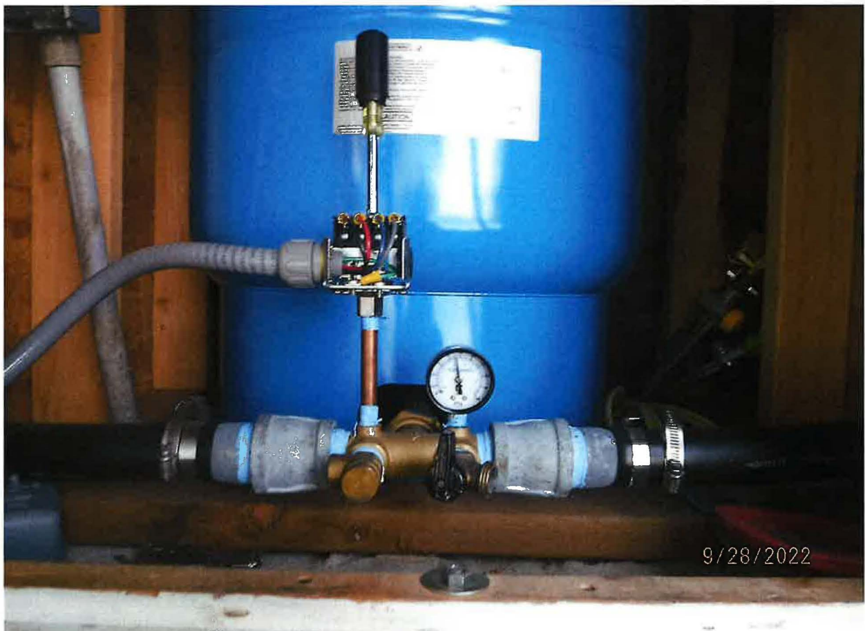
PUMP CONTROL HOUSE WITH PRESSURE TANK
