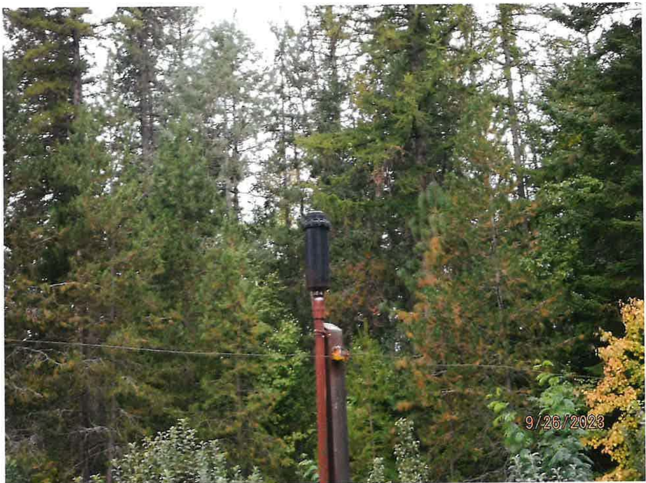
IRRIGATION POU – SPRINKLER RISER PIPE AND PRESSURIZED SPRINKLER RAINBIRD SPRAY NOZZLE
