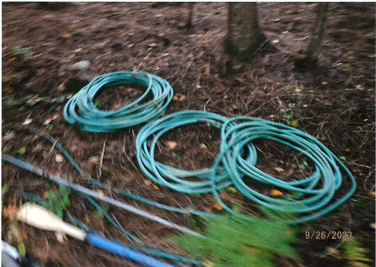
NUMEROUS HOSE TO SPRINKLERS USED IN SYSTEM
