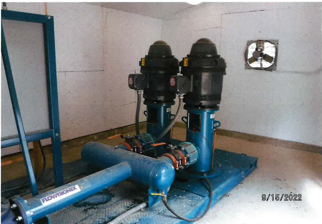
DIVERTING WORKS INCORPORATE 2EA 50 HP PUMPS
