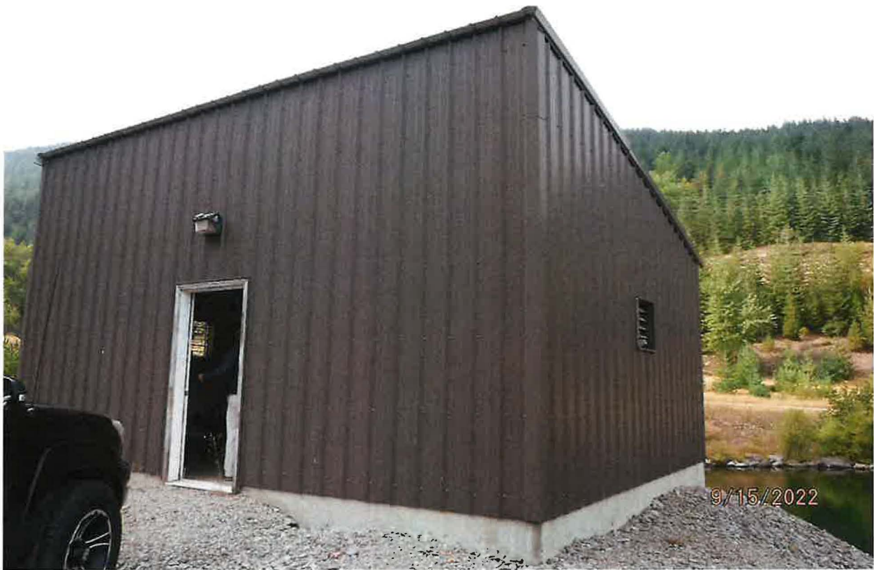
PUMP STATION LOCATED ON CREEK
