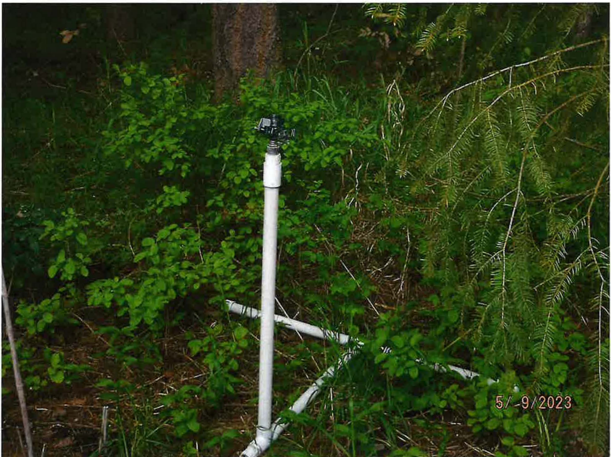
IRRIGATION SYSTEM COMPONENTS – MULTIPLE FROST-FREE HYDRANTS OF MAIN TRUNK LINE TO HOSE & RAINBIRD IMPACT SPRINKLERS
