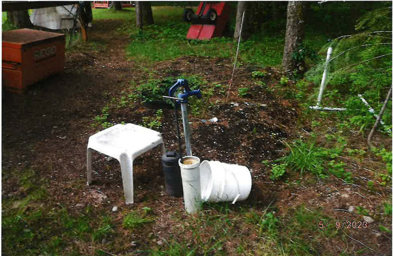
IRRIGATION SYSTEM COMPONENTS – MULTIPLE FROST-FREE HYDRANTS OF MAIN TRUNK LINE TO HOSE & RAINBIRD IMPACT SPRINKLERS
