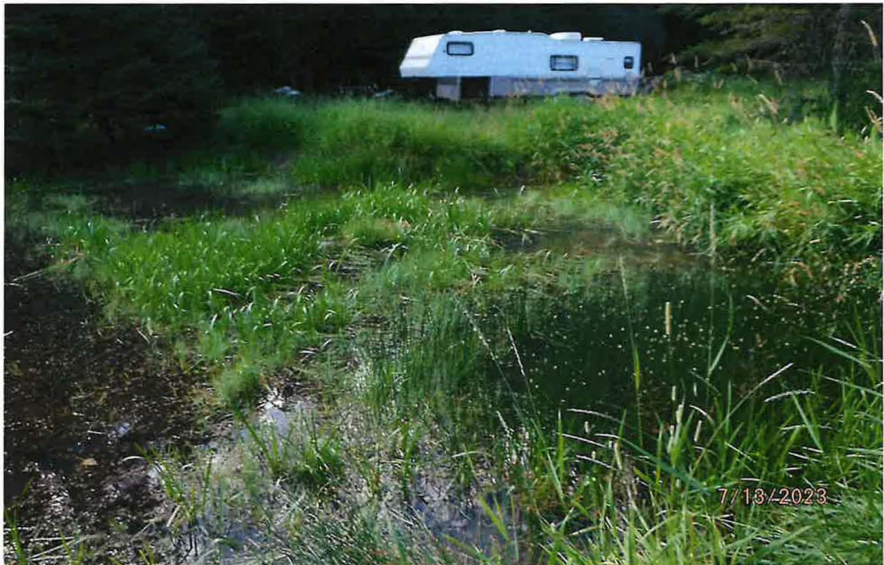
POD – EARTHEN POND DAM IMPOUNDS UNNAMED STREAM WATER
