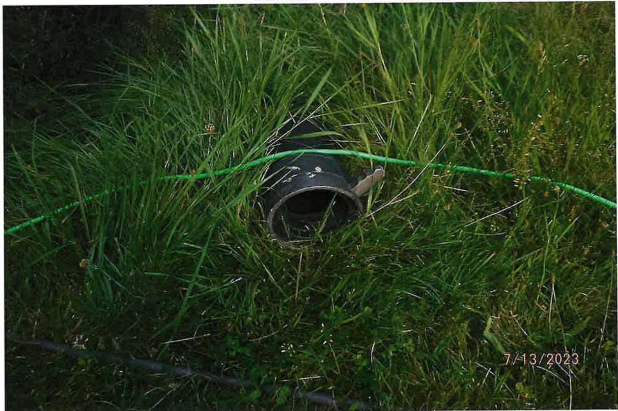
FIRE TRUCK HOSE ATTACHMENT FOR USE IN EVENT OF FIRE
