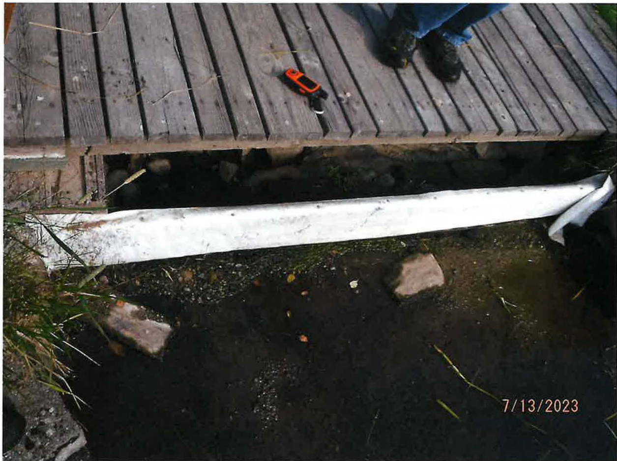
EARTHEN POND DAM WITH ROCKED FLOWTHROUGH CHANNEL WITH BOARD SEGMENTS USED TO RAISE/LOWER POND LEVEL
