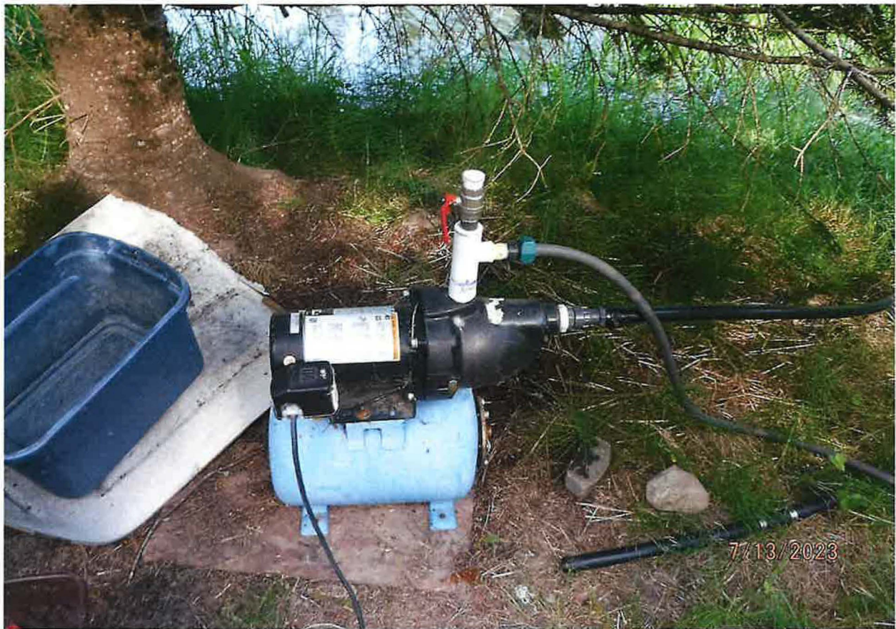
IRRIGATION FROM STORAGE SYSTEM – ½ HP FLOWTEC PUMP, 1 INCH POLY IN POND & 5/8 INCH GARDEN HOSE DISCHARGE
