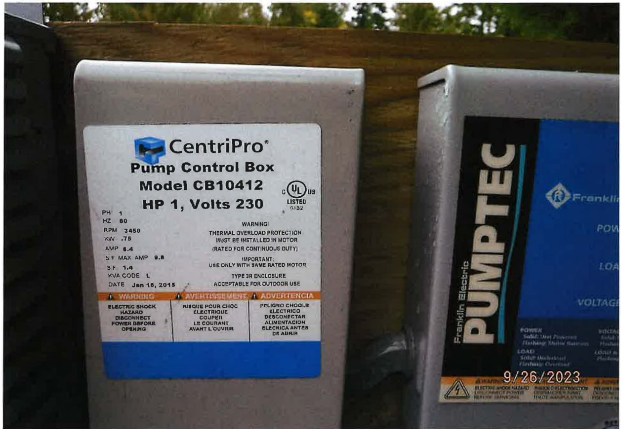
1 HP CENTRIPRO PUMP MOTOR RELAY CONTROL BOX
