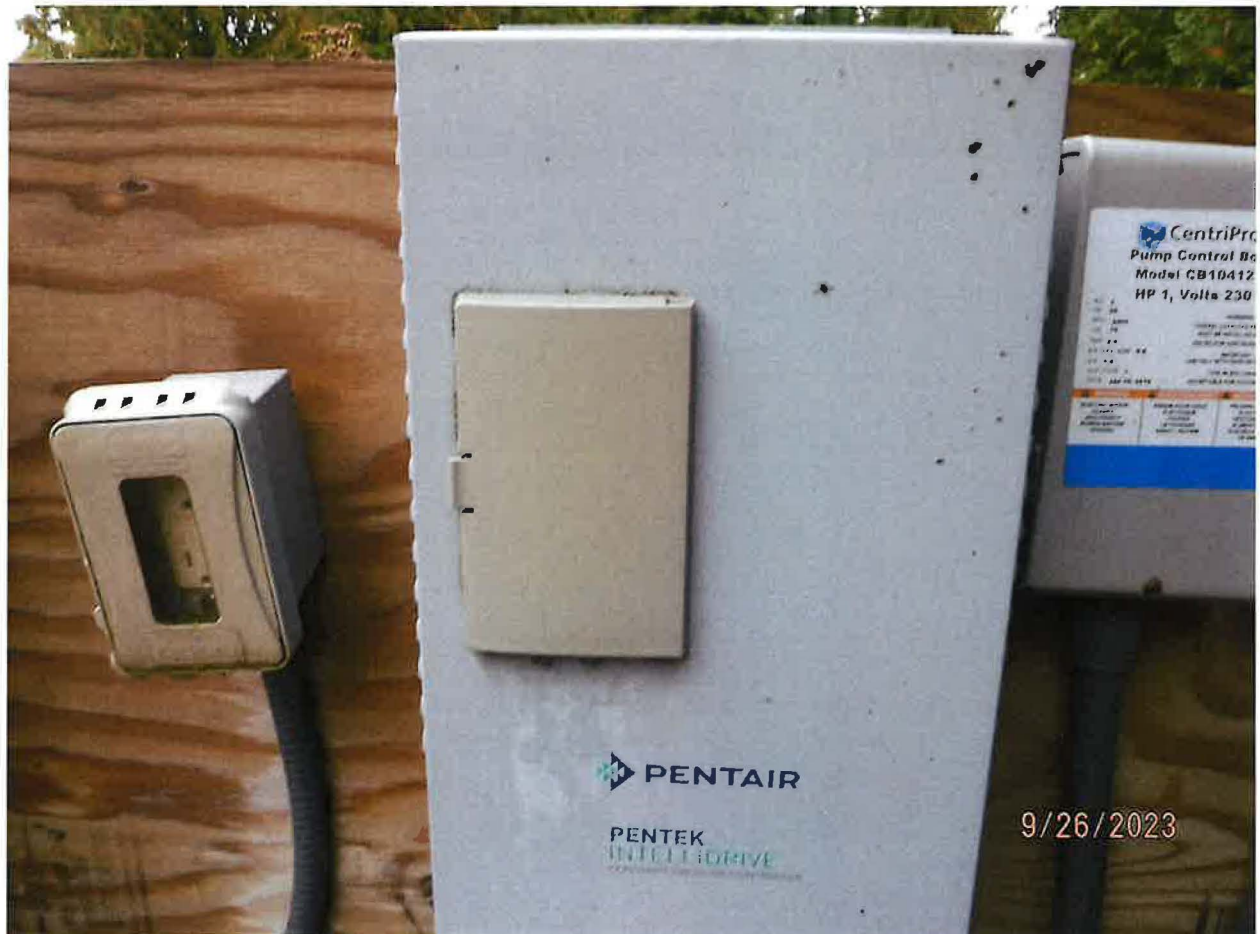
1 HP CENTRIPRO PUMP MOTOR RELAY CONTROL BOX
