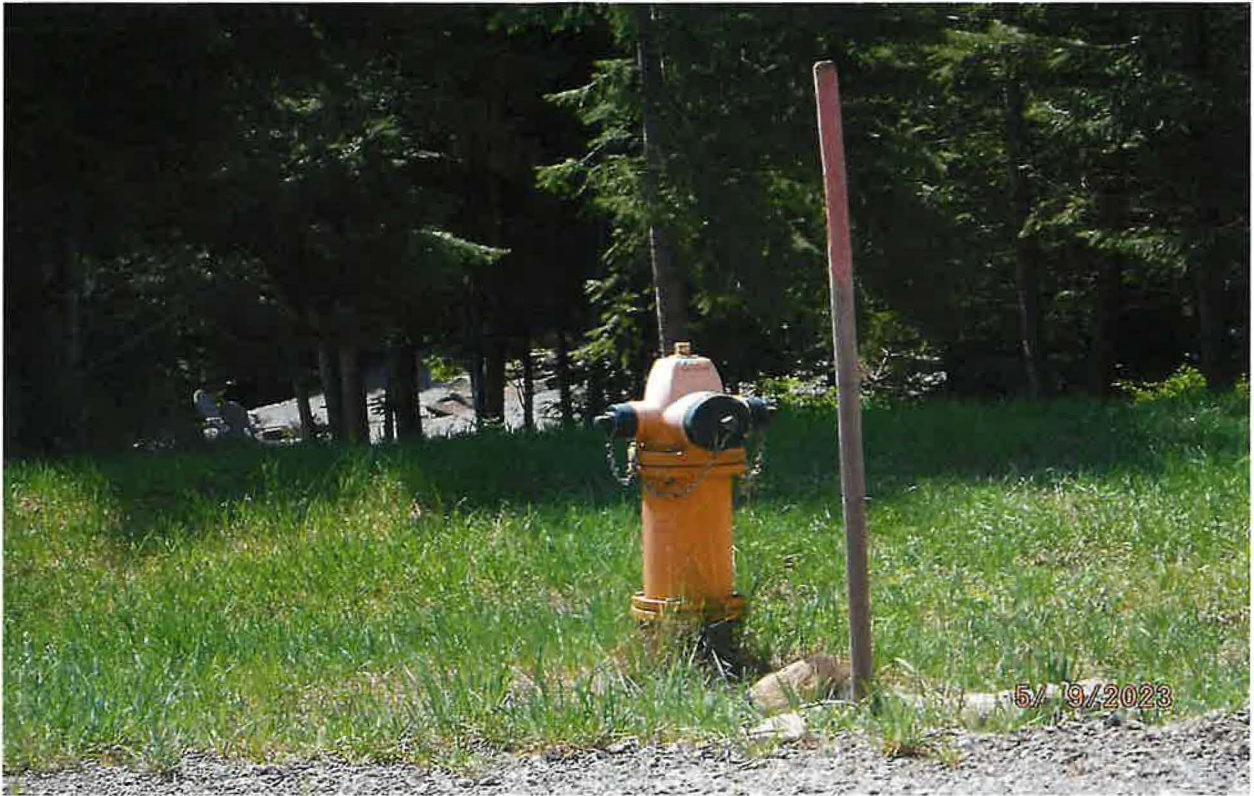
MUNICIPAL WATER SYSTEM INCORPORATES 11EA FIRE HYDRANTS LOCATED THROUGHOUT THE SUBDIVISION FOR FIRE SUPPRESSION REQUIREMENTS
