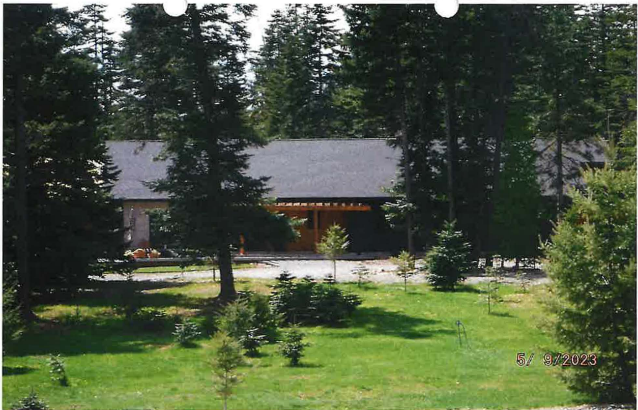
MUNICIPAL POU – EXAMPLE OF BUILT OUT LOT WITH RESIDENCE AND YARD IRRIGATION – NOTE FROST FREE HYDRANT LEFT OF DATE STAMP
