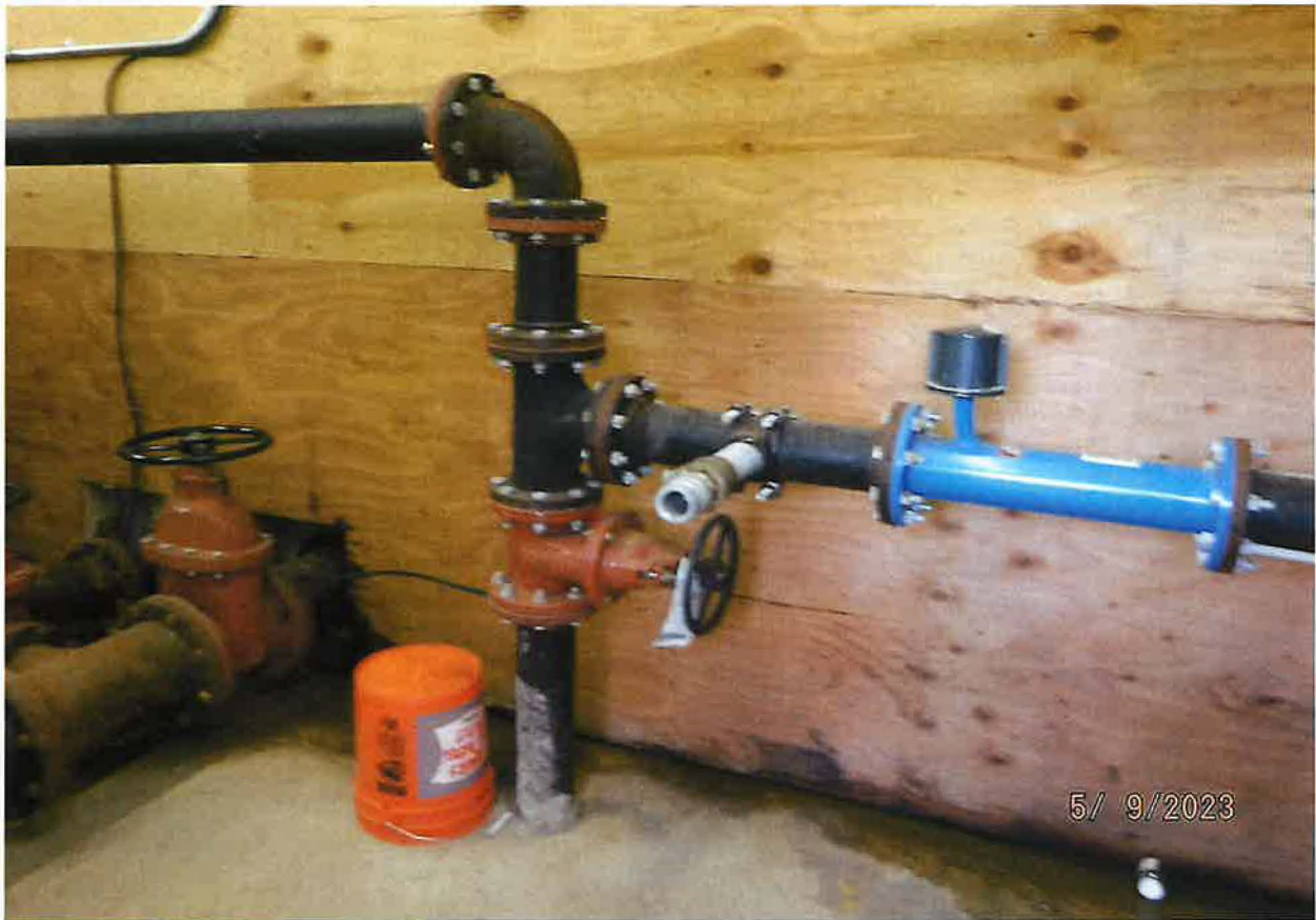
MCCROMETER FLOWMETER INSTALLED INLINE FROM MAIN SERVICE LINE FROM WELL, PRIOR TO RESERVOIR TANK AND WATER DISTRIBUTION VIA BOOSTER PUMPS
