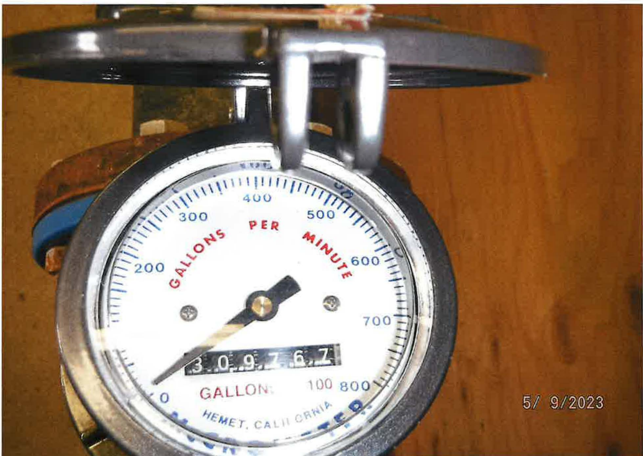
MCCROMETER FLOWMETER INSTALLED INLINE FROM MAIN SERVICE LINE FROM WELL, PRIOR TO RESERVOIR TANK AND WATER DISTRIBUTION VIA BOOSTER PUMPS
