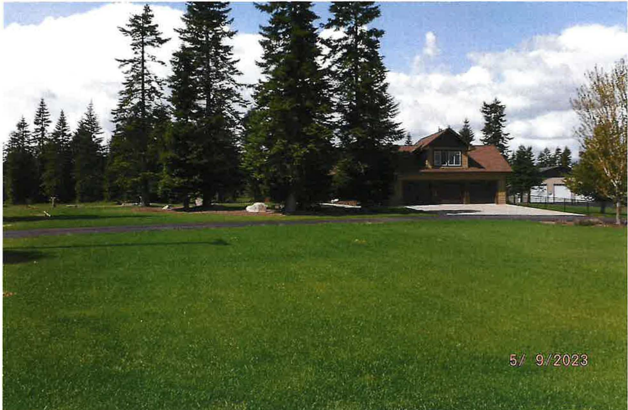
MUNICIPAL POU – 1 OF 19 BUILT OUT RESIDENCES SERVICE CONNECTED; LARGEST LAWN IRRIGATION OF ALL 22 PARCELS ON SYSTEM – RP0K0140020140
