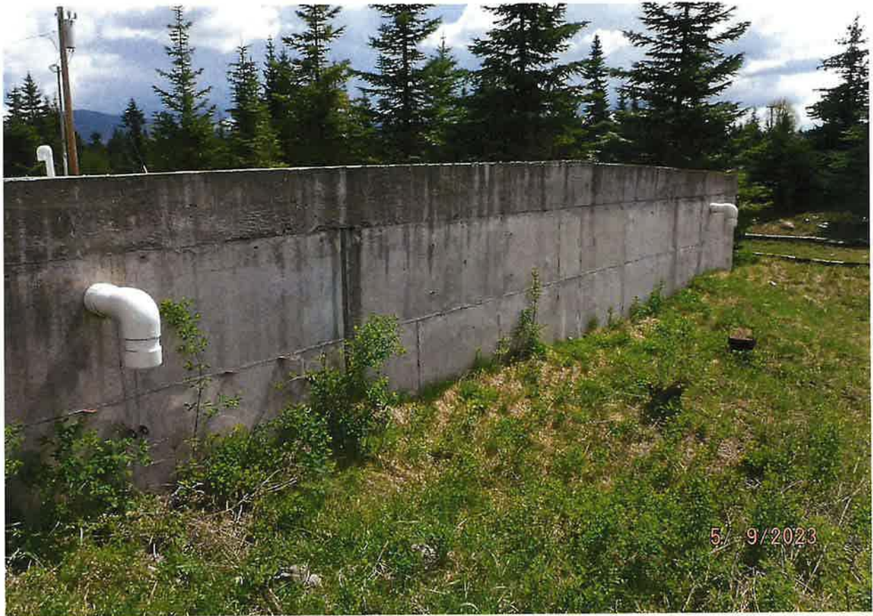
90K STORAGE RESERVOIR WITH WATER LINE SHUTOFF VALVES
