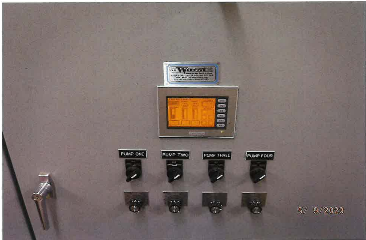
WATER SYSTEM INCORPORATES A DIGITAL SCADA MANAGEMENT SYSTEM
