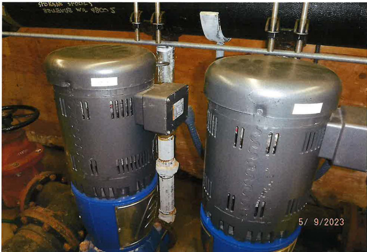
WATER CONVEYANCE SYSTEM - 4EA GOULDS 10 HP BOOSTER PUMPS USED FOR DISTRIBUTION FROM STORAGE RESERVOIR TO SERVICE CONNECTIONS.
