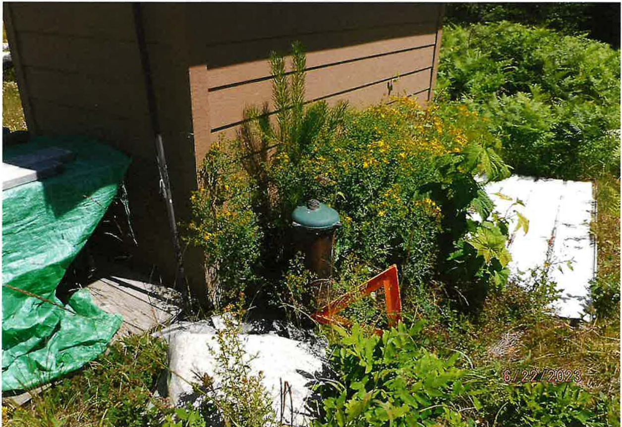
POD – GROUDNWATER WELL D0076054
