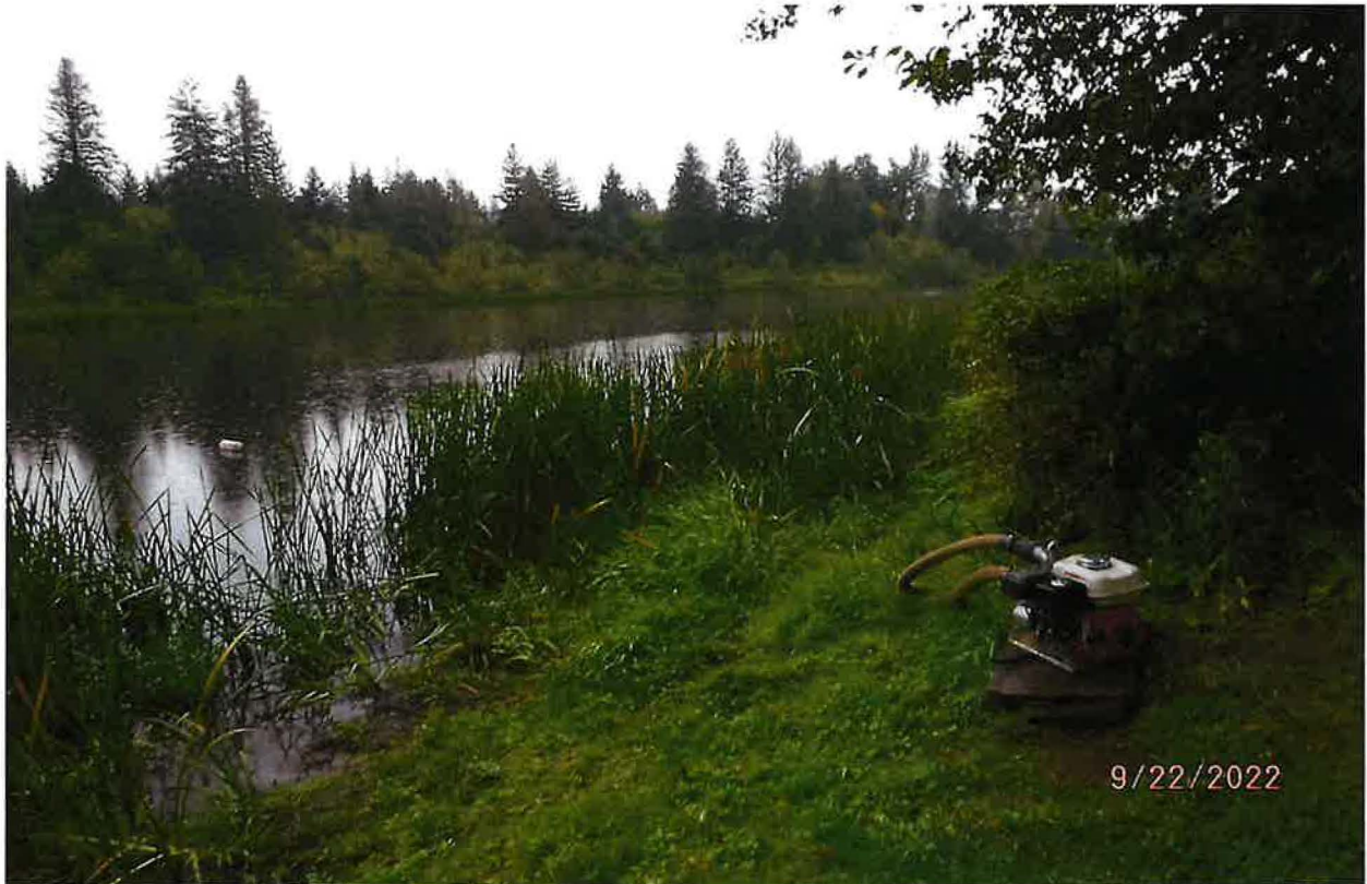
POD – WATER TRANSFER PUMP
