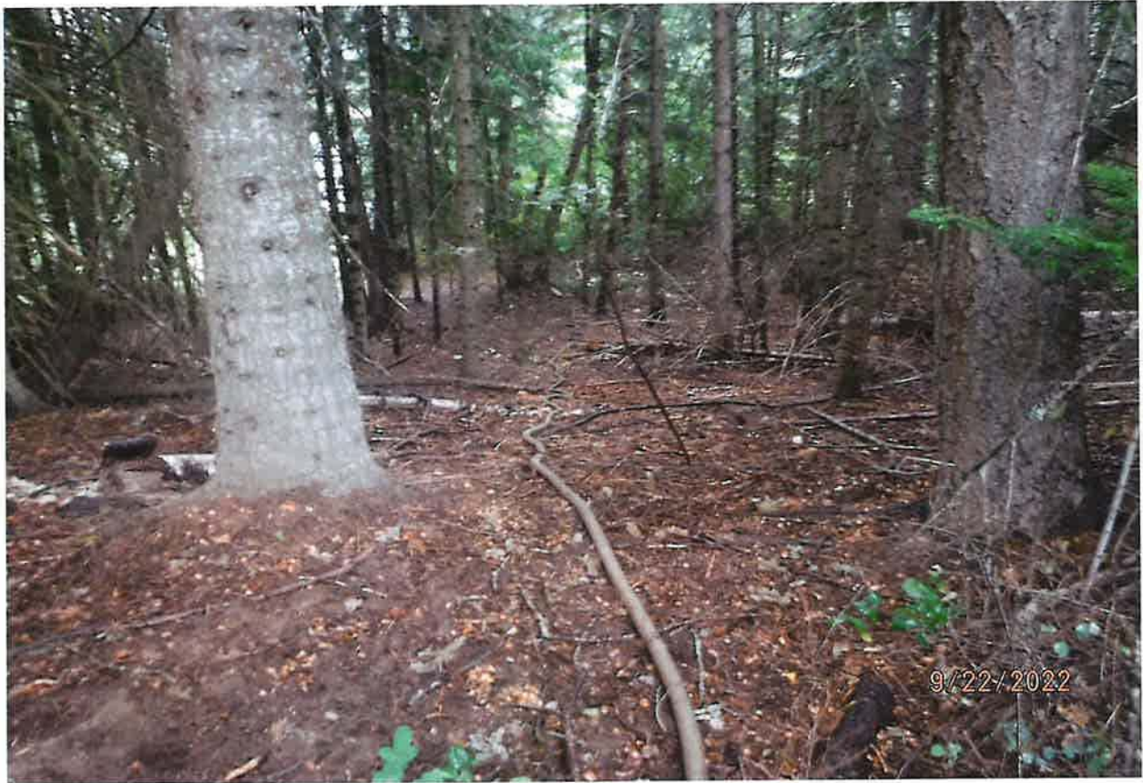
2 INCH DISCHARGE FROM PUMP TO 1.5 INCH FLEX FIRE HOSE ROUTING TO IRRIGATION POU
