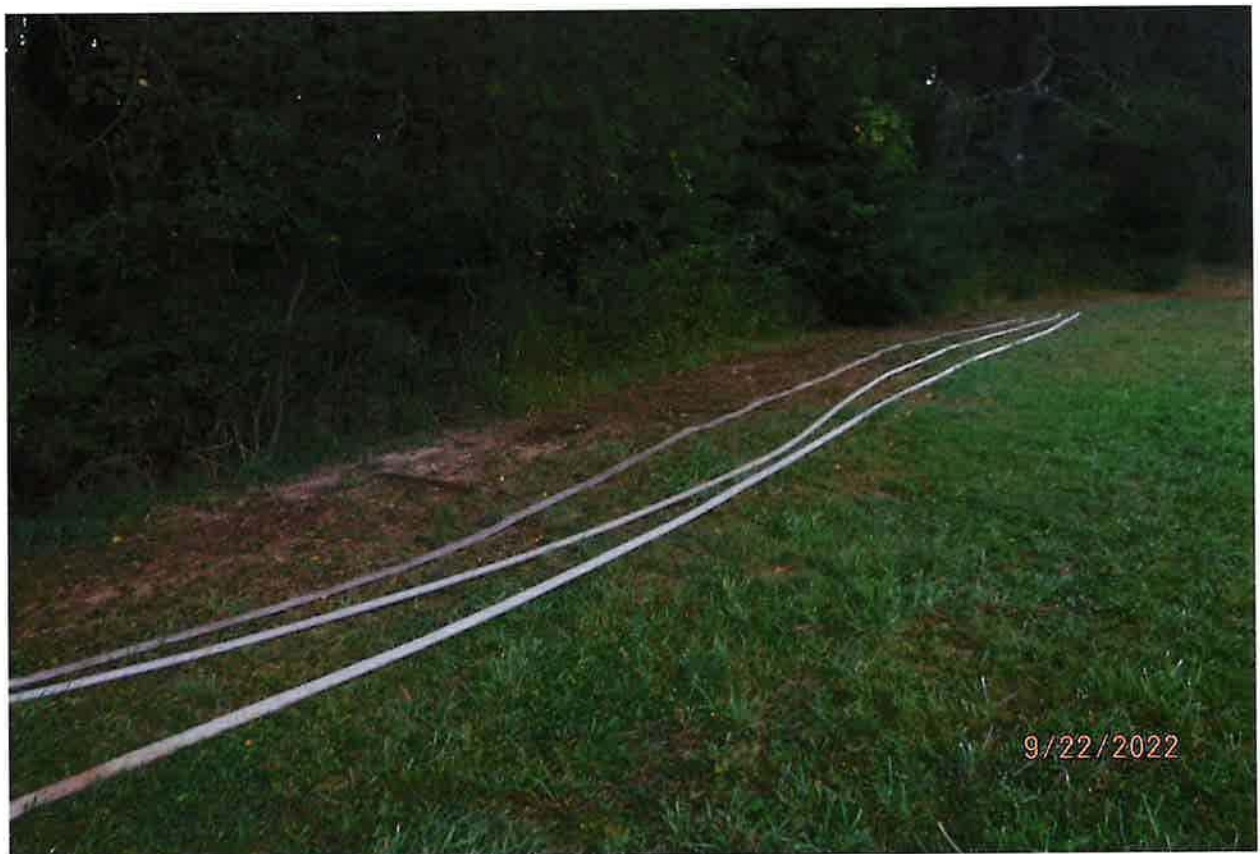
2 INCH DISCHARGE FROM PUMP TO 1.5 INCH FLEX FIRE HOSE ROUTING TO IRRIGATION POU
