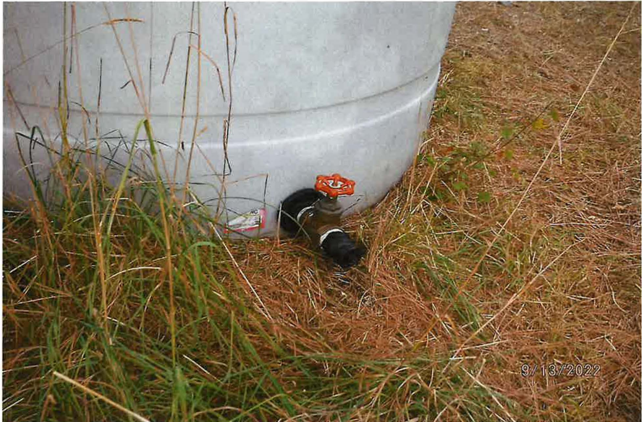
HOSE CONNECTION FROM STORAGE TANKS
