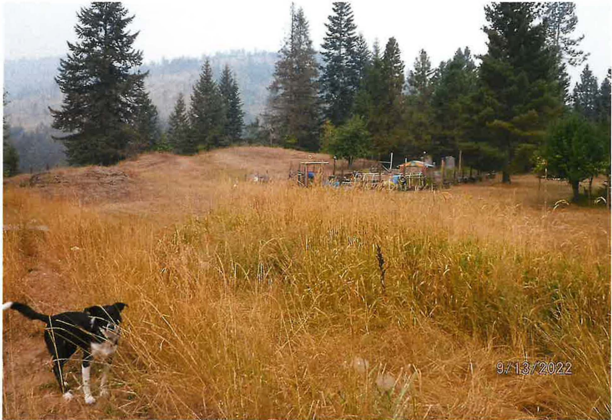
VIEW FROM POD ALONG CREEK TO STORAG TANKS; PUMP FROM POD TO STORAGE, GRAVITY FLOW FOR WATER USE FROM STORAGE TANKS.
