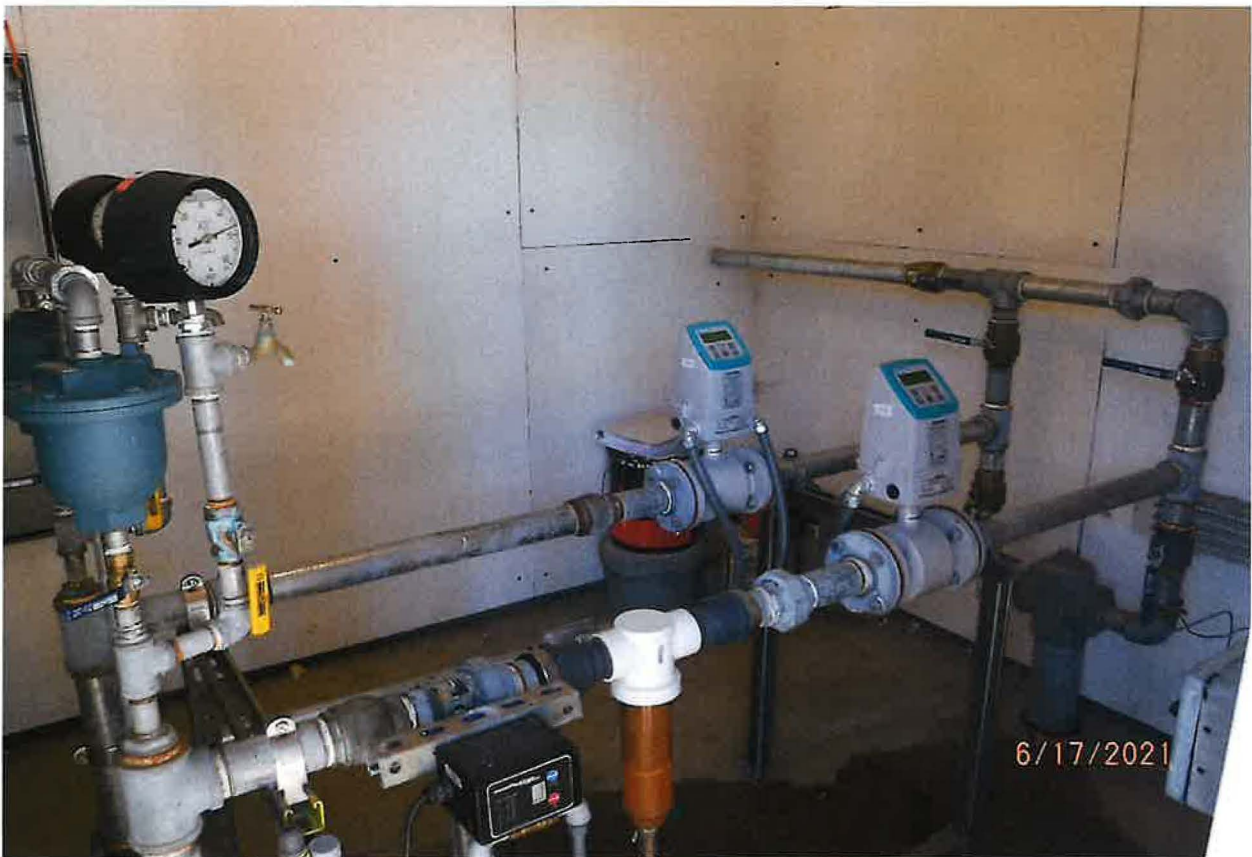
WELL No.6 & No. 7 PUMP STATION WITH DIVERTING WORKS
