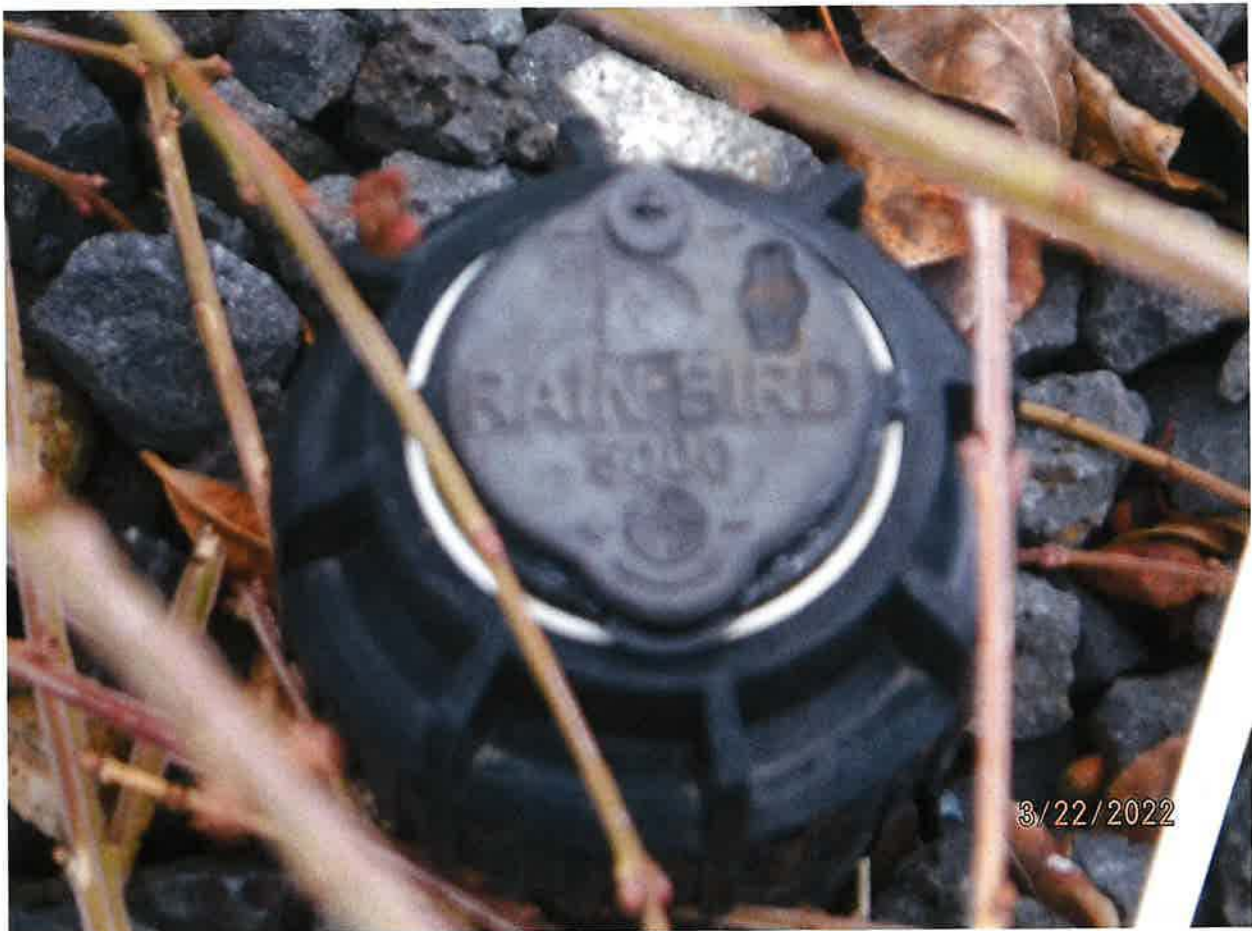
IRRIGATION POU – PRESSURIZED SPRINKLER SYSTEM
