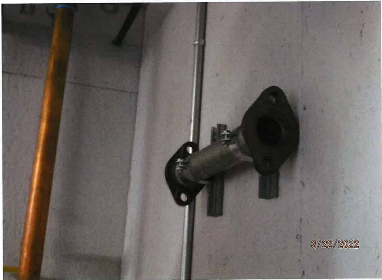
DOMESTIC USE INTERCONNECT W/COUPLER PIPE
