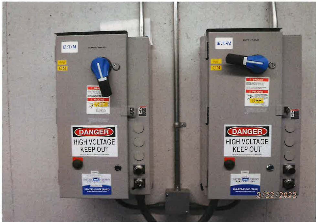
2EA 45 GPM FRANKLIN 7.5 HP PUMPS INSTALLED
