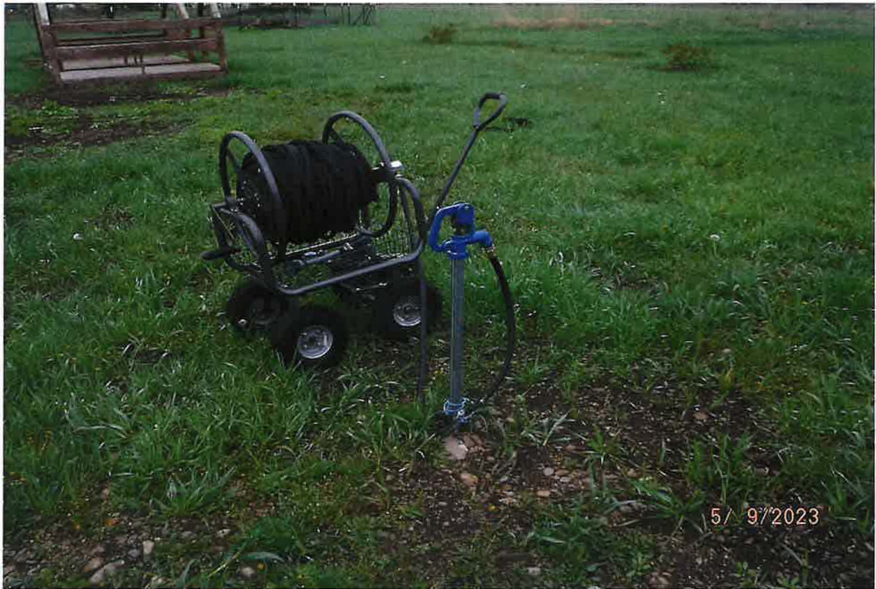
IRRIGATION POU – FROST FREE HYDRANT TO HOSE & SPRINKLER FOR FENCED GARDEN AREA
