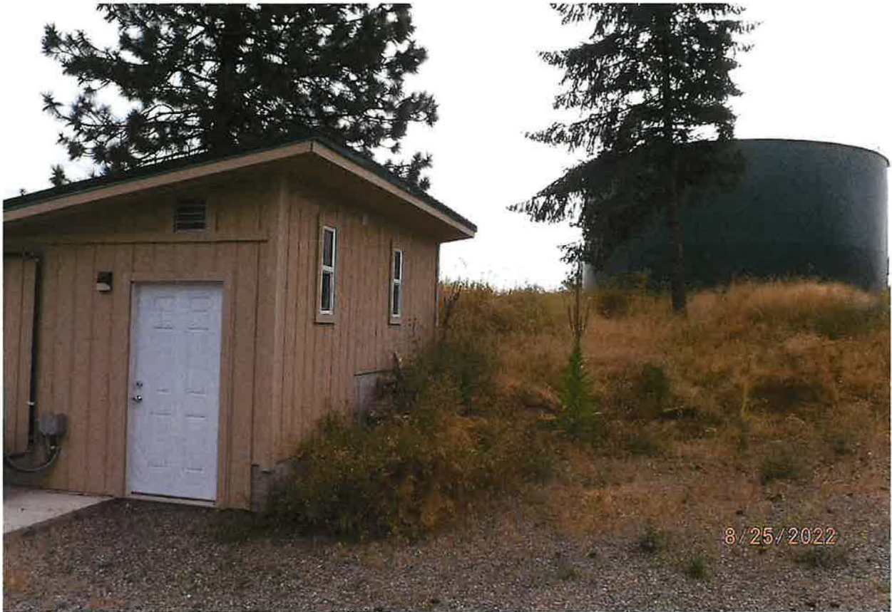
100,000-GAL STORAGE RESERVOIR
