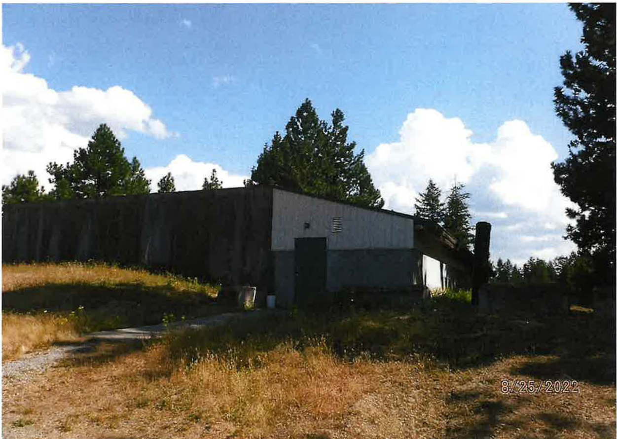
SLOW SAND FILTRATION SYSTEM BUILDING.
