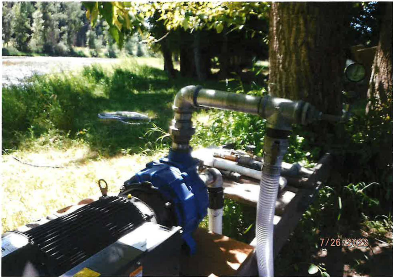
IRRIGATION DIVERSION WORKS – 10 HP CENTREFUGAL PUMP
