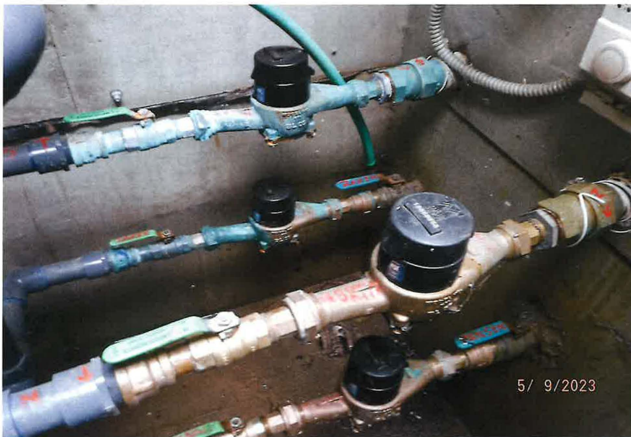
4EA FLOWMETERS INSTALLED ON DISTRIBUTION SERVICE LINE TO 4 HOMES (INLINE AFTER PRESSURE TANK)
