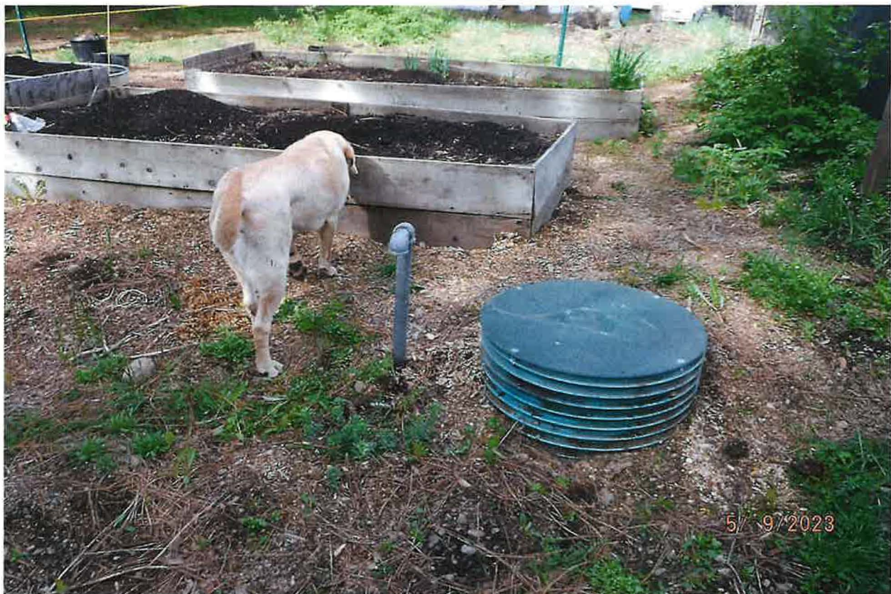
2,500 GAL COMMUNITY STORAGE RESERVOIR (LOCATED OPPOSITE SIDE OF FENCE FROM WELL
