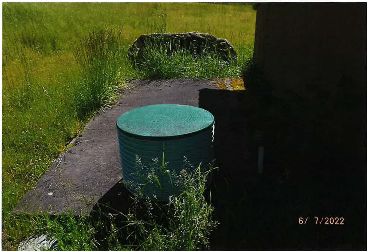
VAULTED 1,500 GAL CISTERN – LID LOCTED OUTSIDE PUMP HOUSE
