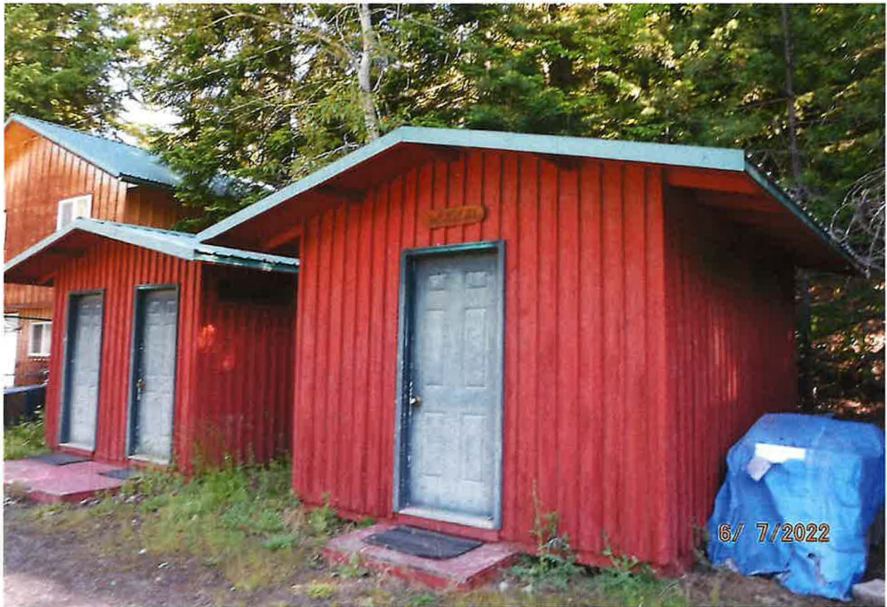
COMMERCIAL POU – OFFIC BUILDING (L/H), BATHROOMS (MIDDLE), & LAUNDARY ROOM (R/H)
