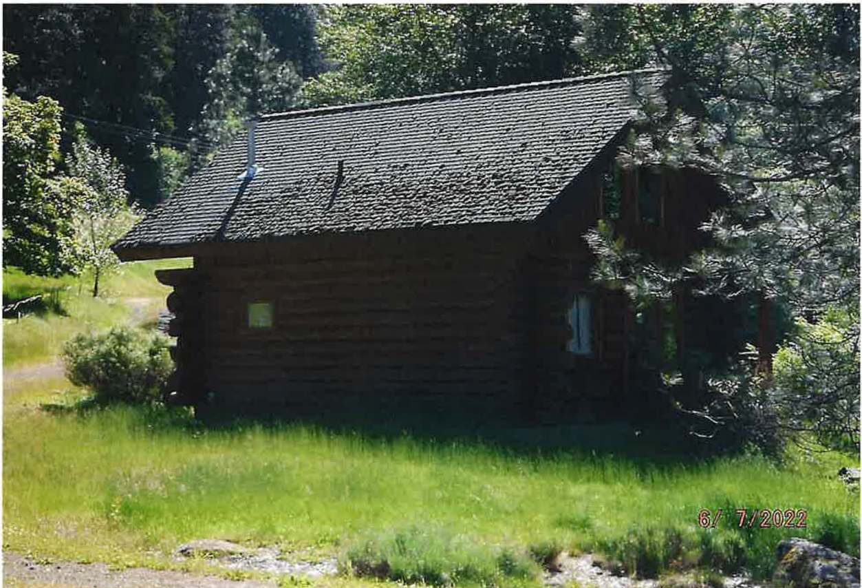
COMMERCIAL POU – 1 OUT OF 4 SINGLE UNIT RENTAL CABINS
