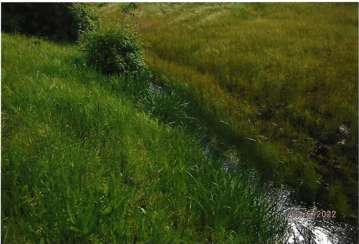
OVERFLOW CHANNEL ALLOWS WATER TO CONTINUE DOWNSTREAM TO LOWER POND
