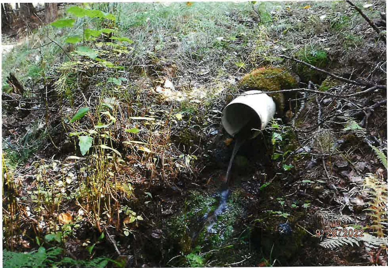
LOWER POND OVERFLOW DISCHARGE PIPE ROUTES DOWN HILL TO PRIEST RIVER
