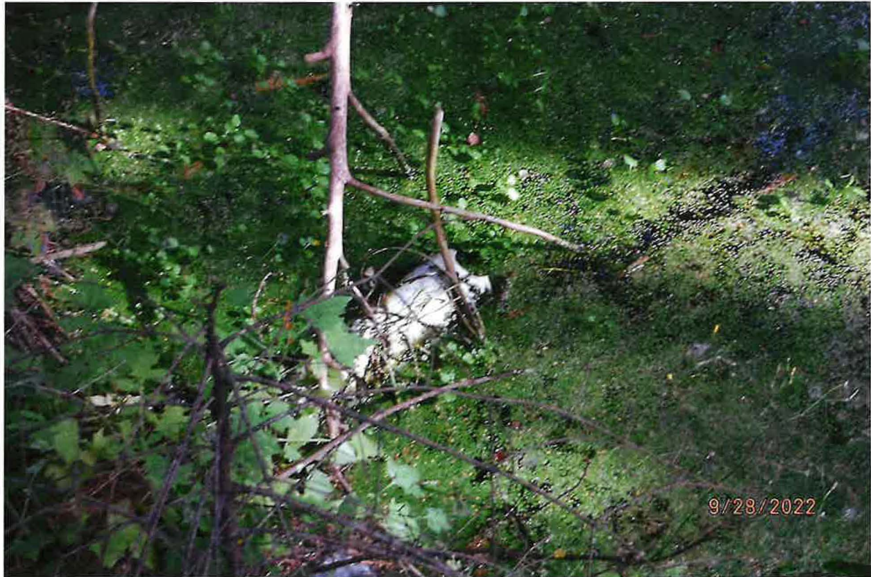
UPPER POND POD – EARTHEN DAM WITH 4 INCH PVC PIPE OVERFLOW INSTALLED
