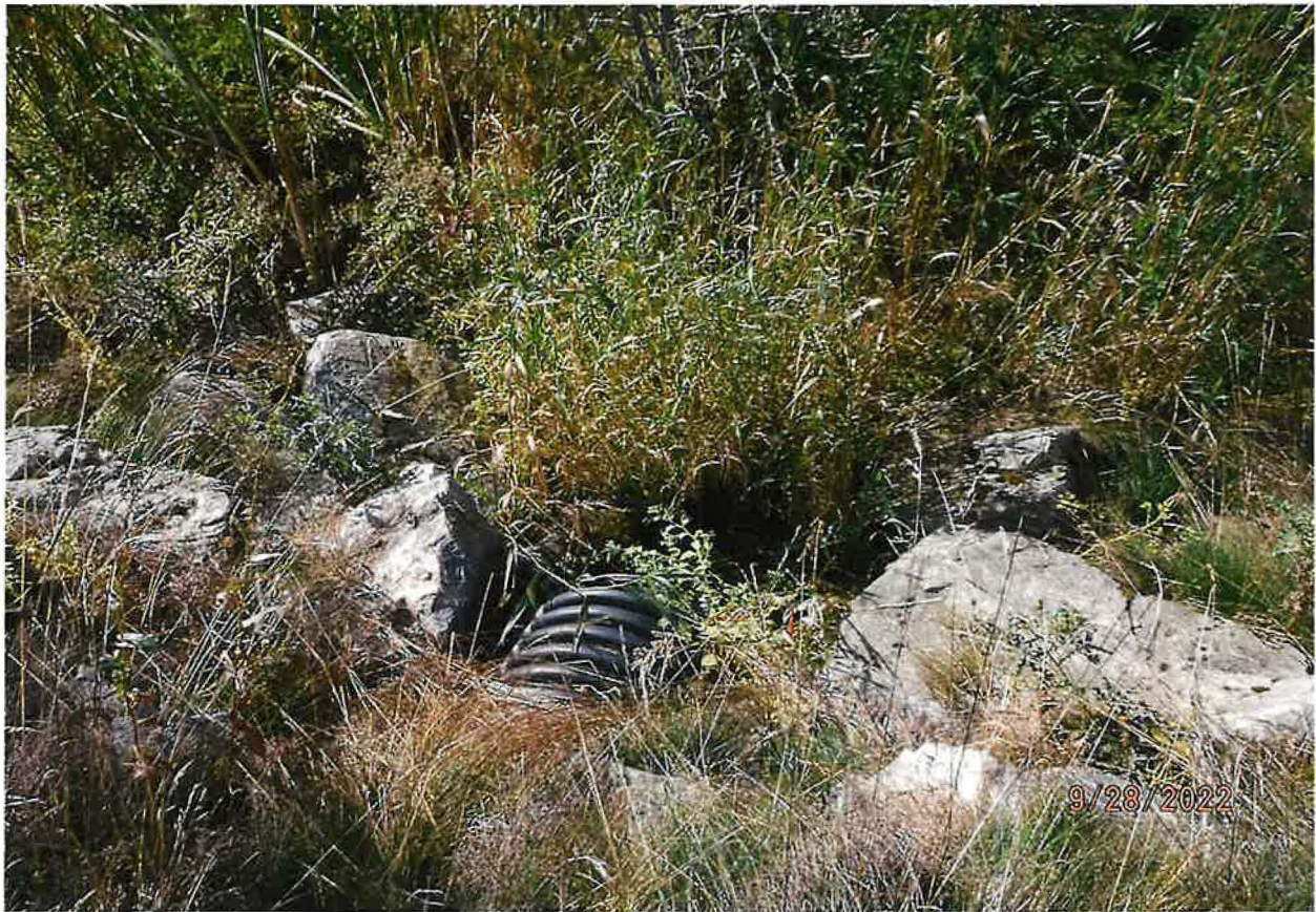
OVERFLOW WATER DISCHARGES DOWN GRADE TO PRIEST RIVER
