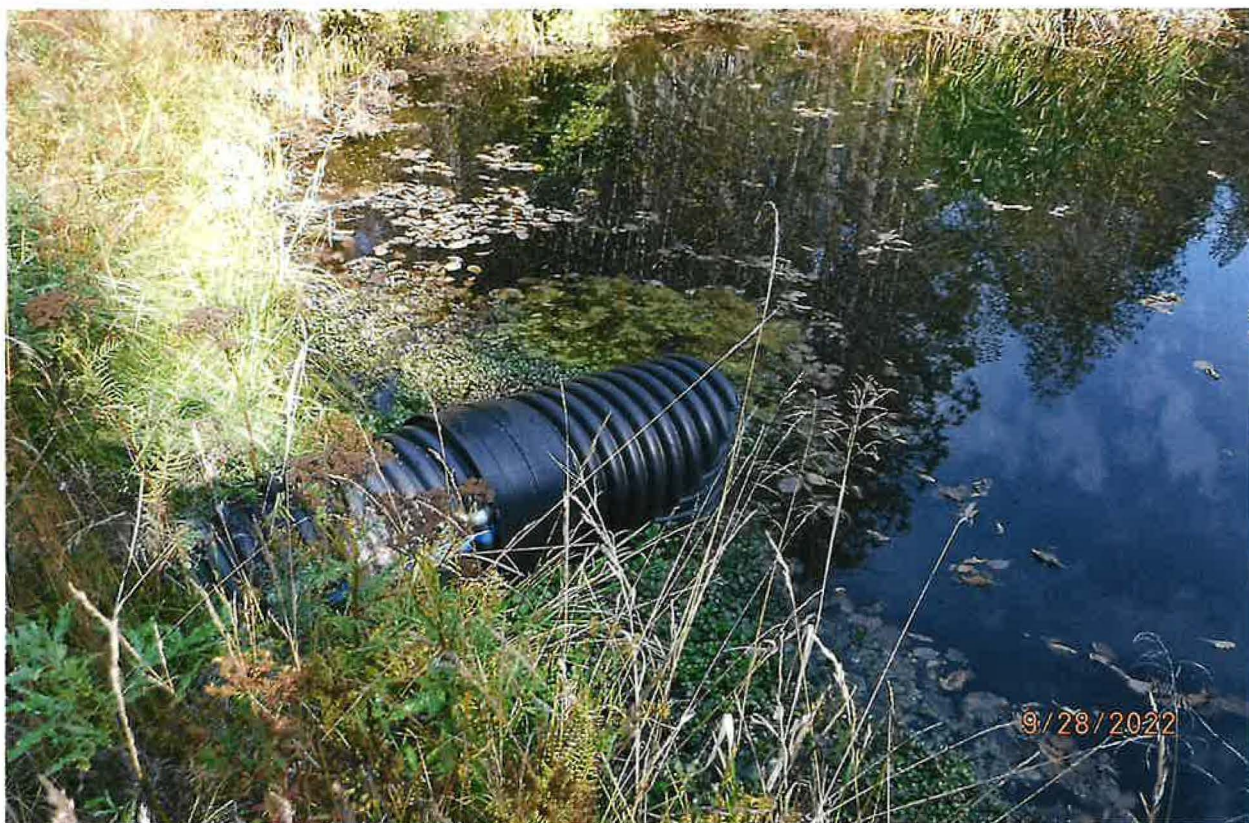
POD – POND EARTHEN DAM WITH STORM DRAIN PIPE OVERFLOW DEVICE INSTALLED
