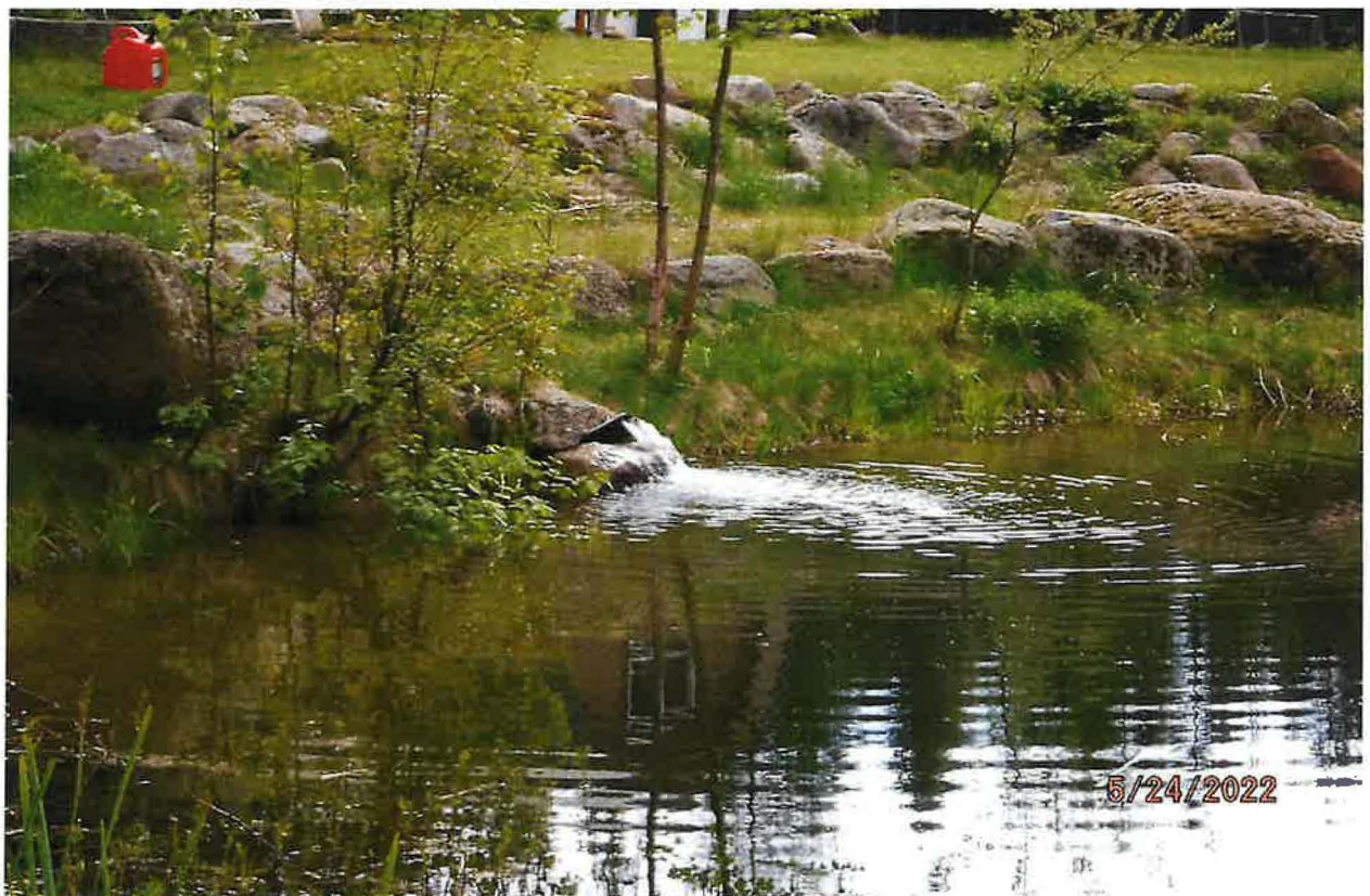
WATER INFLOW TO STORAGE POND
