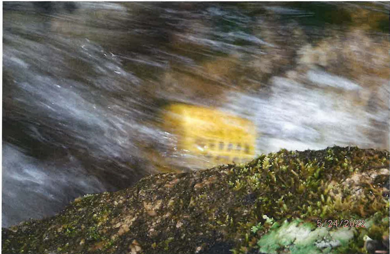
SCREENED INTAKE PIPE
