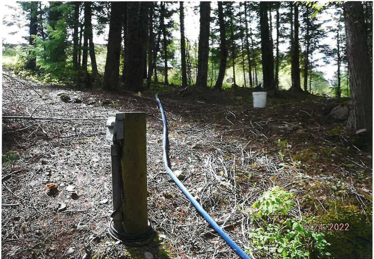
BLUE FLEX FIRE HOSE FROM POD TO STORAGE POND POU
