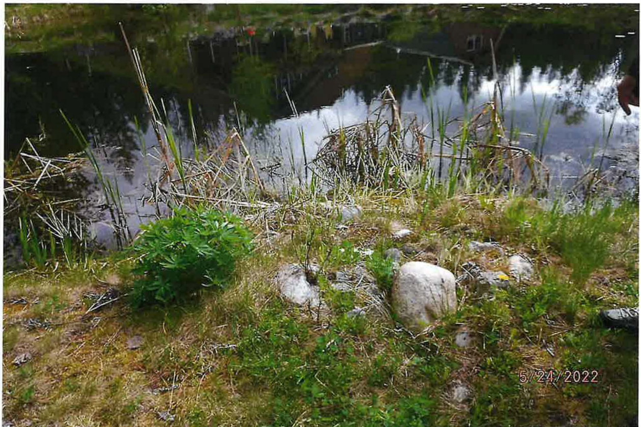
ROCK COVERED OVERFLOW DISCHARGE PIPE
