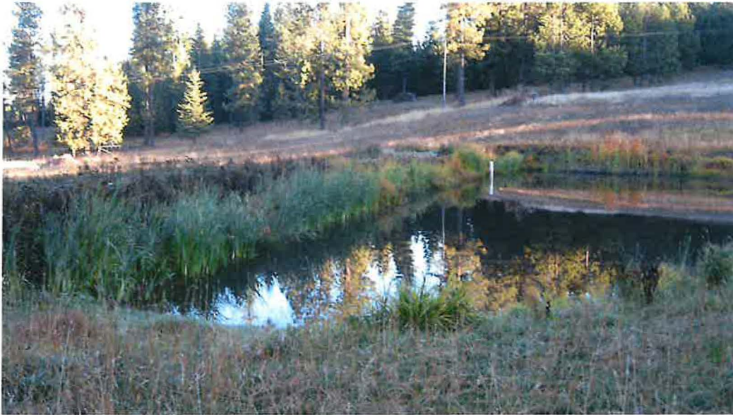
POD – EARTHEN DAM FOR UNNAMED STREAM
