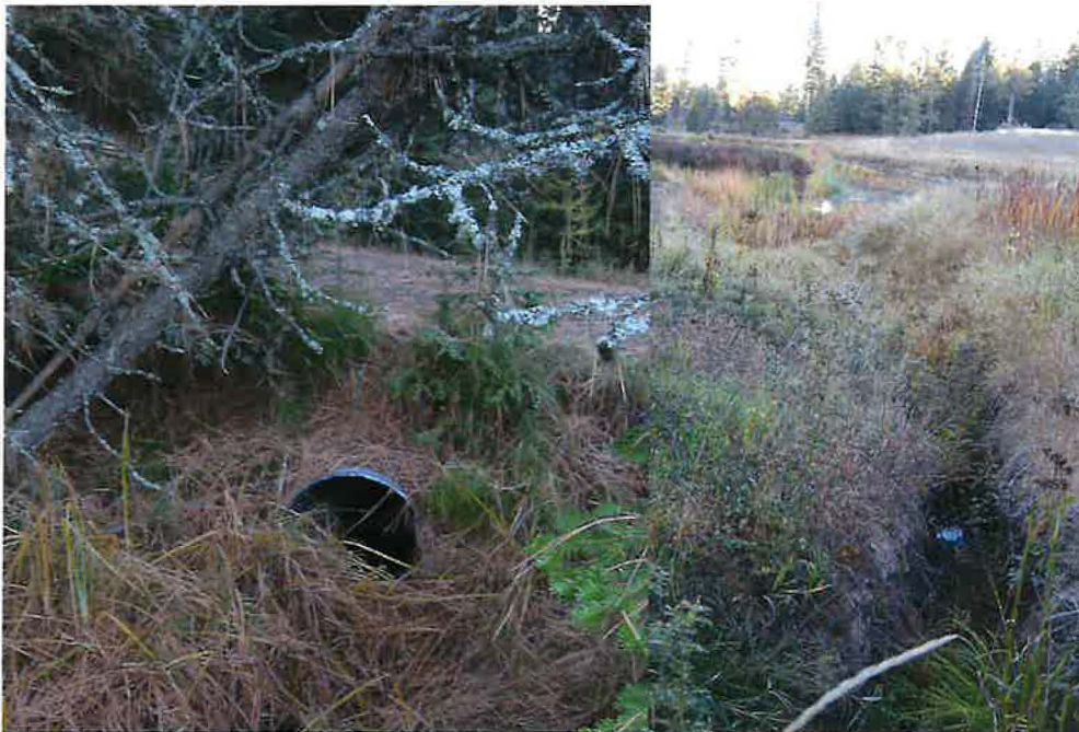
SOURCE – UNNAMED STREAM, CULVERT AND CHANNEL LEADING TO POND
