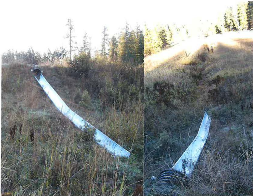
OUTFLOW CHANNEL FROM EARTHEN DAM
