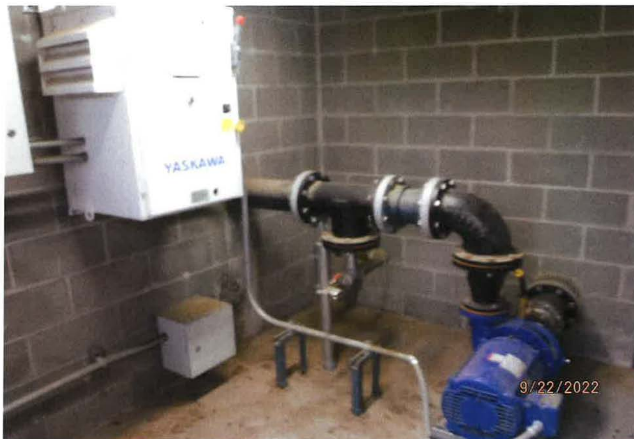
DIVERTING WORKS – 3 PHASE 15 HP CENTRIFUGAL PUMP MODEL HA72
