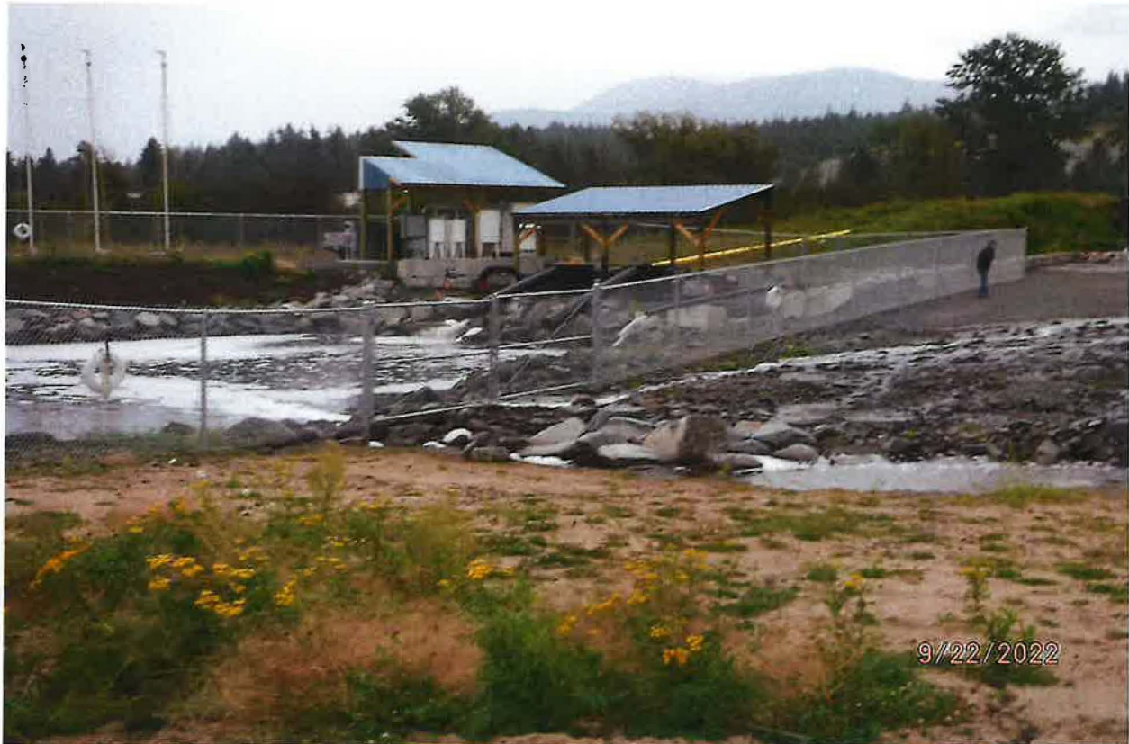
RECIRCULATION POND RECYCLES INDUSTRIAL LOG WATERING OVERFLOW CAPTURE
