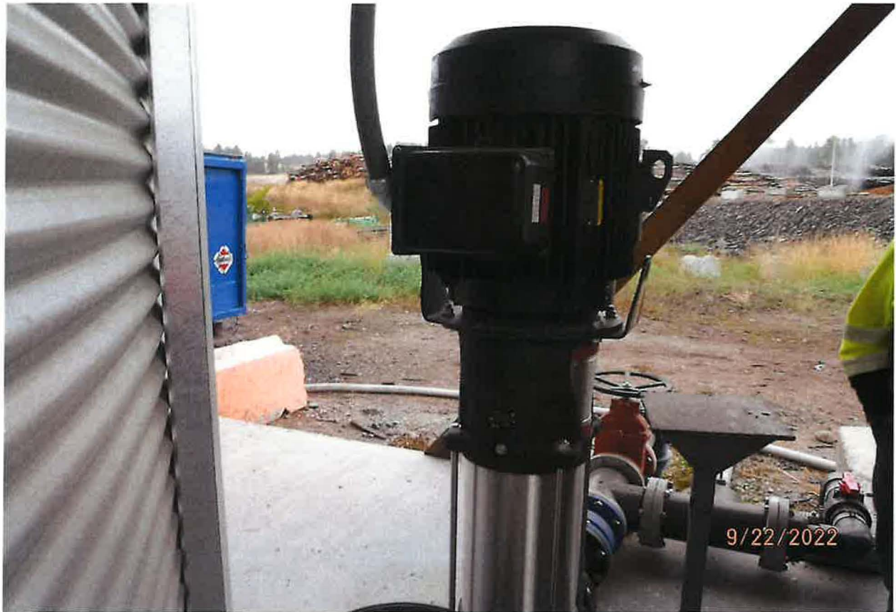
BALDOR 75 HP TRANSFER PUMP FROM STORAGE TANK TO INDUSTRIAL & FIRE PROTECTION USES
