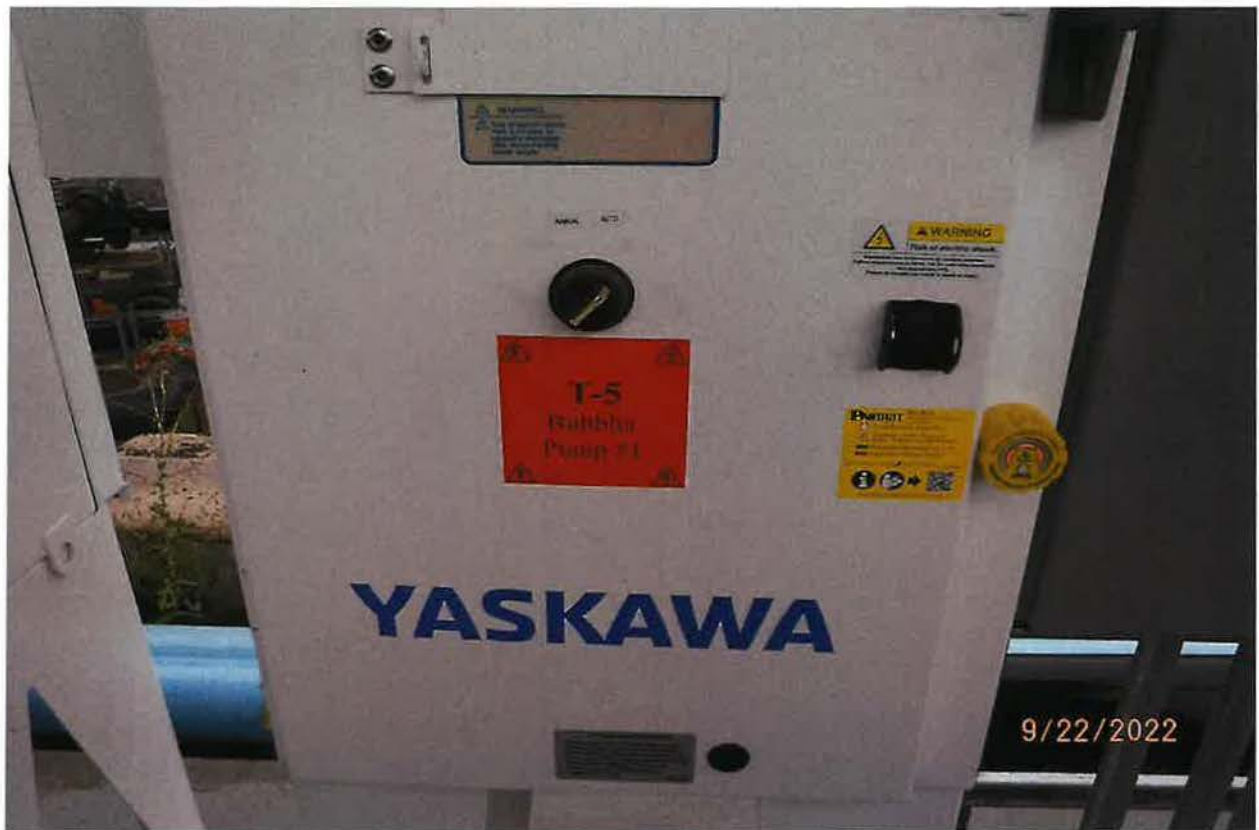
BUBBLER 7.5 HP PUMP FOR SYSTEM # 1 CONTROL PANEL
