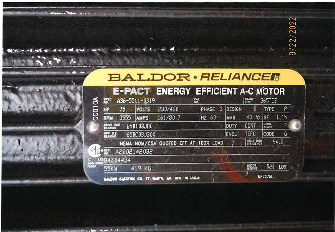
BALDOR 75 HP TRANSFER PUMP FROM STORAGE TANK TO INDUSTRIAL & FIRE PROTECTION USES
