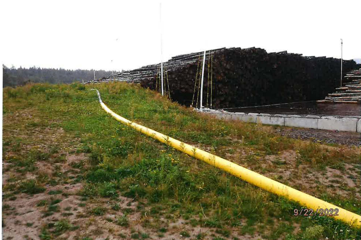
RECLAIMED WATER FROM RECIRCULATION POND - MAIN WATER LINE FOR LOG WATERING
