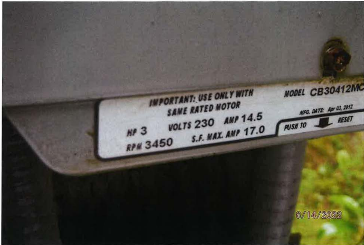
3 HP CENTRIPRO PUMP MOTOR INSTALLED IN WELL
