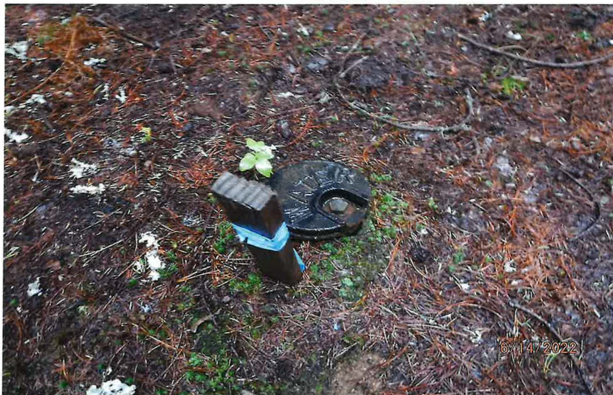
DOMESTIC POU – STUB-IN – LOT 3 PHASE II REPLAT, ELKINS REEDER ACRES PHASE 2 SUB. – RP054070010030A
