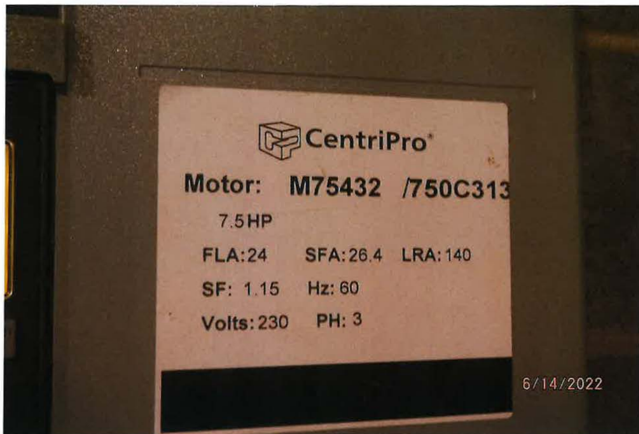
7.5 HP CENTRIPRO PUMP MOTOR INSTALLED ON GOULDS 65GS75 PUMP
