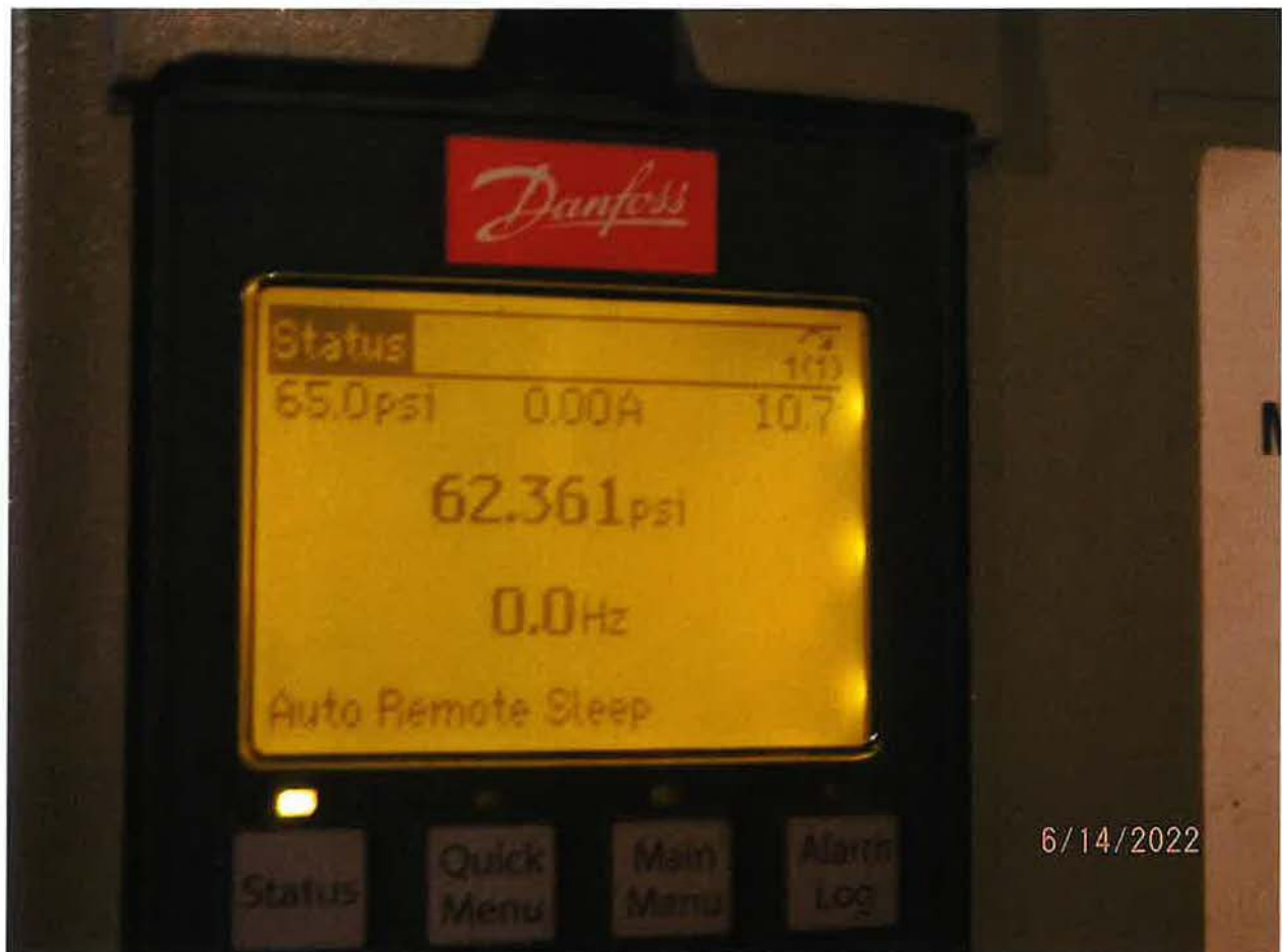
60-65 PSI OPERATING PRESSURE OBSERVED AT TIME OF EXAM
