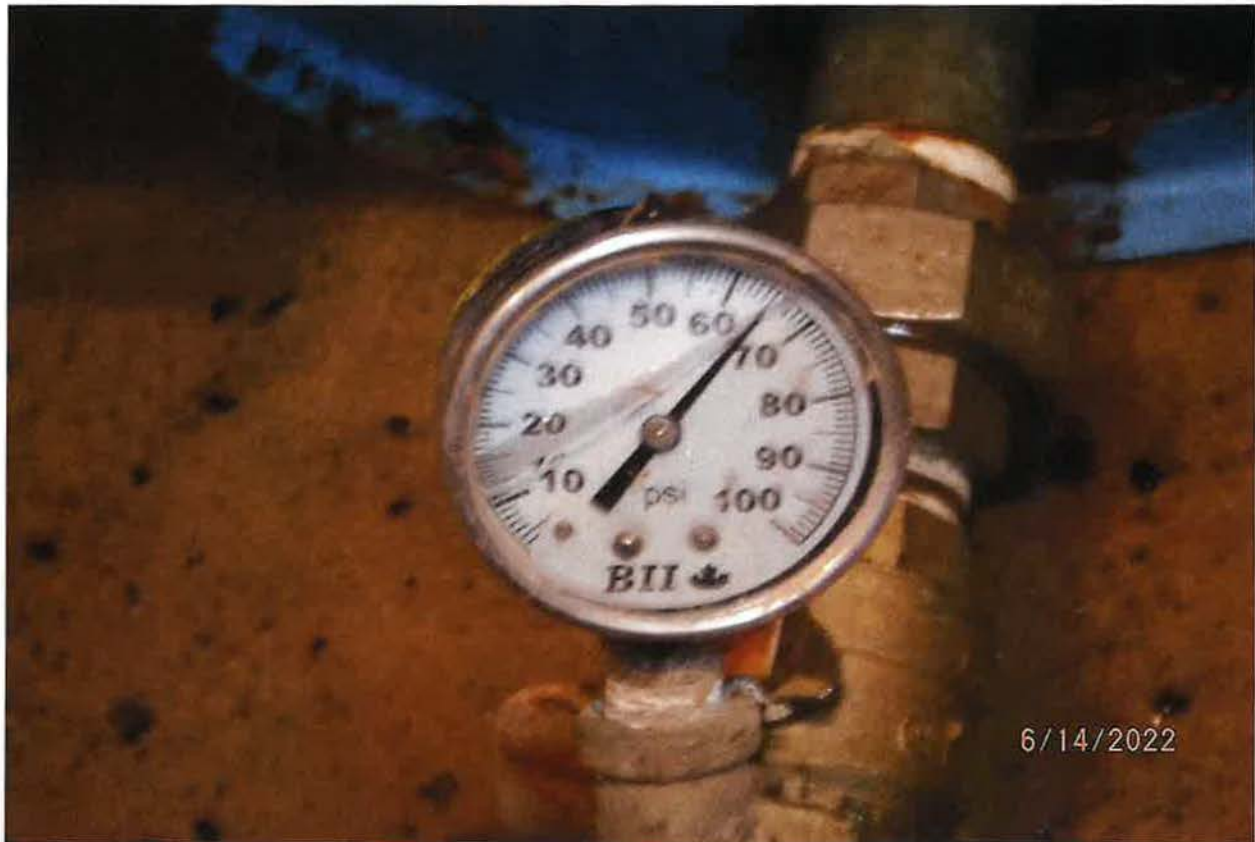
60-65 PSI OPERATING PRESSURE OBSERVED AT TIME OF EXAM
