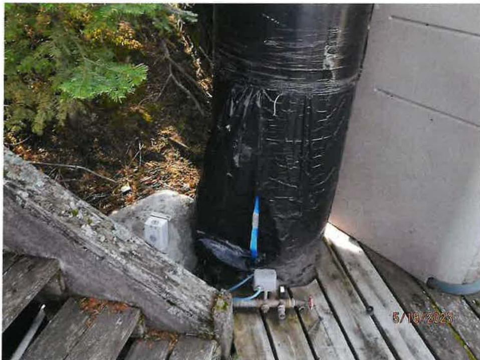
POD - IRRIGATION LINE FROM DOCK TO PRESSURE TANK (BEOW) AND PUMP
