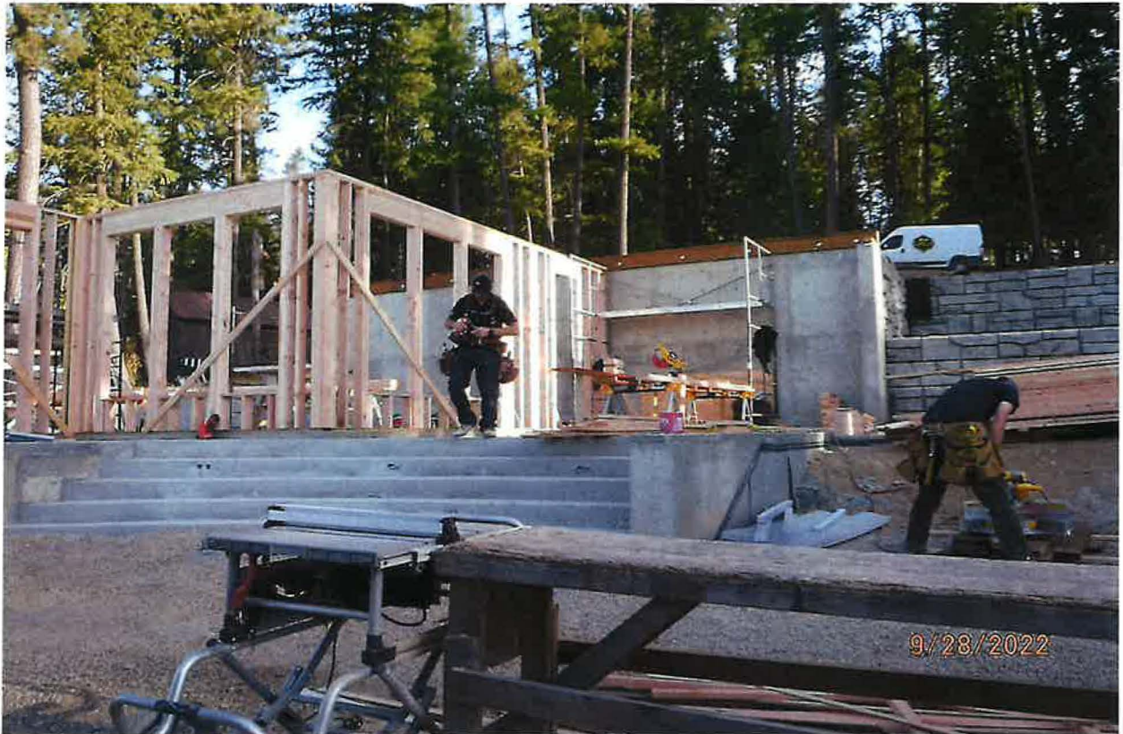
DOMESTIC POU – ORIGINAL CABIN BEING REPLACED AT TIME OF EXAM WITH NEW BUILT – DEDICATED SERVICE CONNECTION STILL IN PLACE
