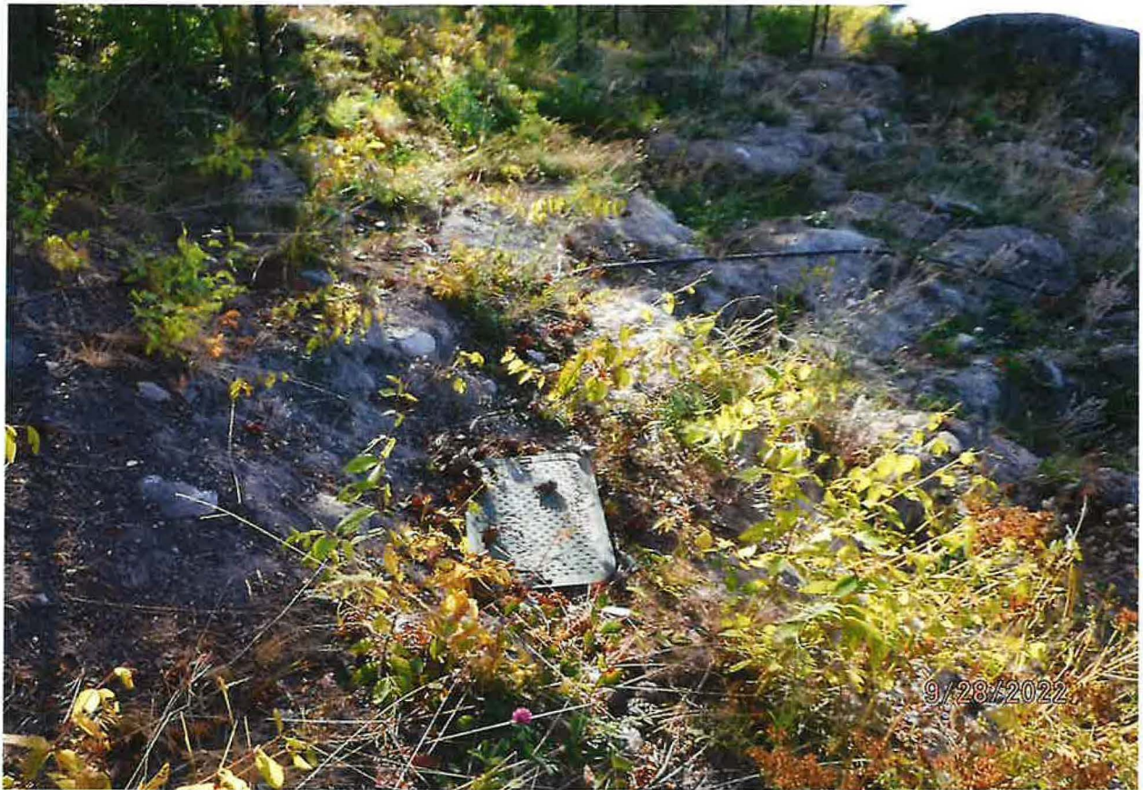
IRRIGATION POU – ZONE CONTROL BOX
