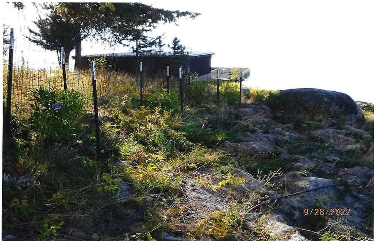
IRRIGATION POU – FENCED IN PLANTS & TREES WATERED BY SOAKER HOSE
