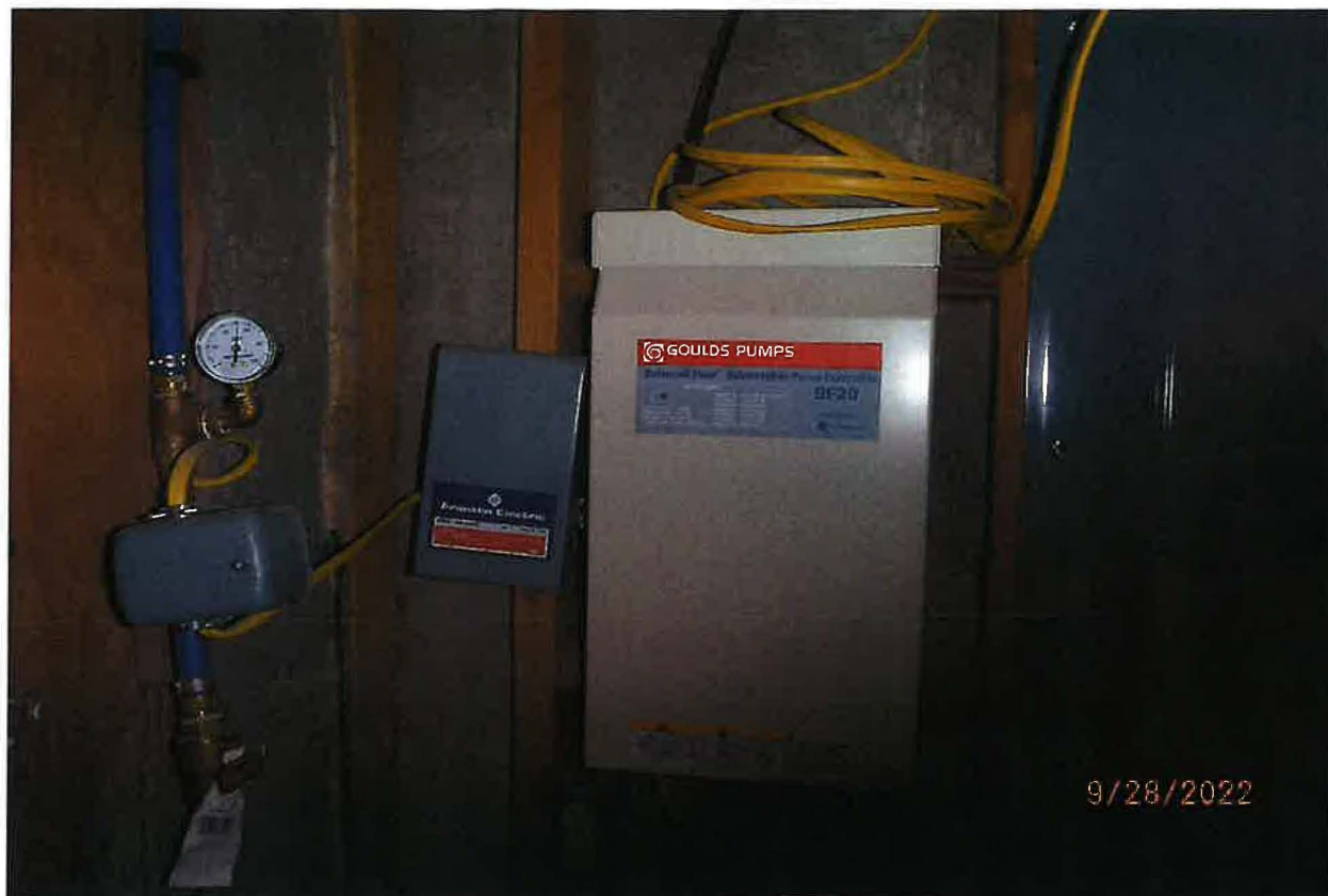
GOULDS 3 HP VARIABLE FREQ DRIVE PUMP WITH BF20 PUMP CONTROLLER
