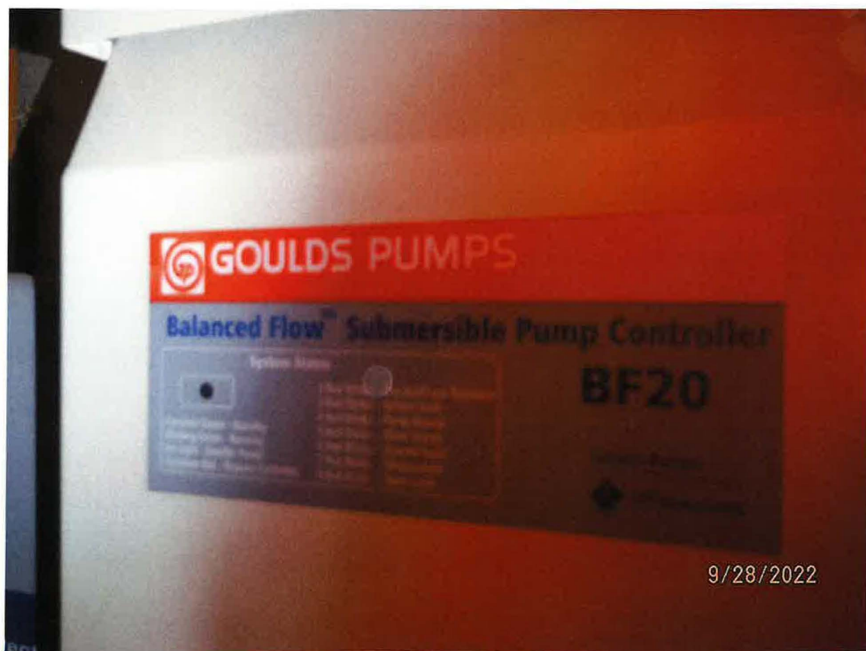
GOULDS 3 HP VARIABLE FREQ DRIVE PUMP WITH BF20 PUMP CONTROLLER
